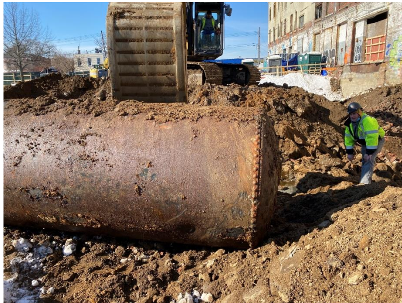
Figure 2: Tank 003 after removal.
