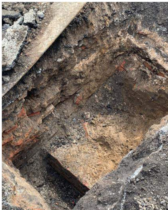
Photograph 3 – View of the interior of TP-02, including a metal plate atop a brick and concrete wall, facing east (06/01/2021)
