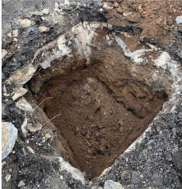
Photograph 7 – View of the interior of TP-07, including reinforce concrete, facing north (06/03/2021)
