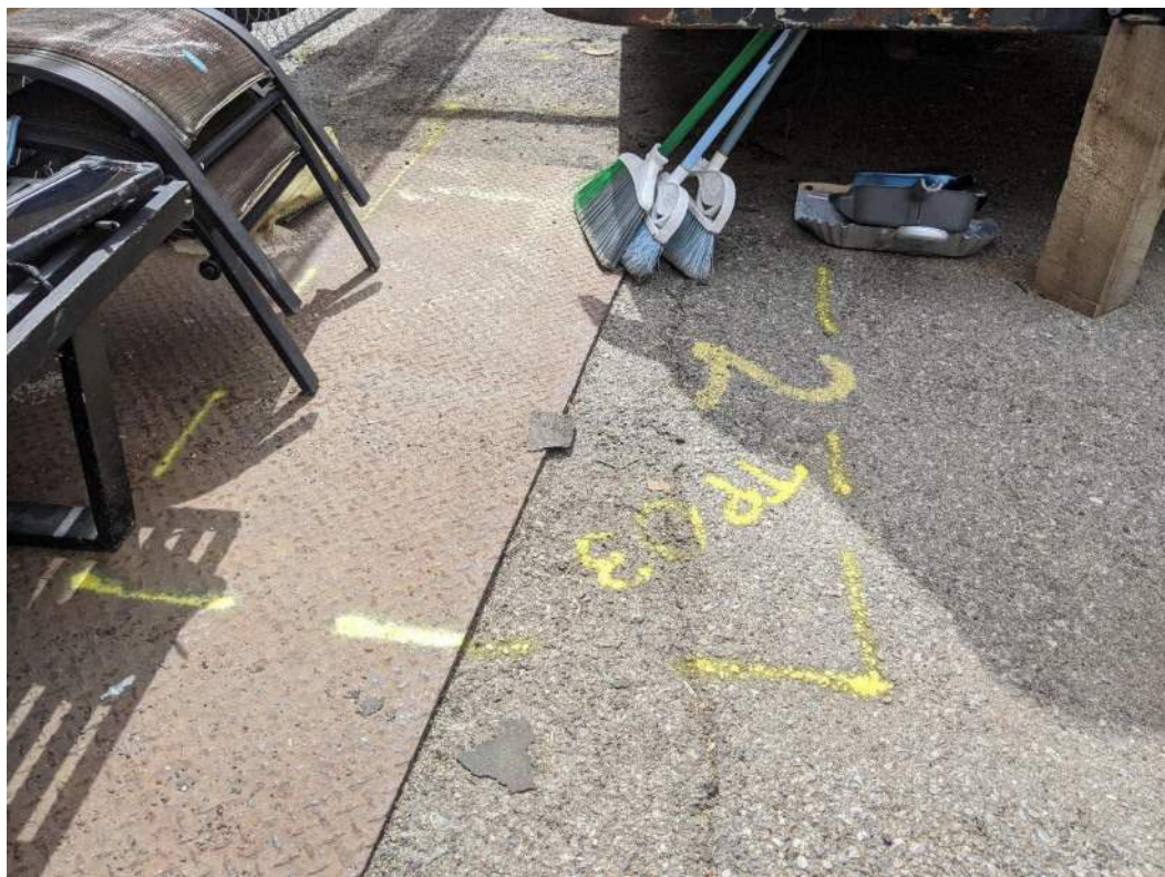
Photo 4: View of TP-03 mark out.
