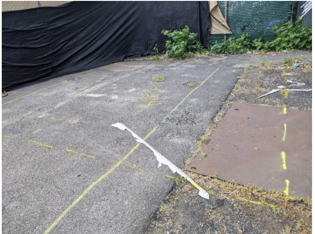
Photo 1: Example test pit mark out (TP-04) for anticipated geophysical survey.
