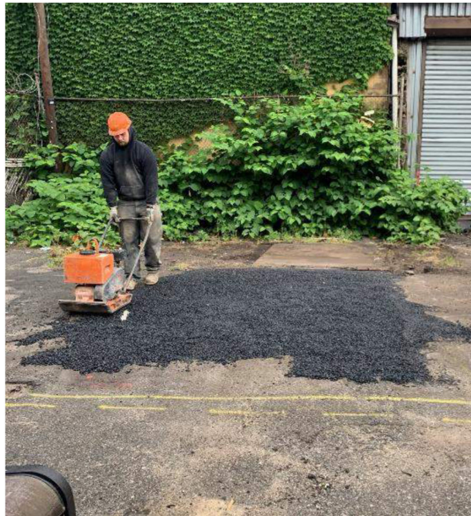
Photograph 8 – Example view of surface restoration with cold patch following test pit advancement at TP-04, facing northwest (06/03/2021)
