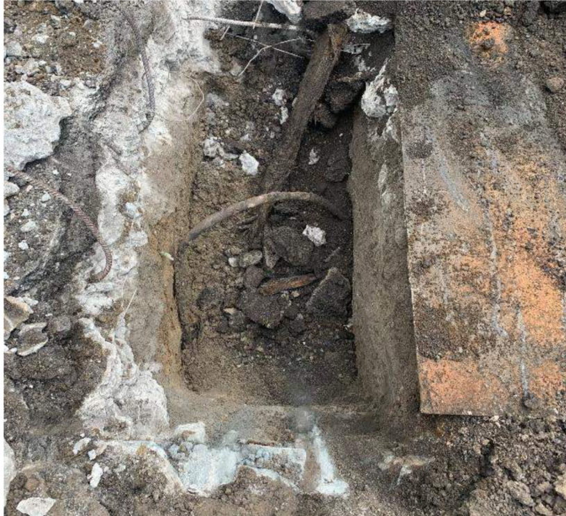
Photograph 5 – View of the interior of TP-06, including a metal plate atop reinforced concrete, facing southwest (06/02/2021)
