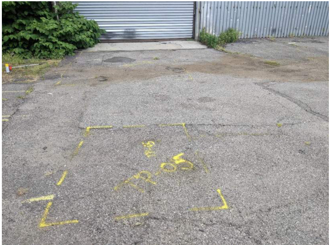
Photo 2: View of TP-05 mark out.
