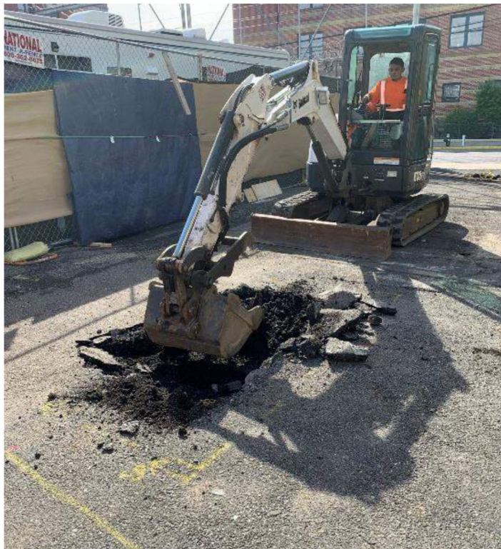
Photograph 2 – View of AARCO advancing TP-02, facing east (06/01/2021)
