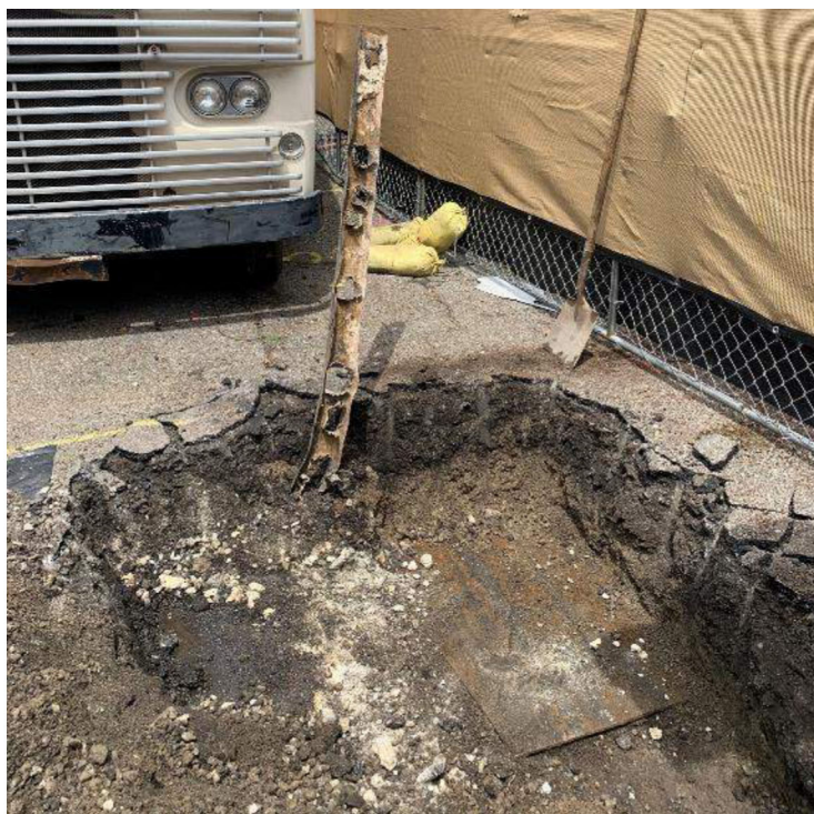
Photograph 4 – View of the interior of TP-03, including metal plates, facing northwest (06/01/2021)
