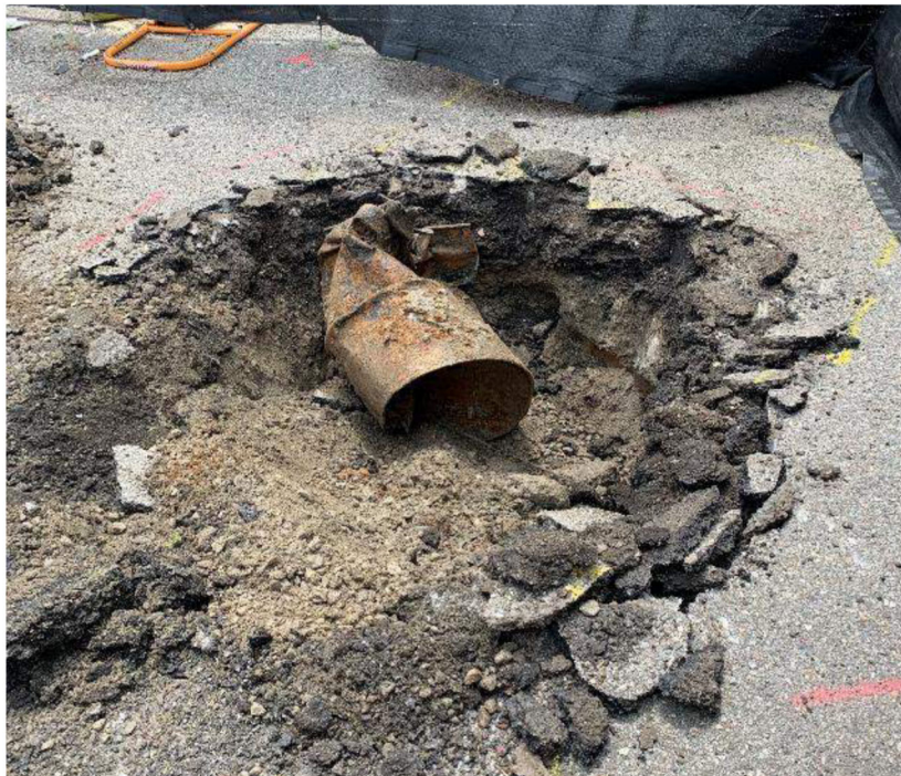
Photograph 6 – View of the interior of TP-05, including an abandoned drum, facing southwest (06/02/2021)
