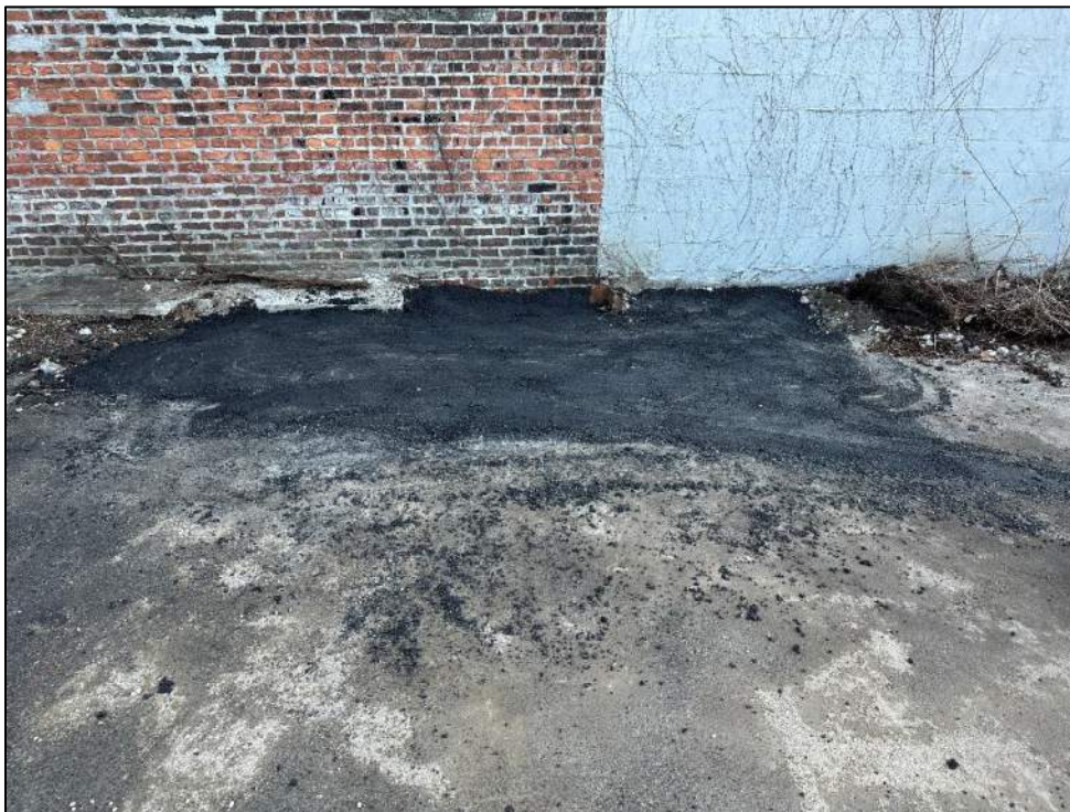
Photo 6: Backfilled and patched test pit TP-1 (facing southeast).
