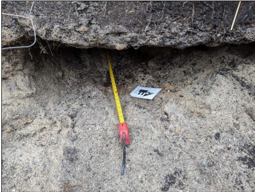
Photo 9: View of footing bottom in test pit TP-2 (facing southwest).
