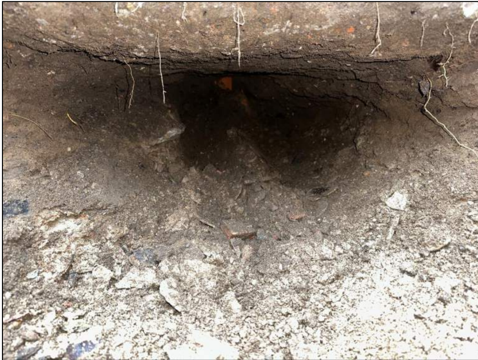
Photo 13: View of footing bottom in test pit TP-3 (facing southwest).
