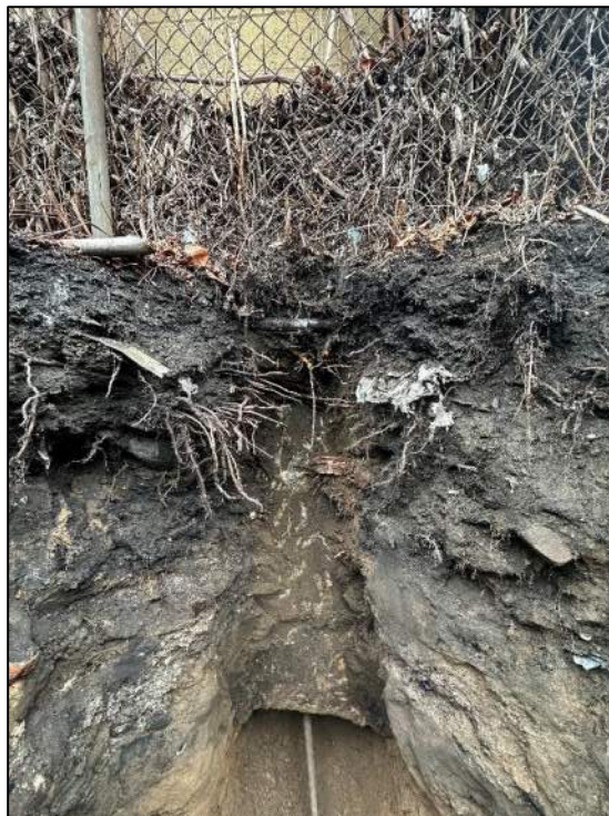
Photo 16: View of footing in test pit TP-4 (facing northwest).
