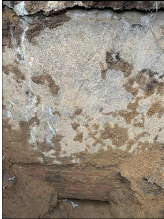
Photo 21: View of footing in test pit TP-5 (facing southwest).
