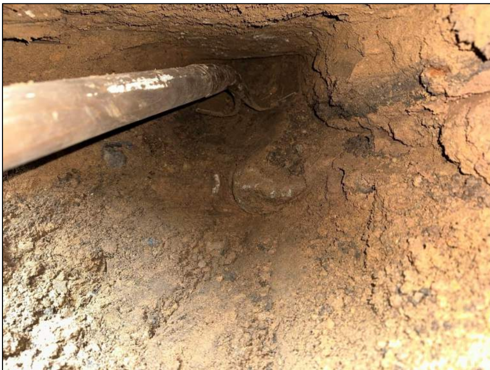
Photo 18: View of footing bottom in test pit TP-4 (facing northwest).
