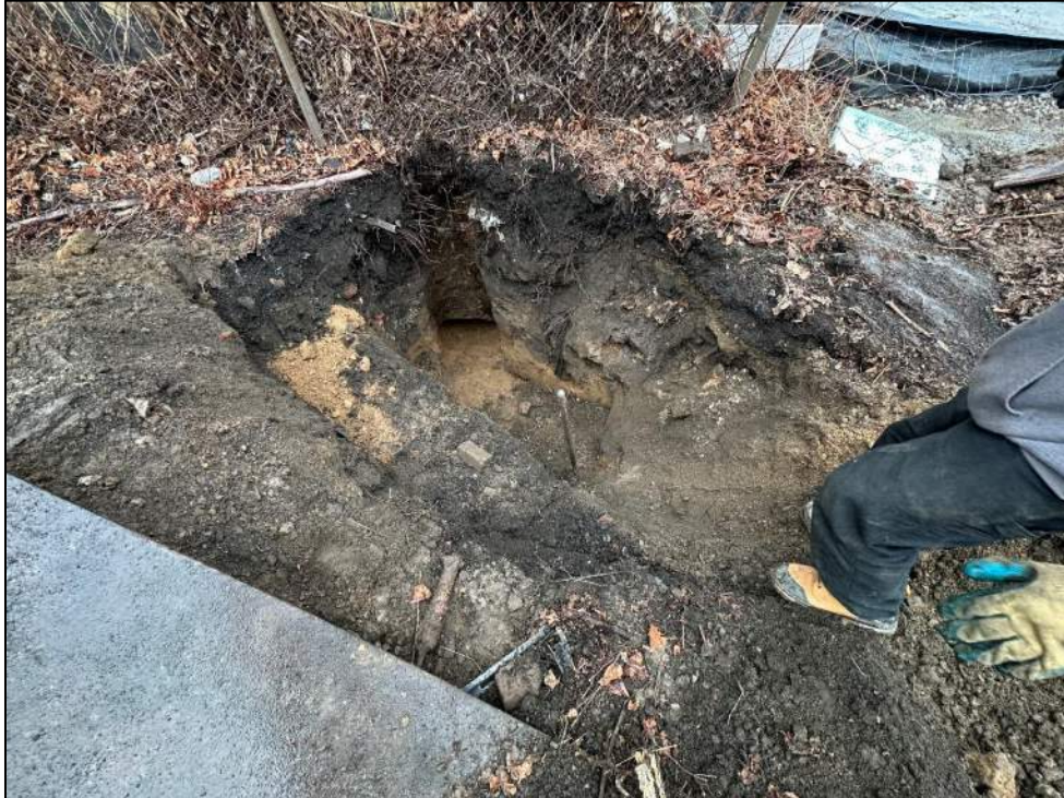
Photo 15: General view of test pit TP-4, 158 Dikeman Street (facing northwest).
