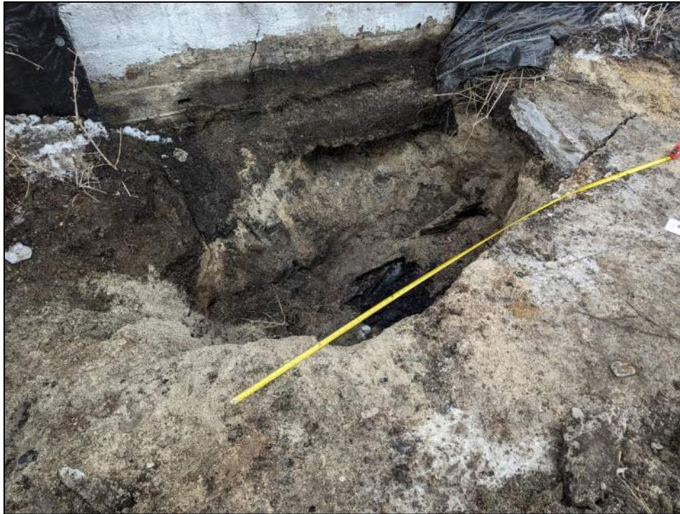
Photo 7: General view of test pit TP-2, 166 Dikeman Street (facing southwest).
