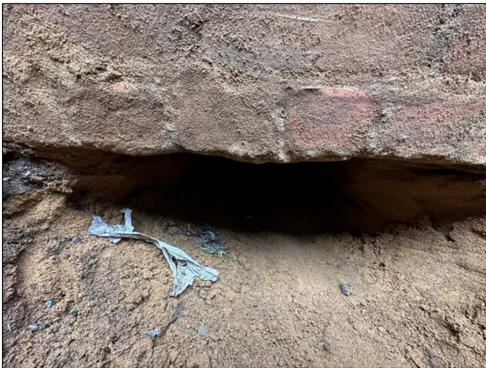
Photo 22: View of footing bottom in test pit TP-5 (facing southwest).
