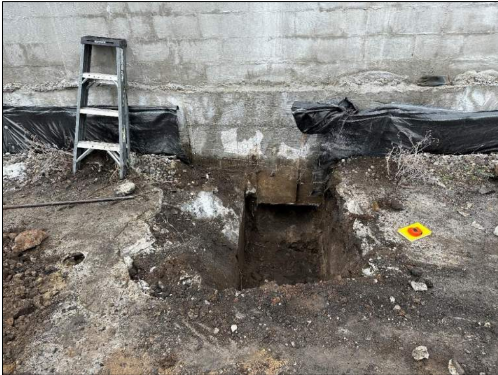
Photo 11: General view of test pit TP-3, 160 Dikeman Street (facing southwest).
