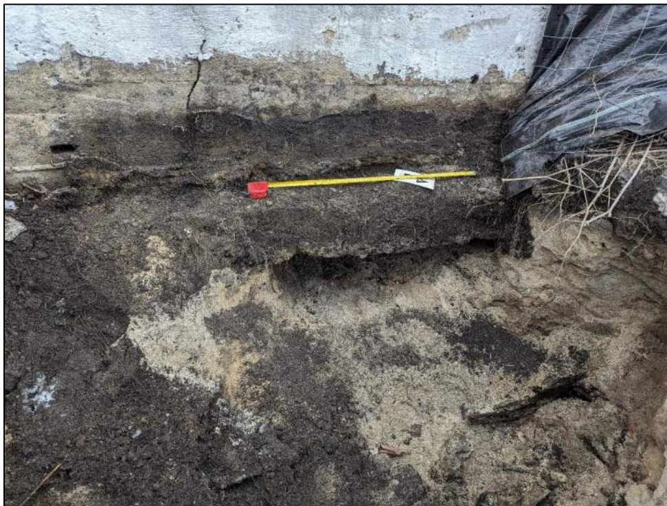
Photo 8: View of footing in test pit TP-2 (facing southwest).
