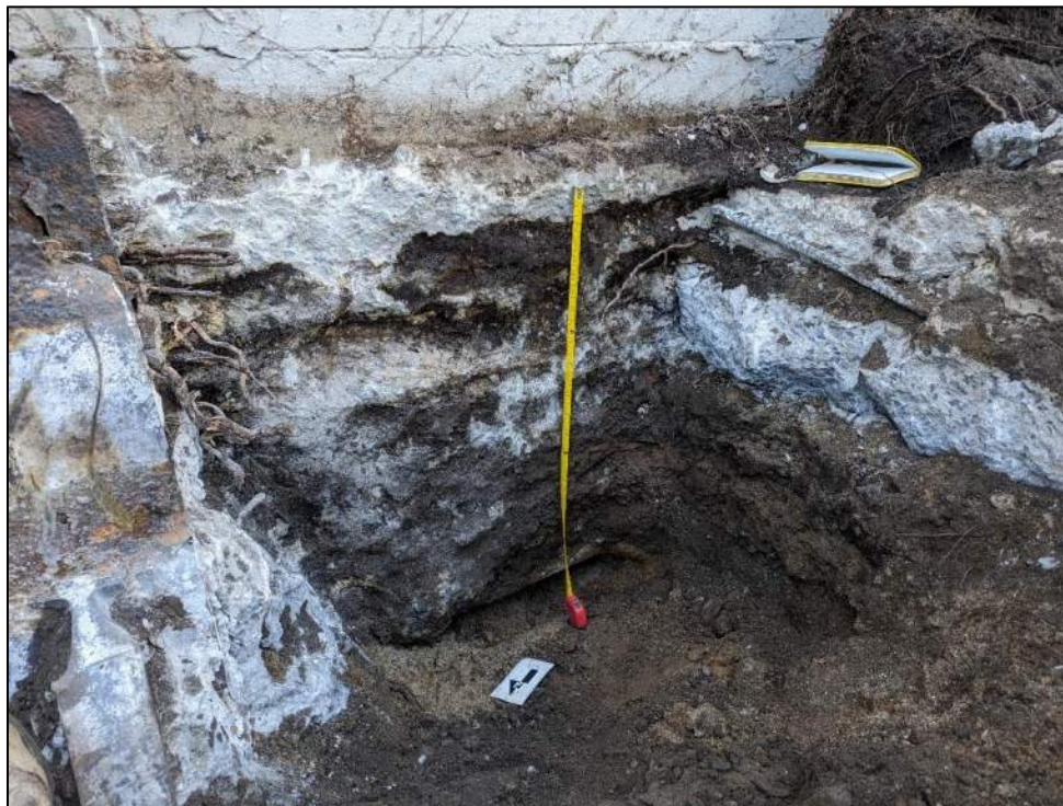
Photo 4: View of footing under 2-story portion of building in test pit TP-1 (facing south).
