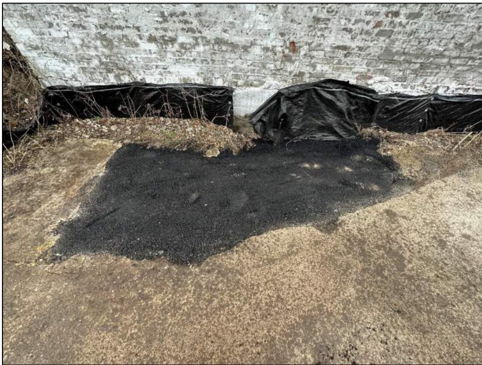
Photo 10: Backfilled and patched test pit TP-2 (facing southwest).
