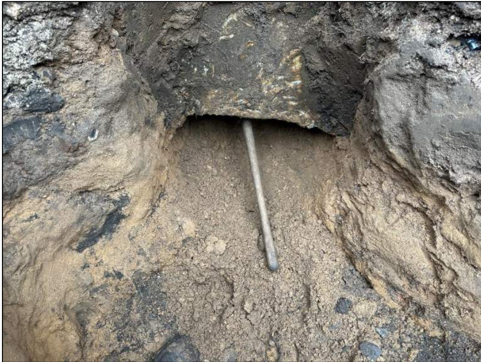
Photo 17: View of footing bottom in test pit TP-4 (facing northwest).
