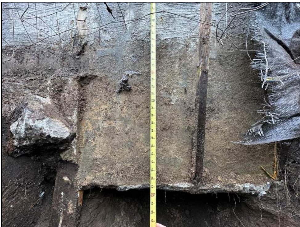
Photo 12: View of footing in test pit TP-3 (facing southwest).
