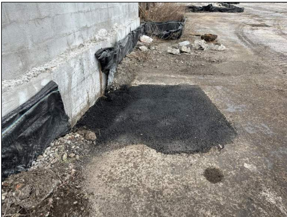
Photo 14: Backfilled and patched test pit TP-3 (facing northwest).
