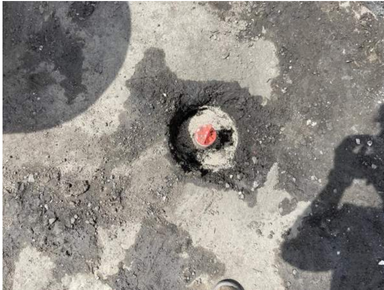
Photo 1: Groundwater monitoring well MW10 post-construction
