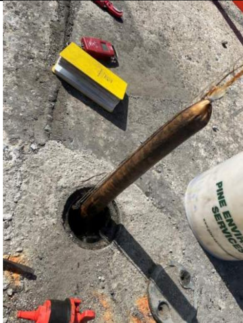
Photo 3: Absorbent sock removed from MW-012
