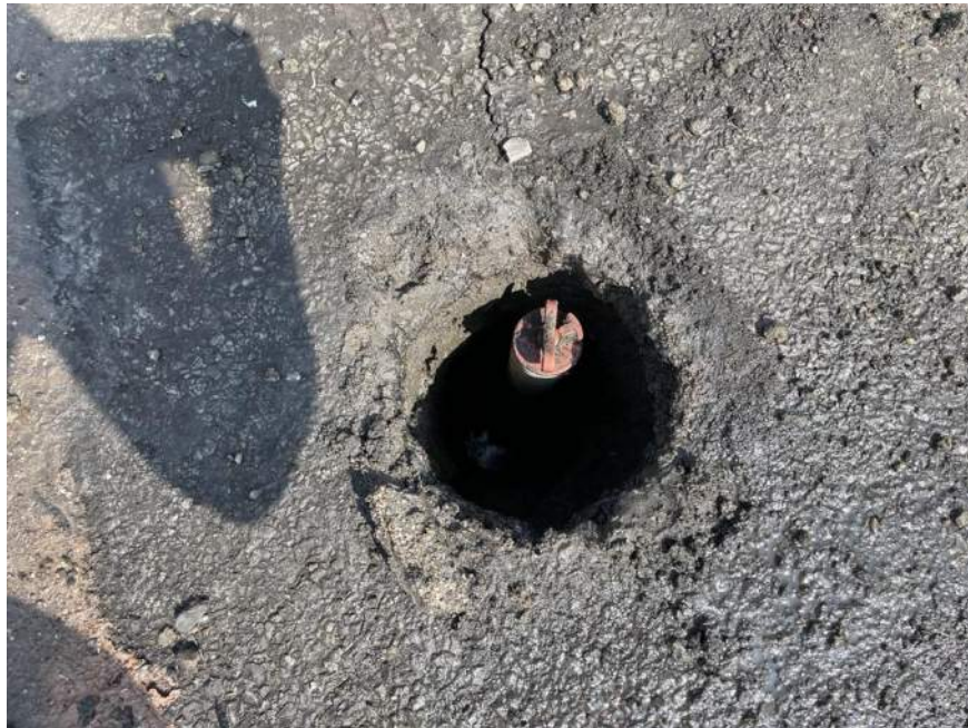
Photo 2: Monitoring well MW-01D installed in the northern part of the site.
