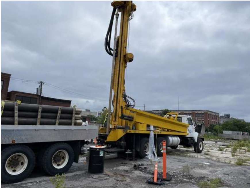
Photo 1: Coastal advancing soil boring SBD08 in the northern part of the site (facing east)
