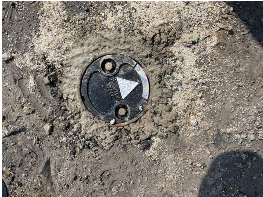
Photo 2: Installed monitoring well MW-03S in the southwestern part of the site.
