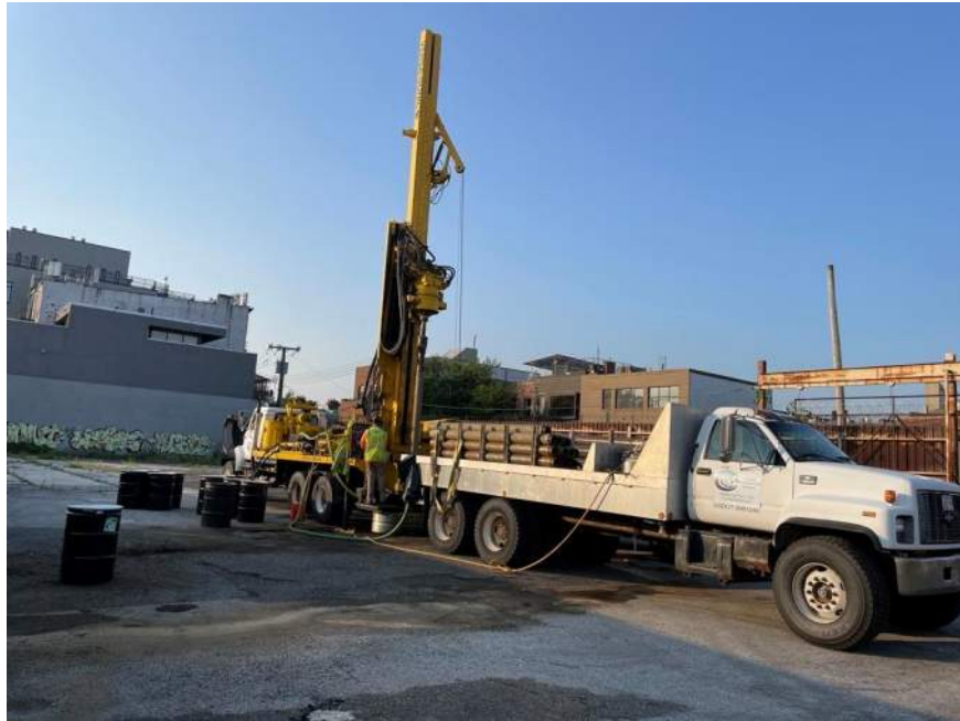
Photo 1: Coastal advancing soil boring SBD09 in the southwestern part of the site (facing south)
