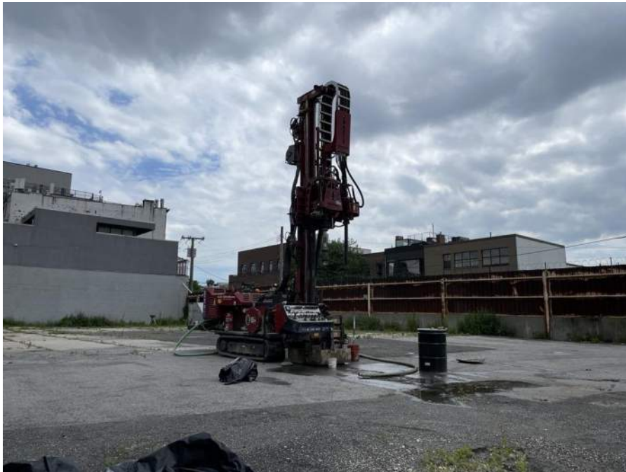
Photo 2: Coastal advancing soil boring SBD04 in the western part of the site (facing south).
