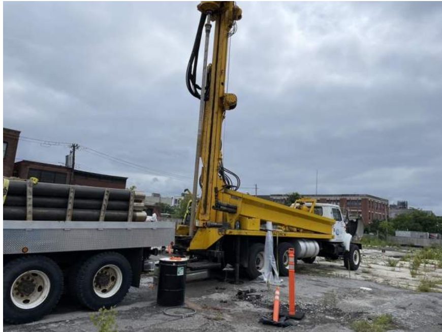
Photo 1: Coastal advancing soil boring SBD08 in the northern part of the site (facing east)
