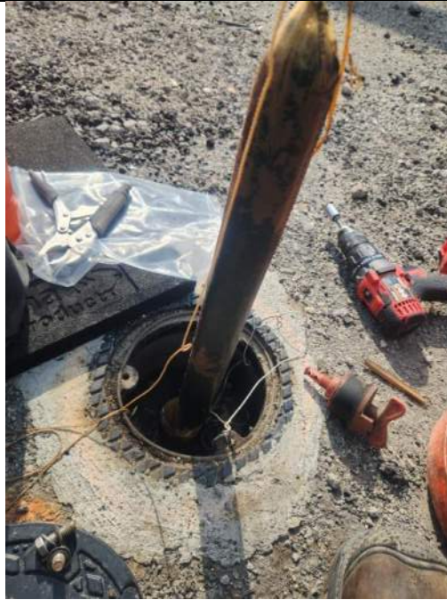
Photo 3: Absorbent sock removed from MW-002
