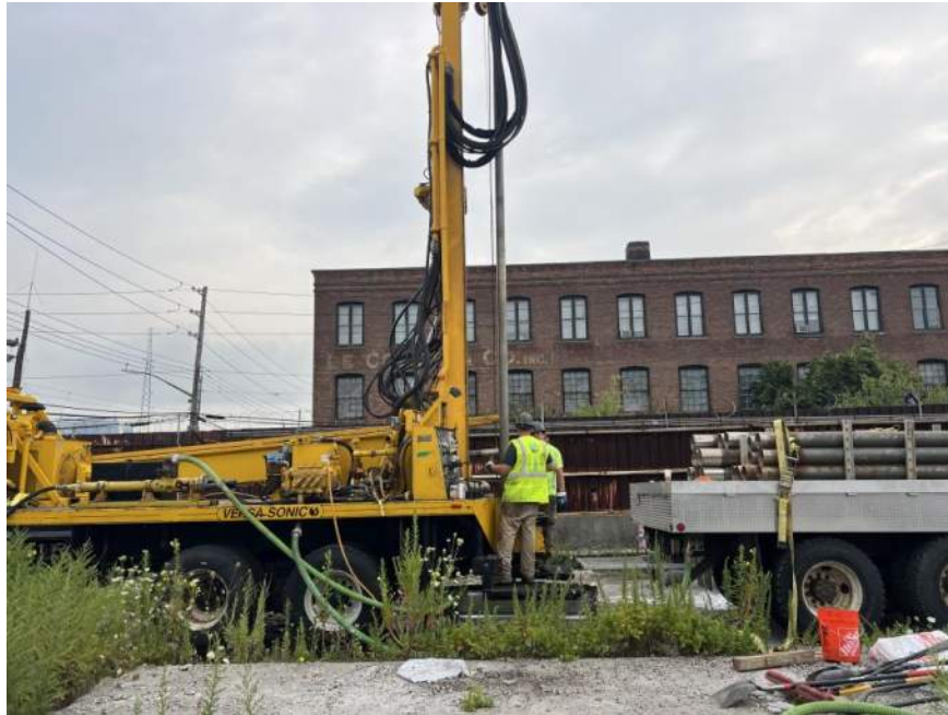
Photo 1: Coastal advancing soil boring SBD07 in the northern part of the site (facing north)
