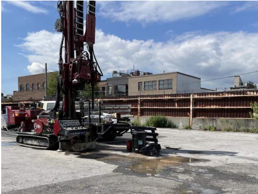
Photo 1: Coastal advancing soil boring SBD04 in the western part of the site (facing southwest)
