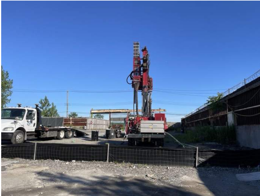
Photo 1: Coastal advancing soil boring SB03 in the northeastern part of the site (facing northwest)
