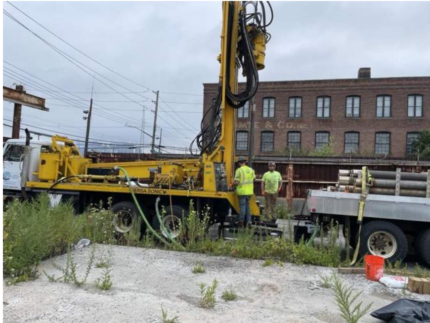
Photo 1: Coastal advancing soil boring SBD07 in the northern part of the site (facing northeast)
