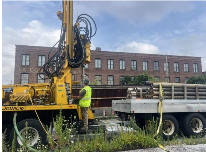
Photo 1: Coastal advancing soil boring SBD07 in the northern part of the site (facing north)
