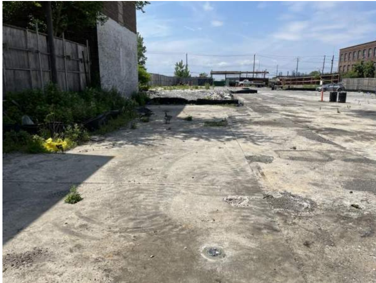
Photo 1: Groundwater monitoring well MW08 post-construction
