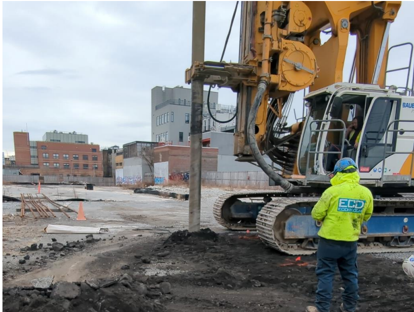
Photo 1: ECD drilling displacement pile R-3C in the northern part of the site (facing southeast).
