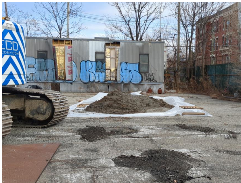
Photo 2: Stockpiled drilling spoils from CFA piles R-5B and R-5D in the eastern part of the site (facing northeast).
