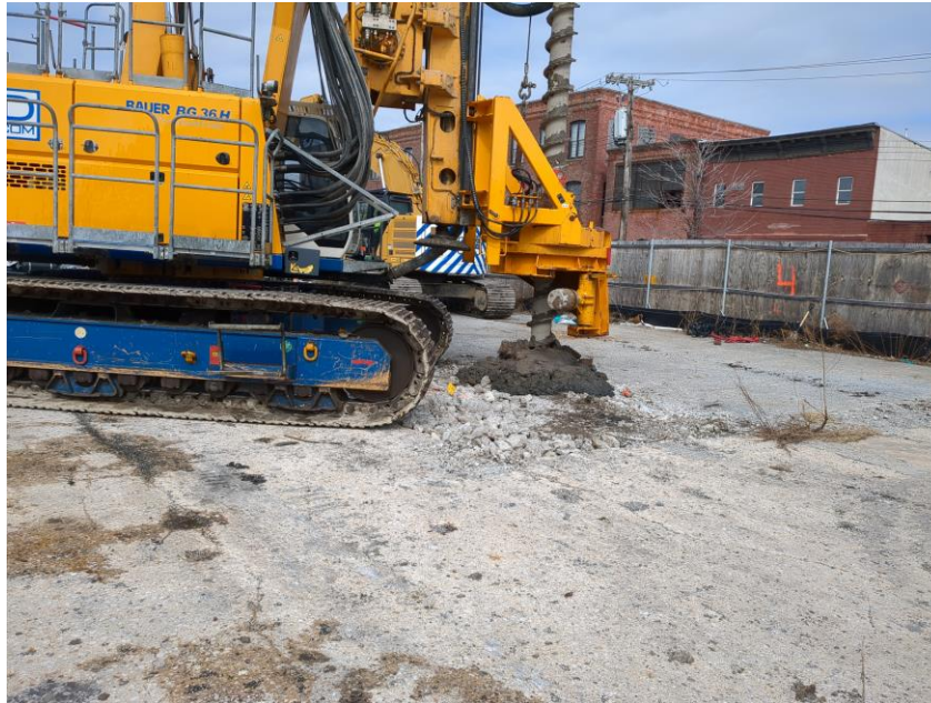
Photo 1: ECD advancing CFA pile R-4C in the central part of the site (facing north).
