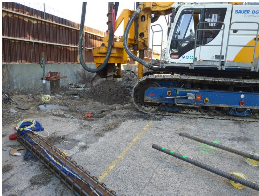
Photo 1: ECD advancing CFA pile C-2 in the southern part of the site (facing west)
