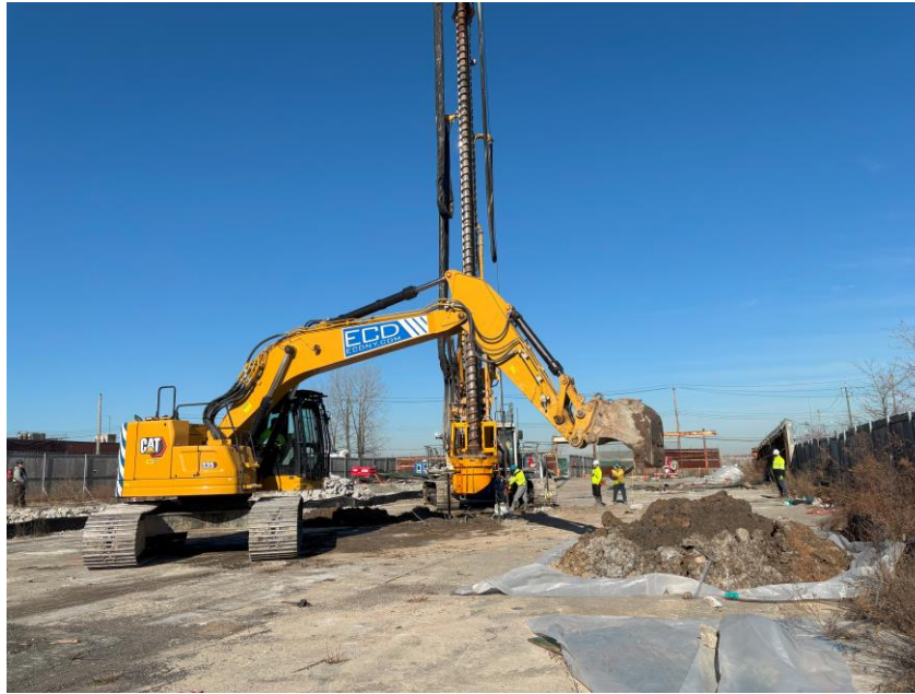
Photo 1: Stockpiled drilling spoils from CFA piles R-15 and R-16 staged in the eastern part of the site (facing northwest)
