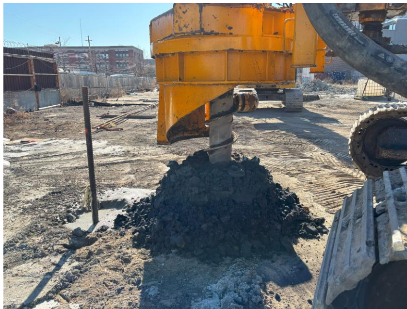
Photo 2: ECD advancing CFA pile R-12 in the northern part of the site (facing east)
