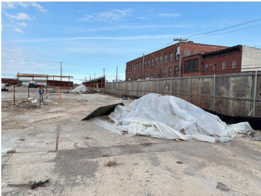
Photo 2: Stockpiled drilling spoils from CFA piles R-13, R-14, R-15, R-16 and CT-4 staged in the eastern part of the site (facing north)
