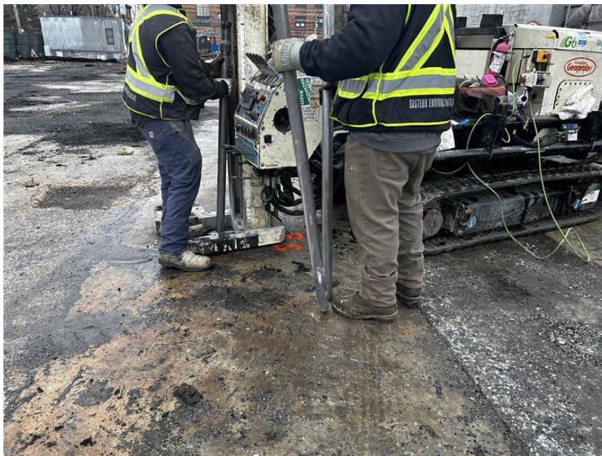
Photo 1: Eastern advancing soil boring WC08B in the central part of the site (facing southwest)
