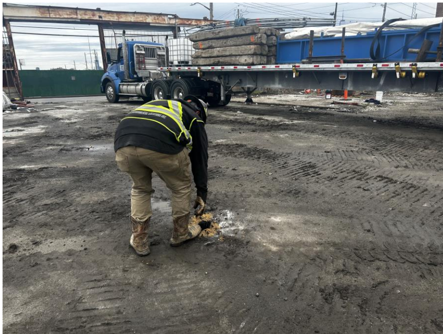
Photo 2: Eastern restoring boring location WC06E with clean sand to surface grade (facing north)
