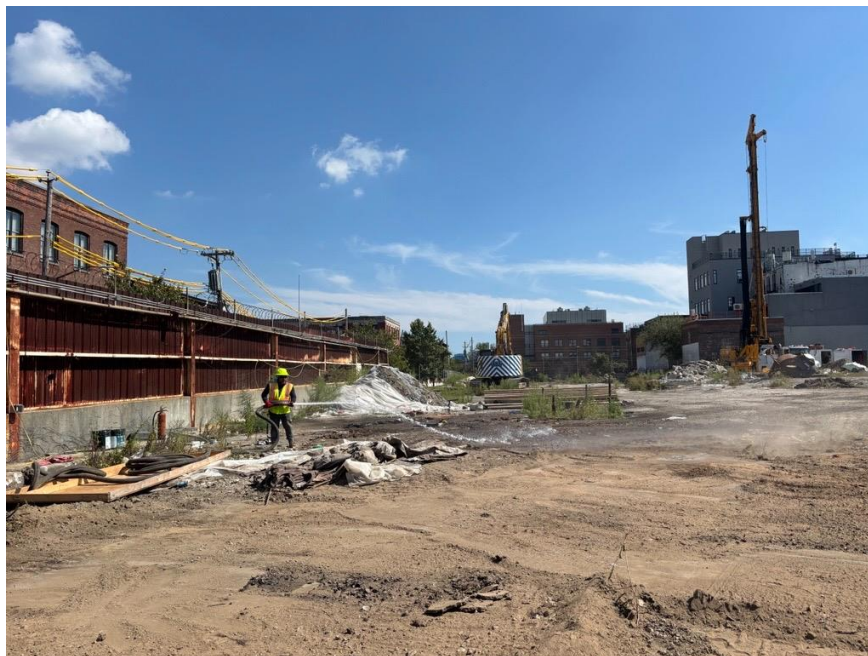
Photo 2: ECD spraying water for dust suppression during concrete removal (facing east).
