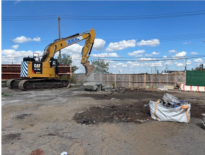
Photo 1: ECD removing concrete and asphalt in the western part of the site (facing northwest)
