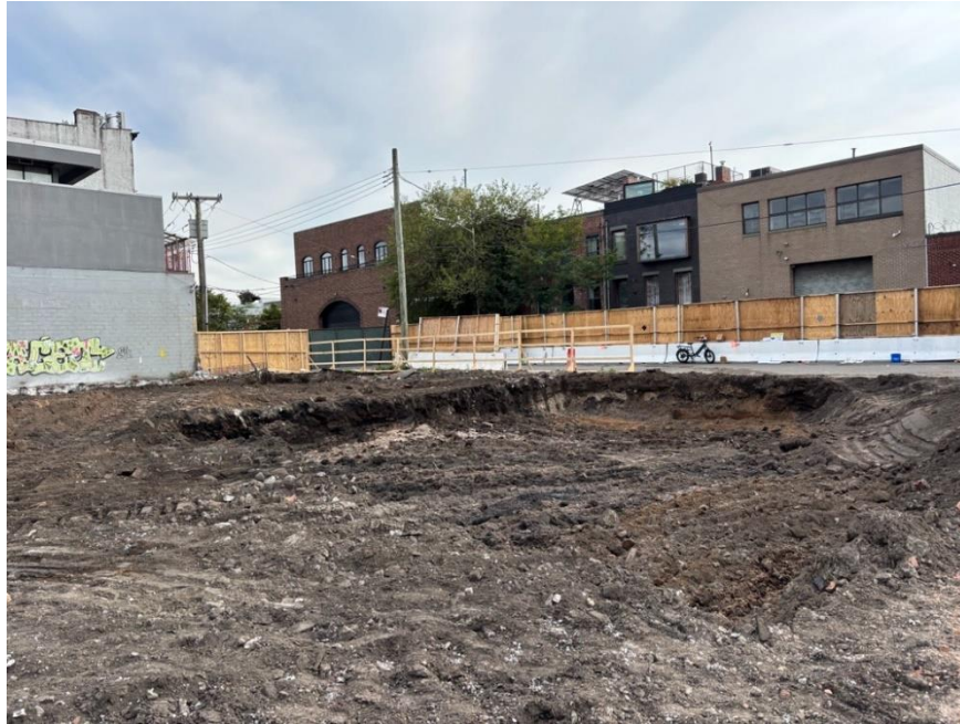
Photo 1: Excavated area to about 3 feet bgs in the western part of the site (facing southwest)
