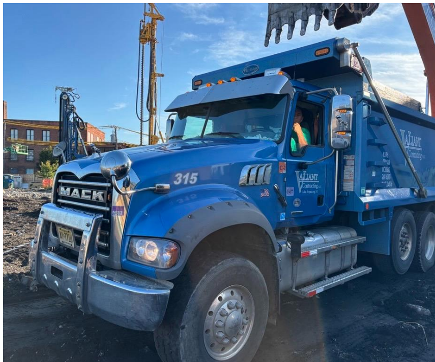
Photo 2: ECD live-loading non-hazardous non-native fill for off-site disposal (facing east).
