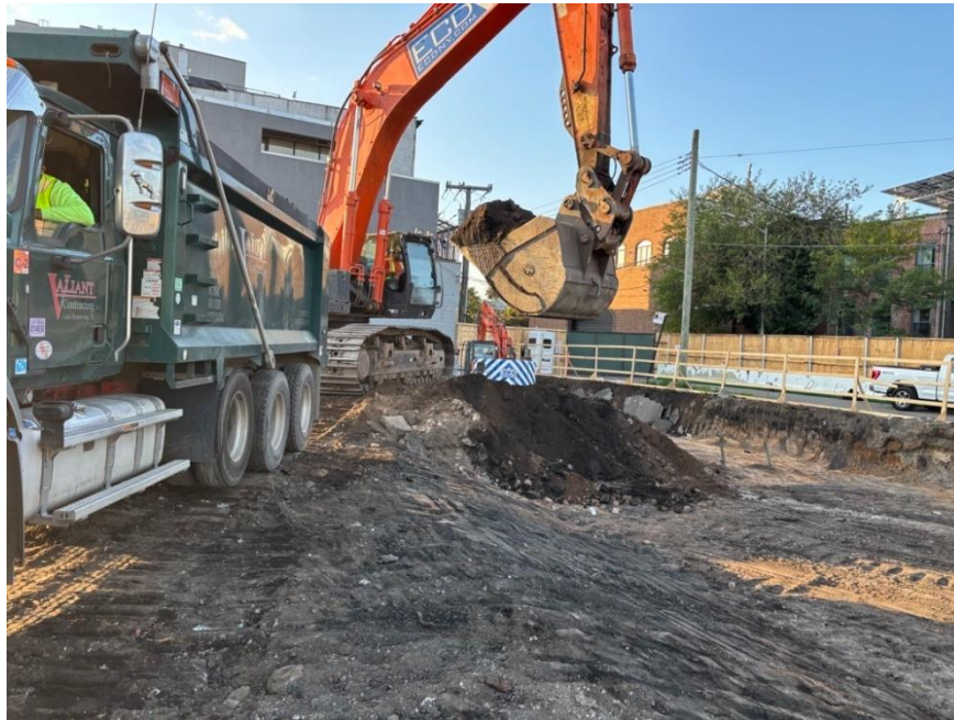
Photo 1: ECD loading non-hazardous non-native fill in the central part of the site for off-site disposal (facing north)
