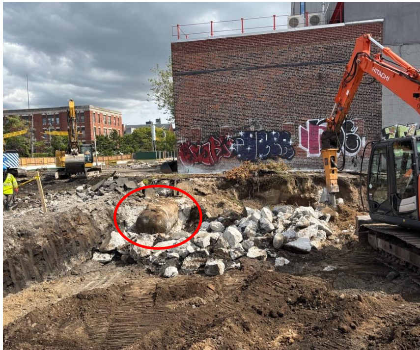
Photo 2: Uncovered UST and demolished concrete and asphalt in the western part of the site (facing south).
