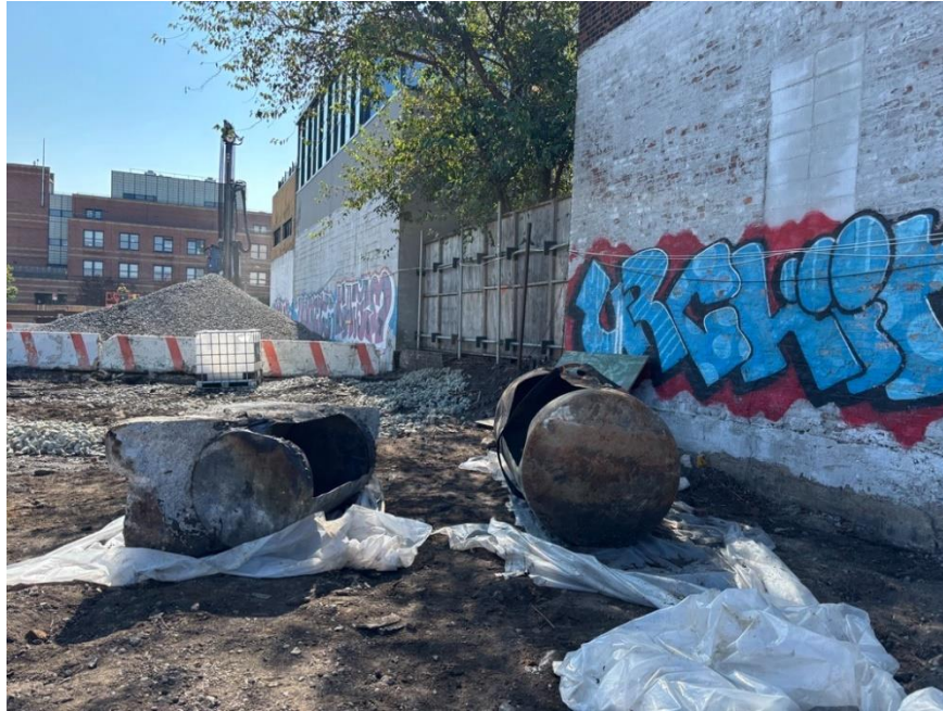
Photo 1: View of the emptied UST and suspected boiler staged on polyethylene sheeting in the central part of the site (facing southeast)
