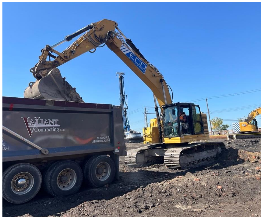
Photo 2: ECD loading non-hazardous non-native fill in the northern part of the site for off-site disposal (facing north).
