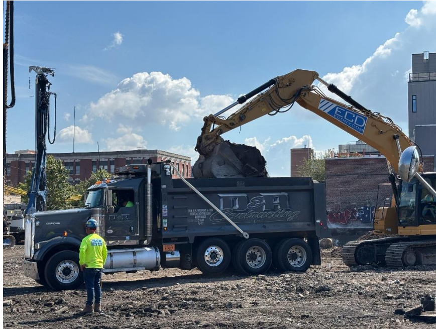
Photo 1: ECD loading non-hazardous non-native fill in the western part of the site for off-site disposal (facing east)
