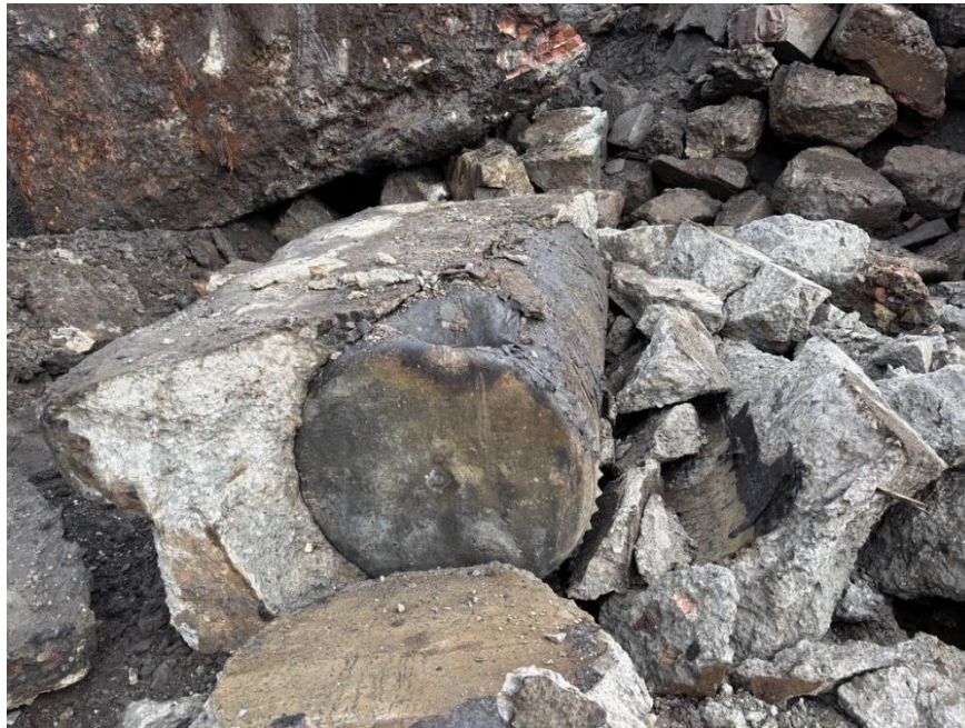
Photo 1: View of suspected boiler encased in concrete in the western part of the site (facing west)
