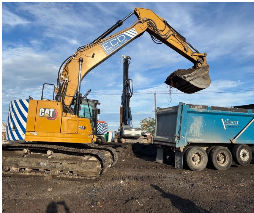
Photo 2: ECD loading non-hazardous non-native fill in the western part of the site for off-site disposal (facing north).
