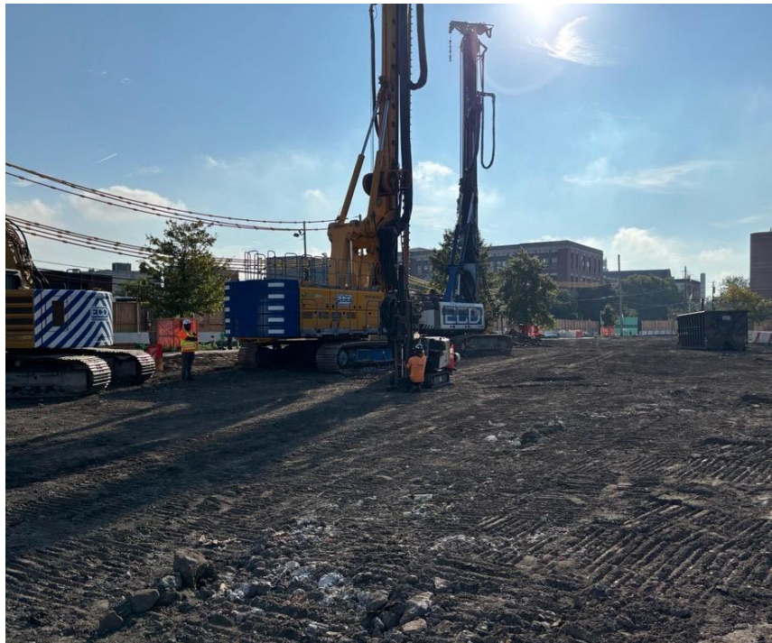
Photo 2: Lakewood advancing soil borings for supplemental sulfate sampling in the central part of the site (facing east).
