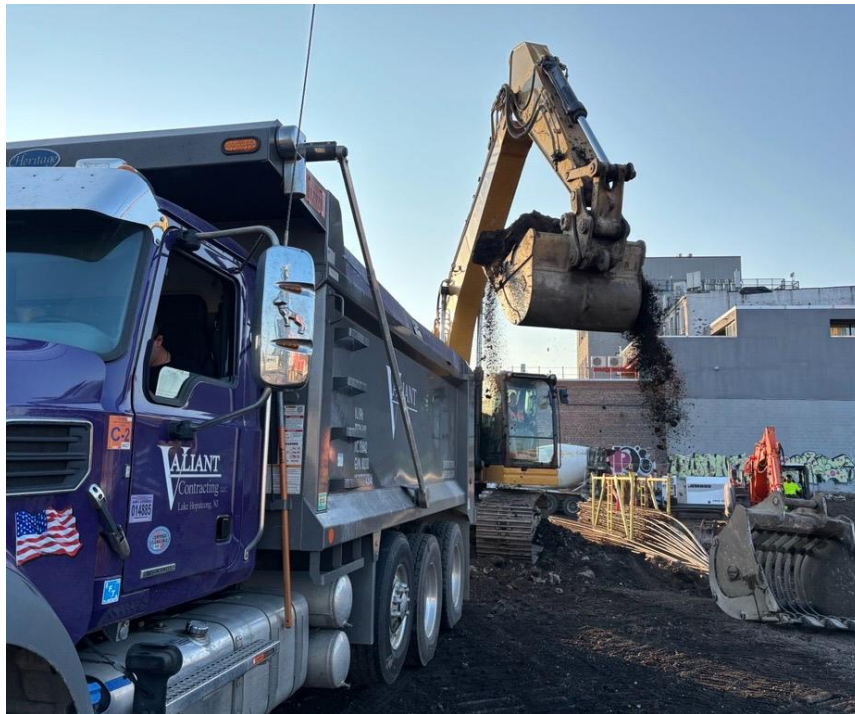
Photo 2: ECD loading non-hazardous non-native fill in the western part of the site for off-site disposal (facing south).
