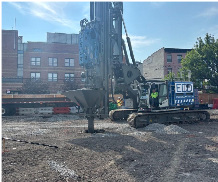
Photo 2: ECD advancing stone column ground improvement elements in the southern part of the site (facing south).
