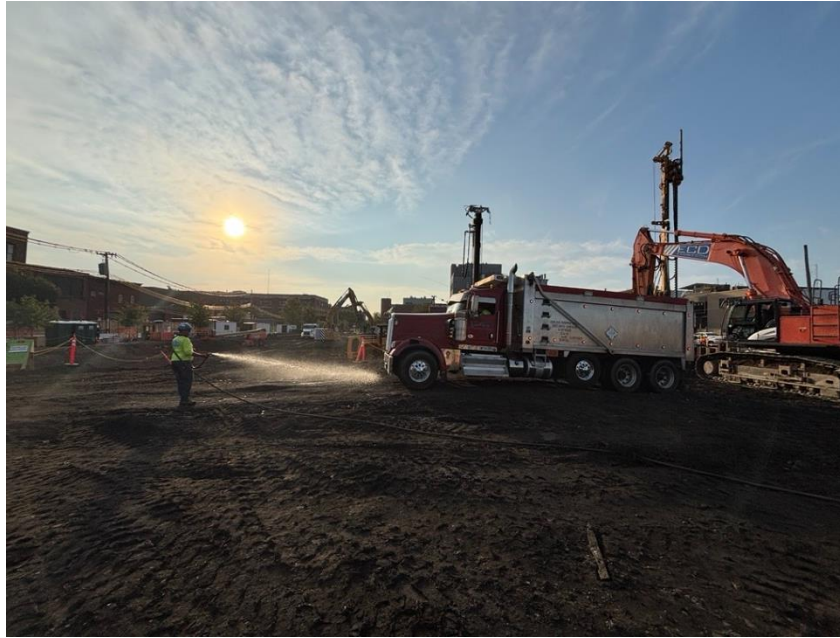
Photo 3: ECD spraying water for dust suppression during off-site disposal within the northern part of the site (facing southeast).
