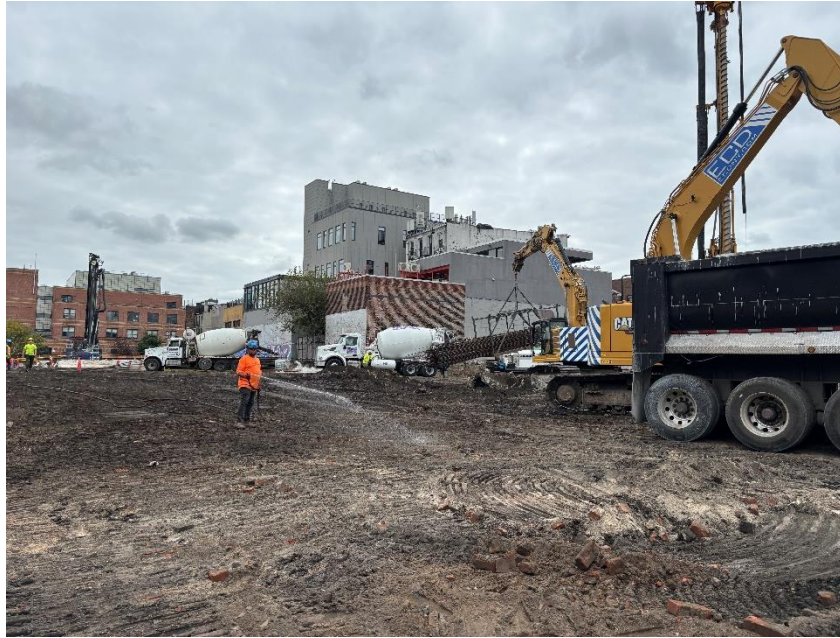
Photo 3: ECD spraying water for dust suppression within the northern part of the site (facing southeast).
