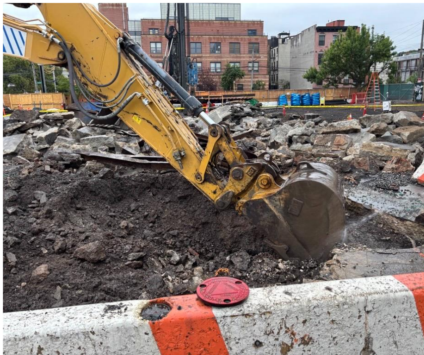
Photo 2: ECD excavating hazardous non-native fill in the southern part of the site (facing south).
