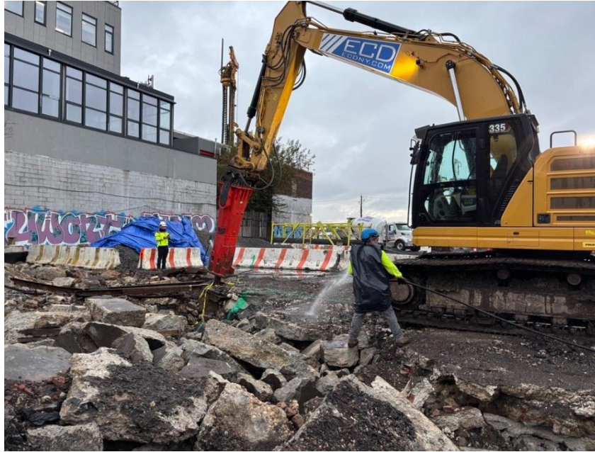
Photo 3: ECD spraying water for dust suppression during concrete removal within the southern part of the site (facing northwest).
