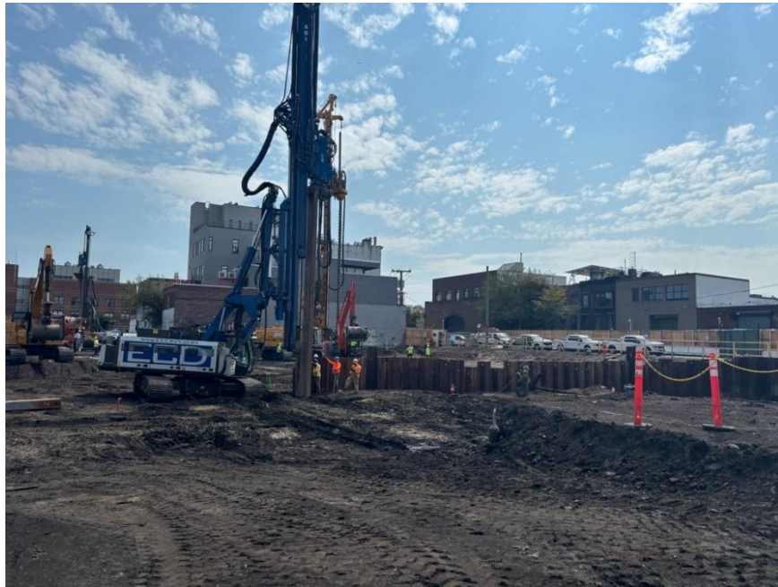
Photo 1: View of ECD installing sheet piles in the western part of the site (facing southwest)
