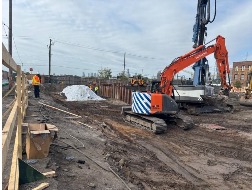
Photo 1: View of the drilling spoils staged on and covered with polyethylene sheeting in the western part of the site (facing north)
