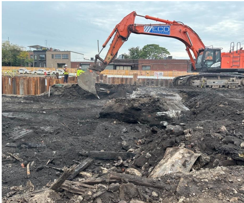
Photo 2: ECD removing concrete and asphalt in the northwestern part of the site (facing west).
