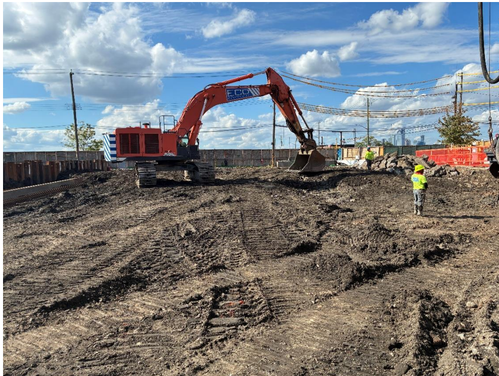
Photo 2: ECD grading the northwestern part of the site (facing west).
