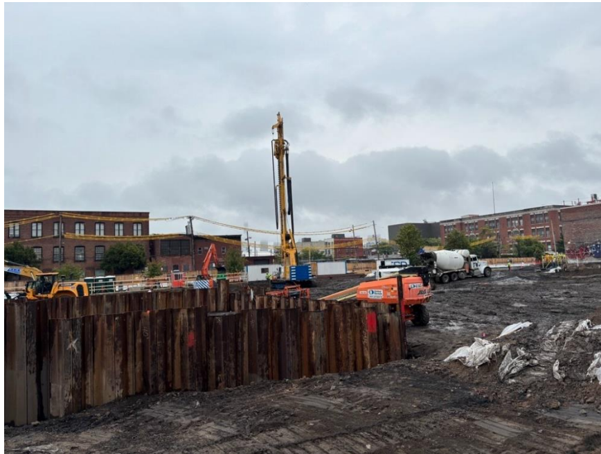
Photo 1: View of ECD installing CFA piles in the eastern part of the site (facing east)
