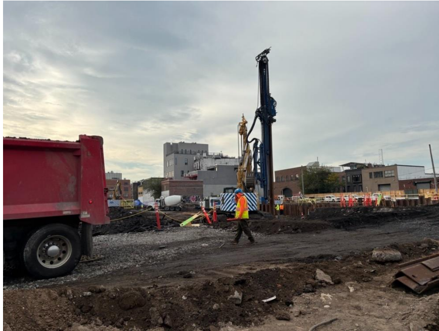
Photo 1: ECD installing sheet piles in the western part of the site (facing southwest)
