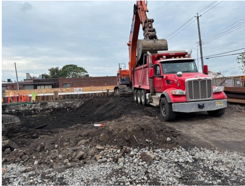
Photo 3: ECD loading non-hazardous non-native fill in the northwestern part of the site for off-site disposal (facing west).
