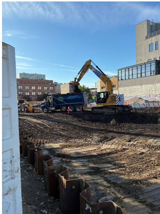
Photo 2: ECD live loading non-hazardous non-native fill in the southern part of the site (facing southeast).
