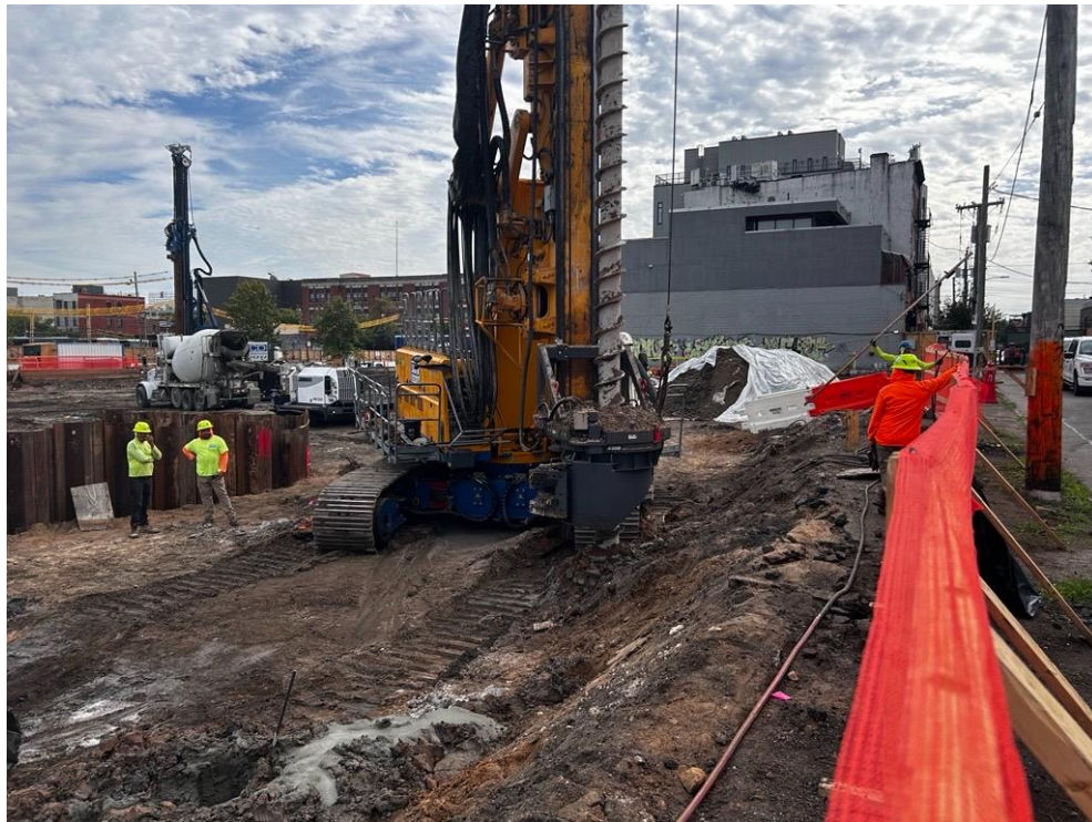
Photo 2: ECD advancing continuous flight auger in the southwestern part of the site (facing southeast).
