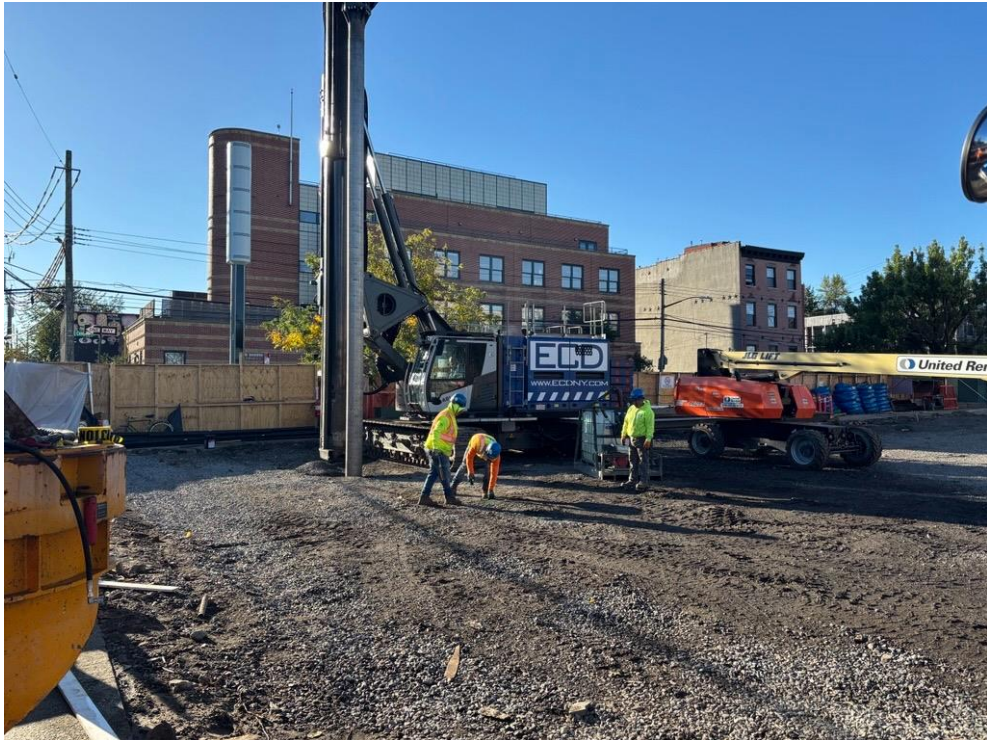
Photo 2: ECD advancing stone columns for geotechnical ground improvement in the southern part of the site (facing south).
