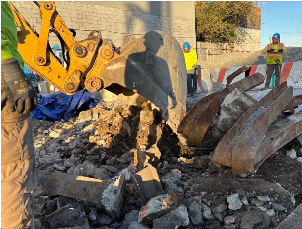
Photo 1: View of ECD removing asphalt and concrete in the eastern part of the site (facing northwest)
