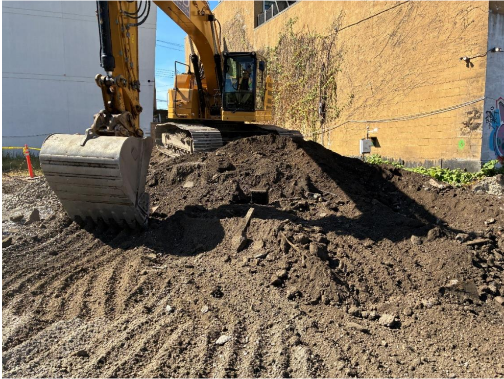
Photo 1: ECD excavating and stockpiling non-native fill in the southern part of the site (facing northwest)
