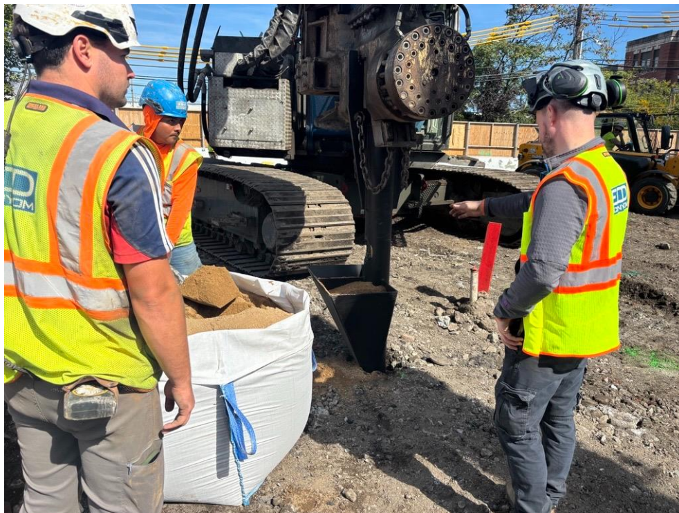
Photo 2: ECD advancing Petrofix pilot test injection points in the eastern part of the site (facing southeast).
