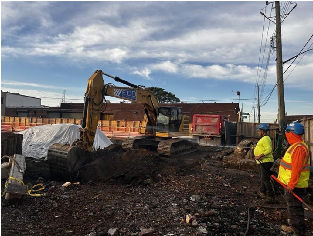
Photo 1: View of ECD live-loading non-hazardous non-native material in the western part of the site (facing west)
