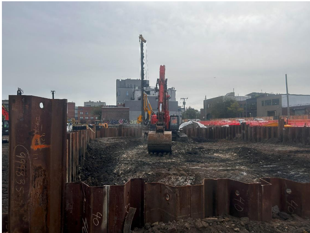
Photo 2: ECD grading in the western part of the site (facing south).
