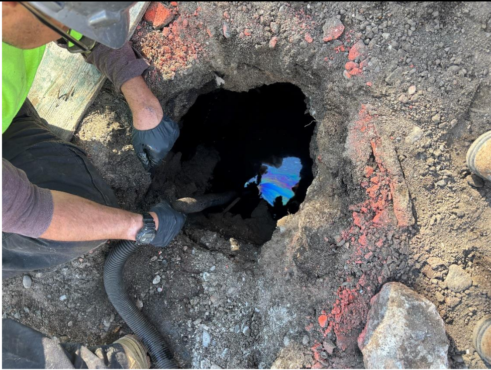
Photo 3: IRT removing water with a sheen from the approximately 200-gallon UST in the southern part of the site.
