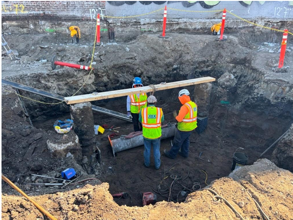
Photo 2: ECD preparing for lateral load test in the western part of the site (facing south).
