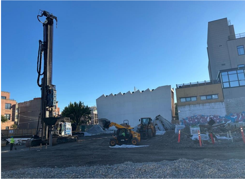
Photo 1: ECD installing stone columns in the eastern part of site (facing south)
