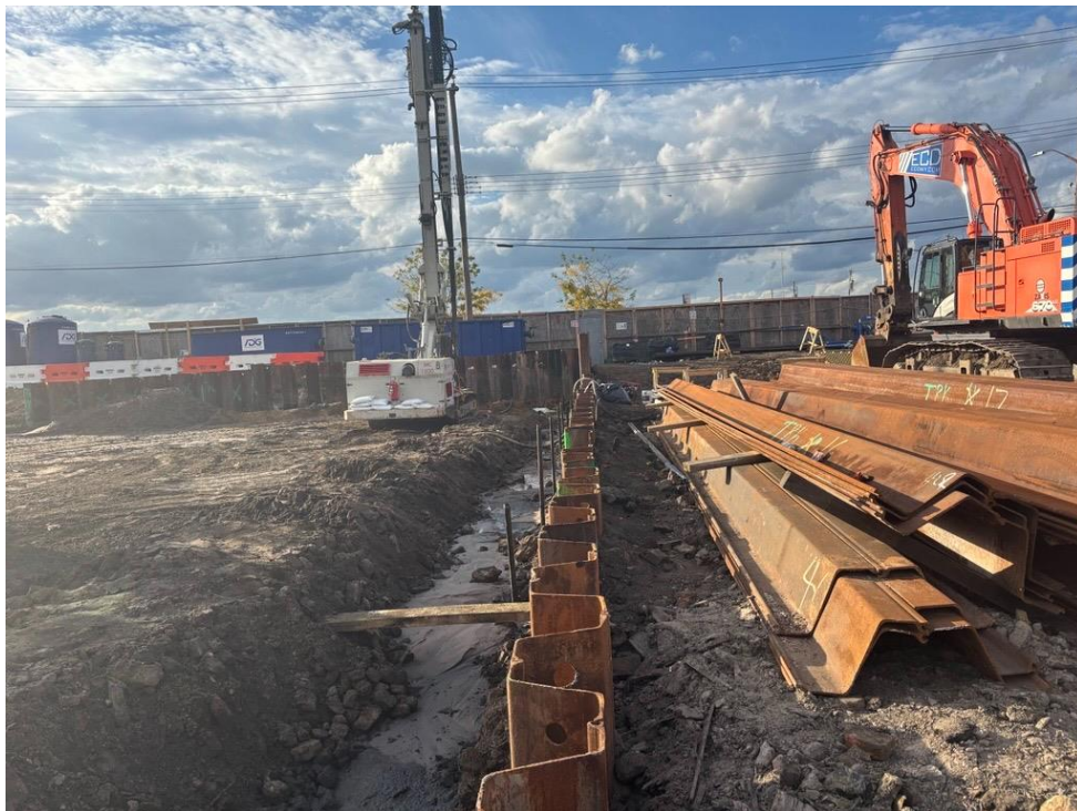
Photo 2: ECD installing dewatering wells in the northern part of the site (facing north).
