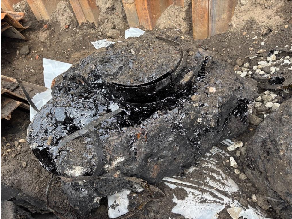
Photo 3: Concrete-encased wooden cask stockpiled on poly in the eastern part of the site (facing east).
