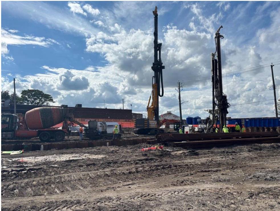
Photo 1: ECD installing CFA piles in the western part of site (facing northwest)
