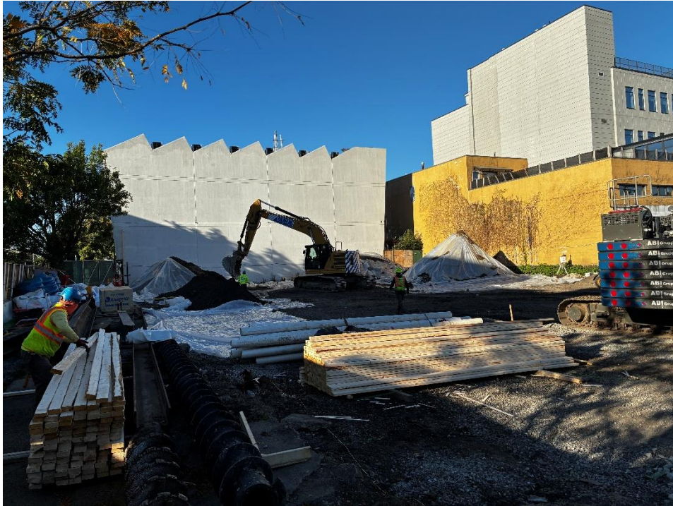
Photo 1: ECD consolidating drilling spoils stockpiles in the southern part of the site (facing south)
