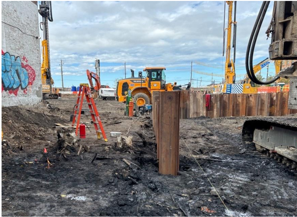
Photo 1: ECD installing sheet piles in the central part of site (facing north)
