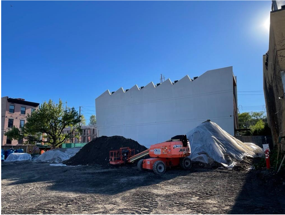
Photo 1: Stockpiled non-native fill generated during CFA advancement area in the southern part of the site (facing south)
