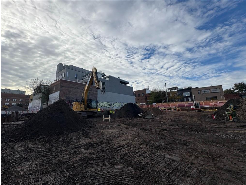
Photo 3: General view of the southwestern part of the site (facing south)
