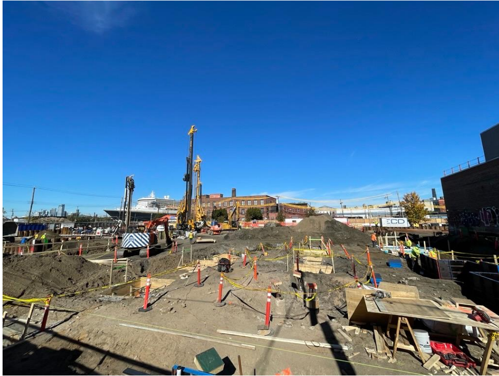
Photo 1: General view of the site (facing north)
