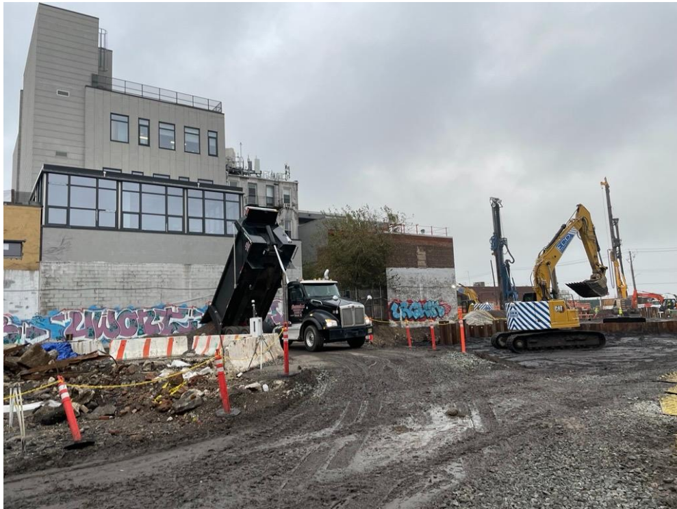
Photo 1: ECD importing 3/4-inch recycled clean stone (facing west)
