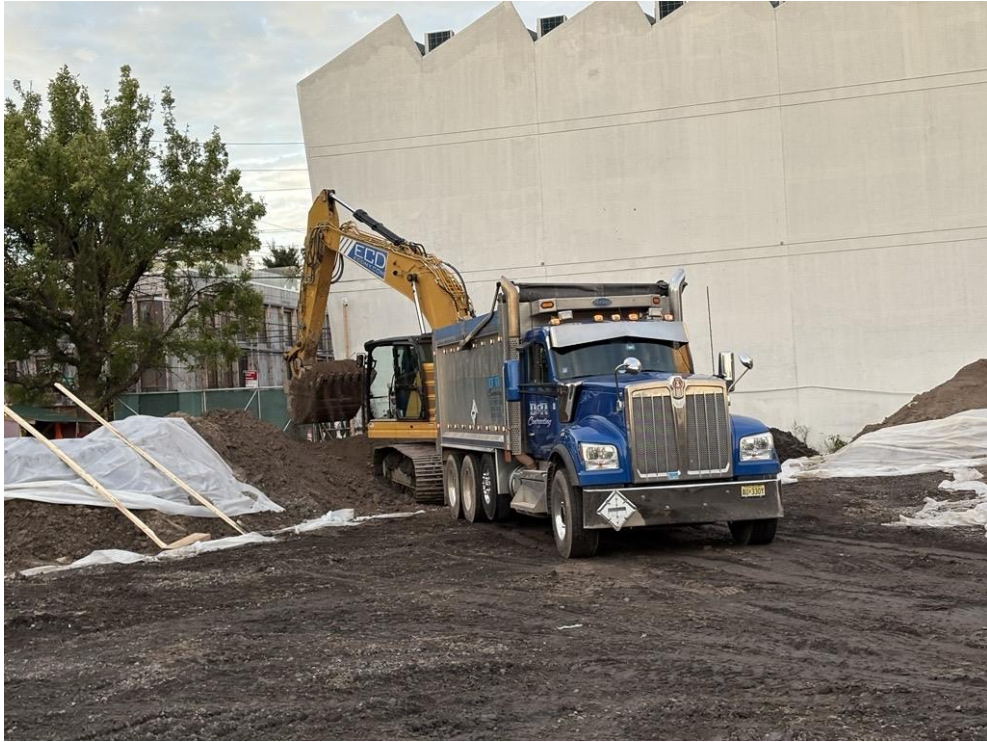
Photo 1: ECD live-loading stockpiled non-hazardous non-native fill into tri-axle trucks for off-site disposal (facing south)
