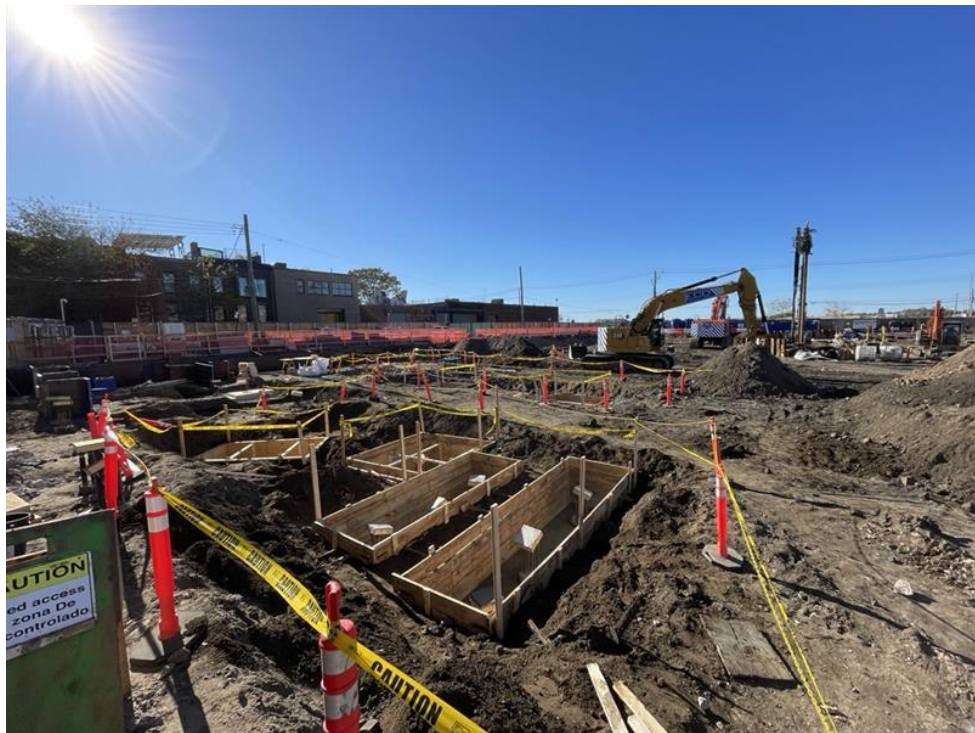
Photo 2: Excavated area to crush/form pile caps (facing west)
