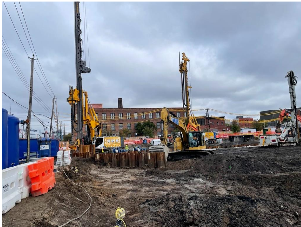
Photo 2: ECD installing CFA piles in the northern part of the site (facing northeast)
