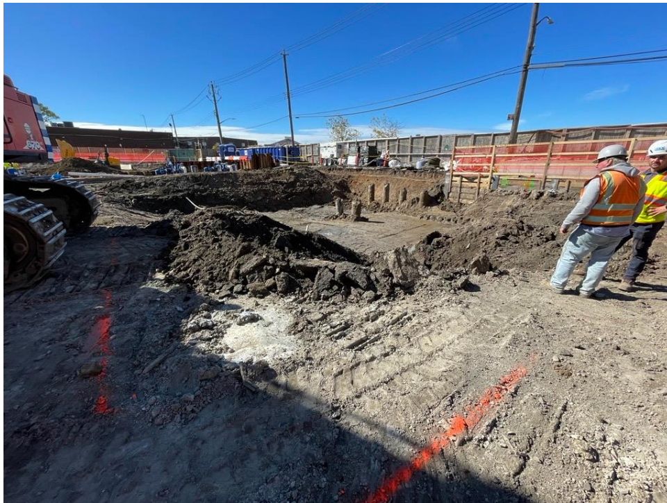
Photo 2: Excavated area in the northern part of the site (facing west)
