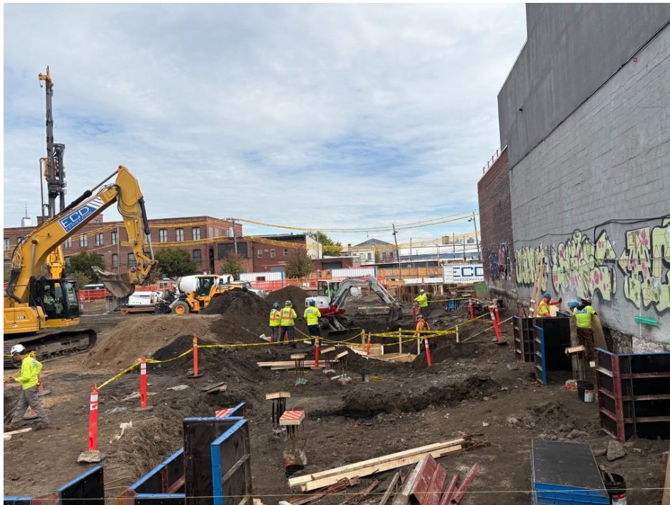
Photo 2: ECD excavating to crush/form pile caps (facing northeast)
