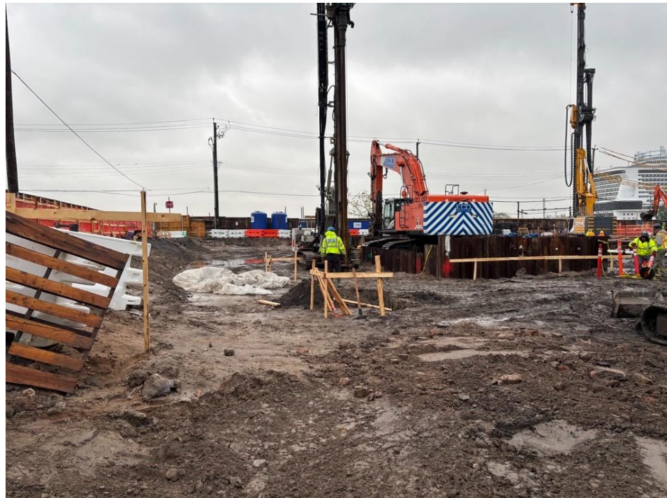
Photo 2: ECD installing CFA piles in the northern part of the site (facing north).
