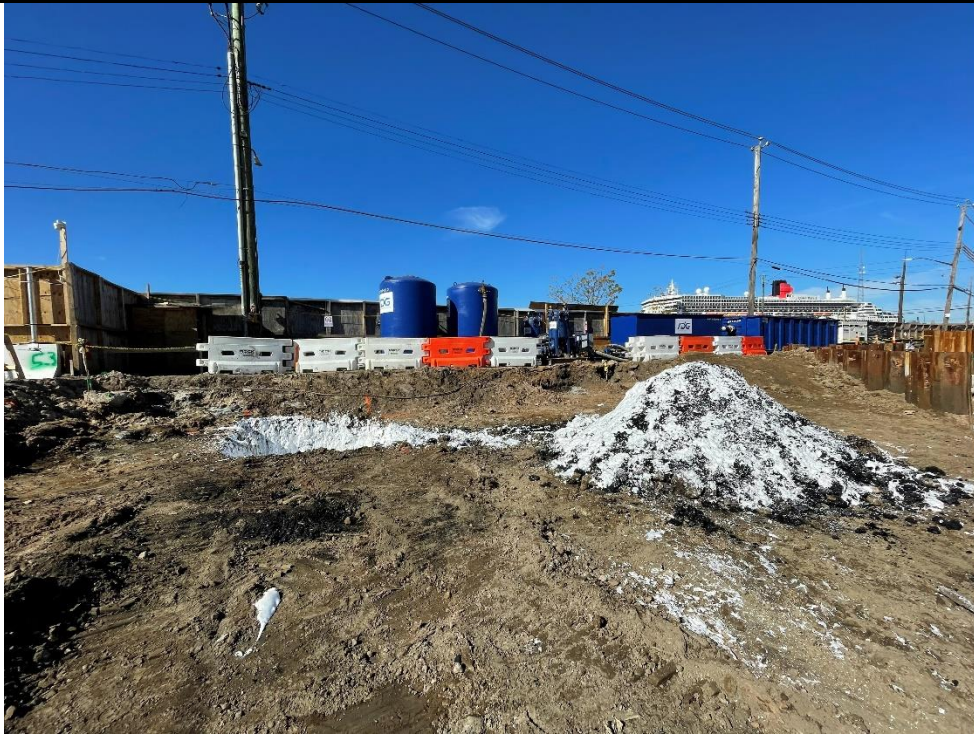
Photo 3: Odor suppressing foam over open excavation and stockpiled non-native fill in the northern part of the site (facing northwest)
