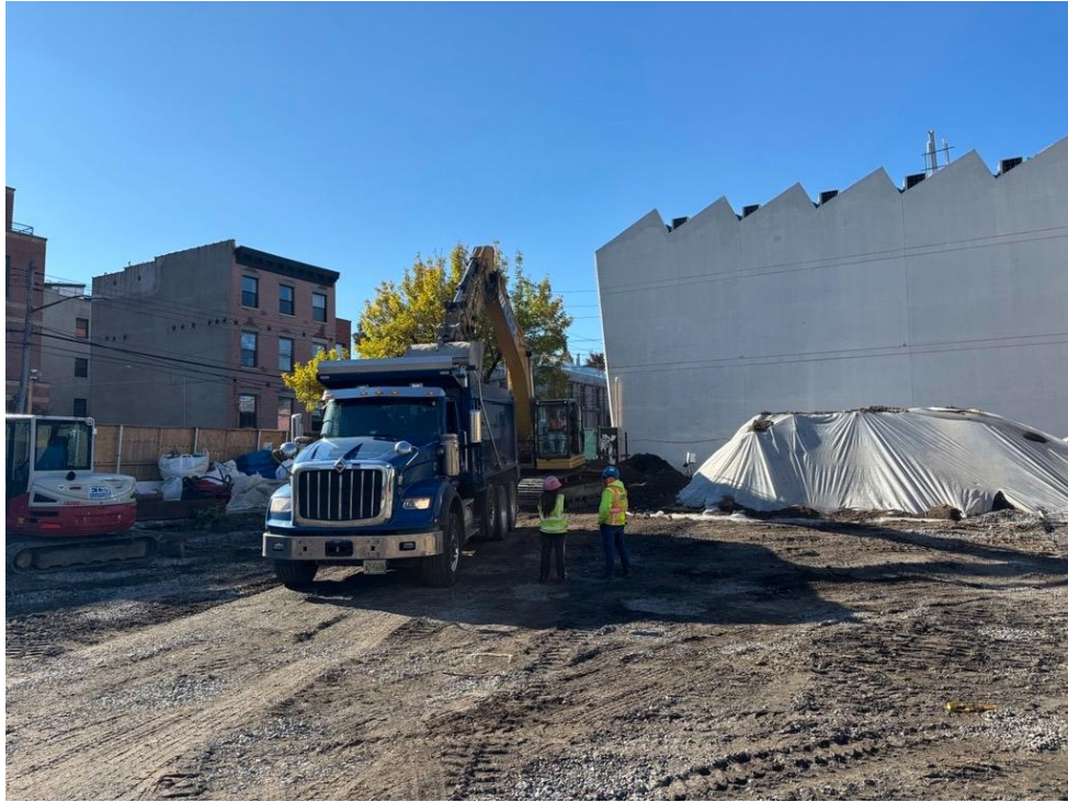
Photo 1: ECD live-loading non-hazardous non-native fill into triaxle trucks for off-site disposal in the southern part of the site (facing south)
