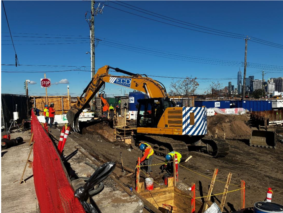
Photo 1: ECD excavating non-hazardous non-native fill in the western part of the site (facing northwest)
