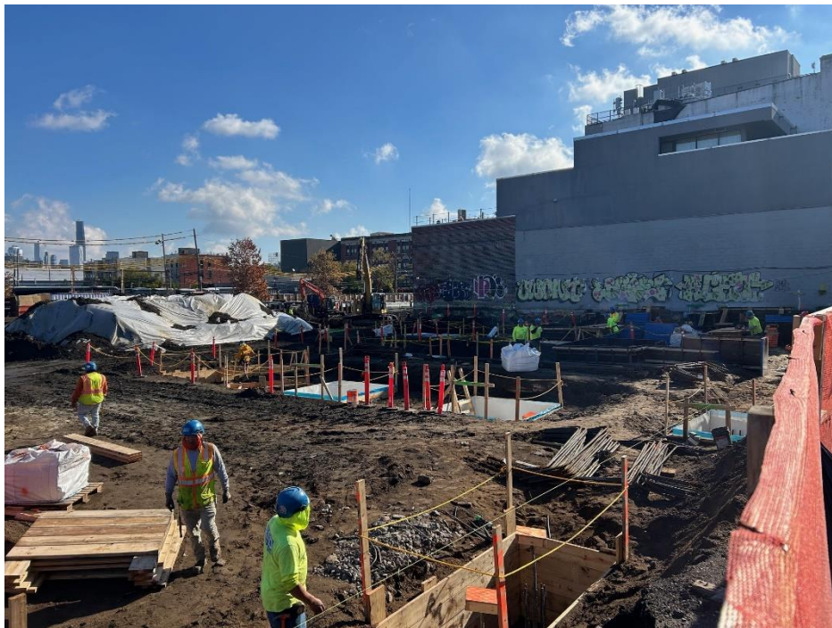
Photo 4: ECD installing formwork for pile caps in the western part of the site (facing southeast)
