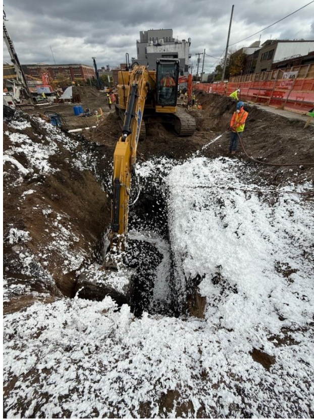
Photo 3: Odor suppressing foam applied to an open excavation and stockpiled non-native fill in the northern part of the site (facing northwest)
