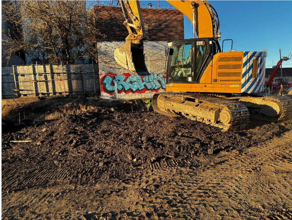
Photo 3: ECD excavating in central part of site. (facing southwest)
