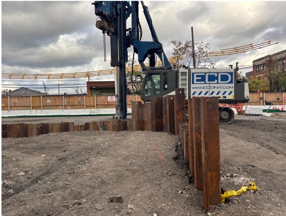
Photo 1: ECD advancing sheet piles in the central part of the site (facing east)
