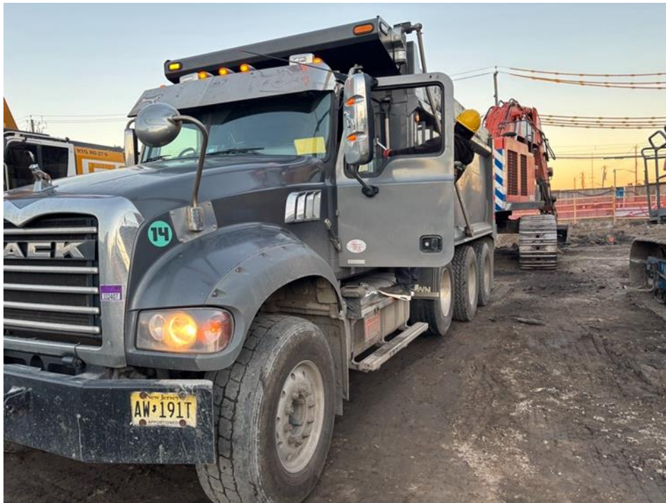
Photo 2: ECD live-loading non-hazardous non-native fill into triaxle trucks in the western part of the site for off-site disposal (facing west)
