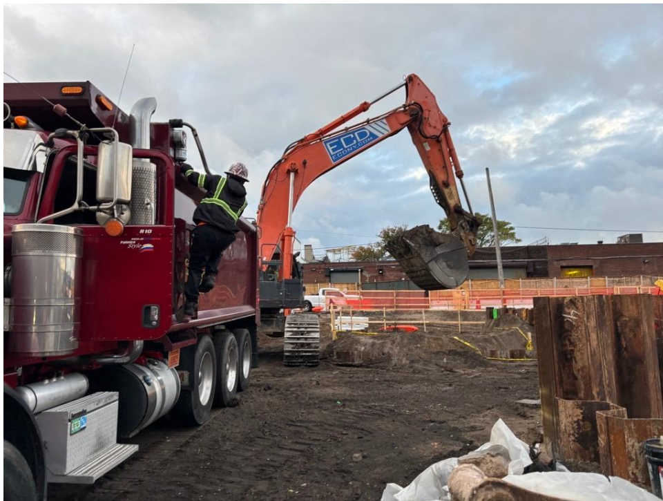
Photo 2: ECD live-loading non-hazardous fill into triaxle trucks in the western part of the site for off-site disposal (facing west)
