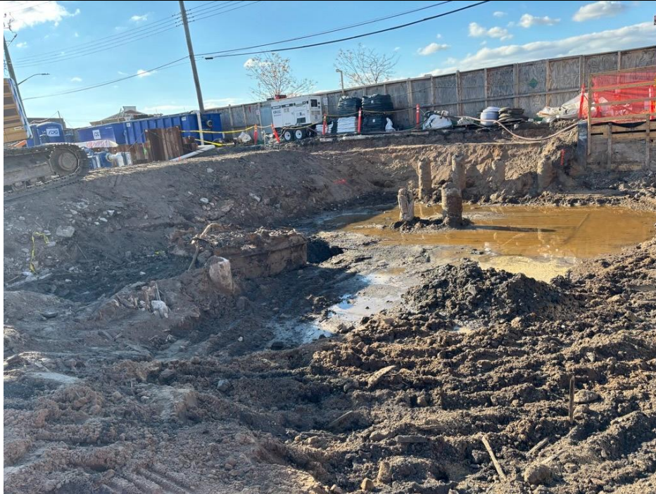
Photo 3: General view of the northern remedial excavation area in the northern part of the site (facing northwest)
