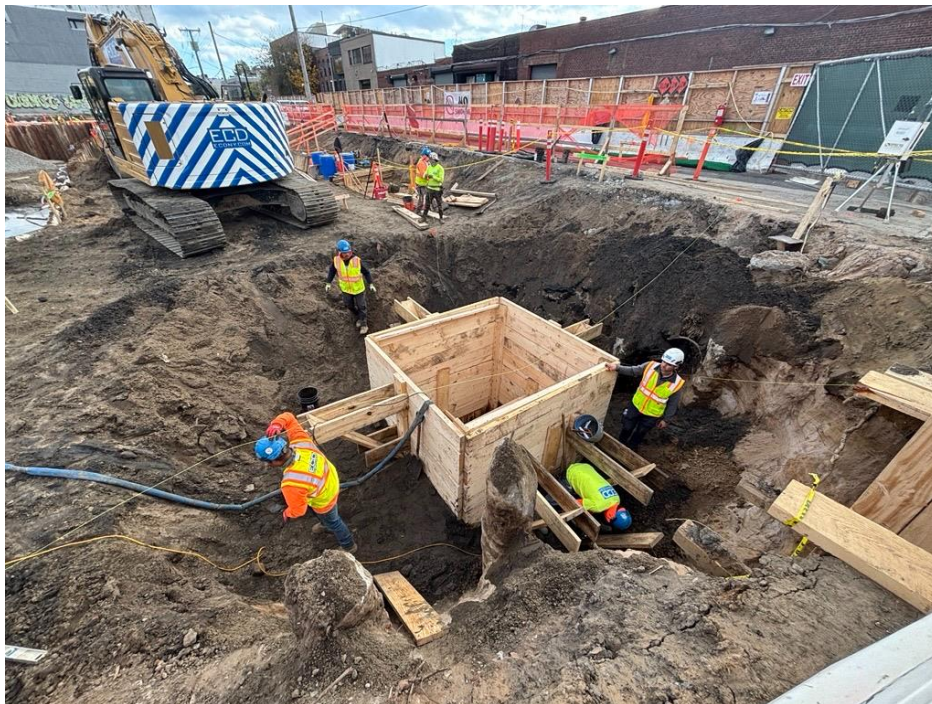
Photo 4: ECD installing formwork for house trap in the northwestern part of the site (facing southwest)
