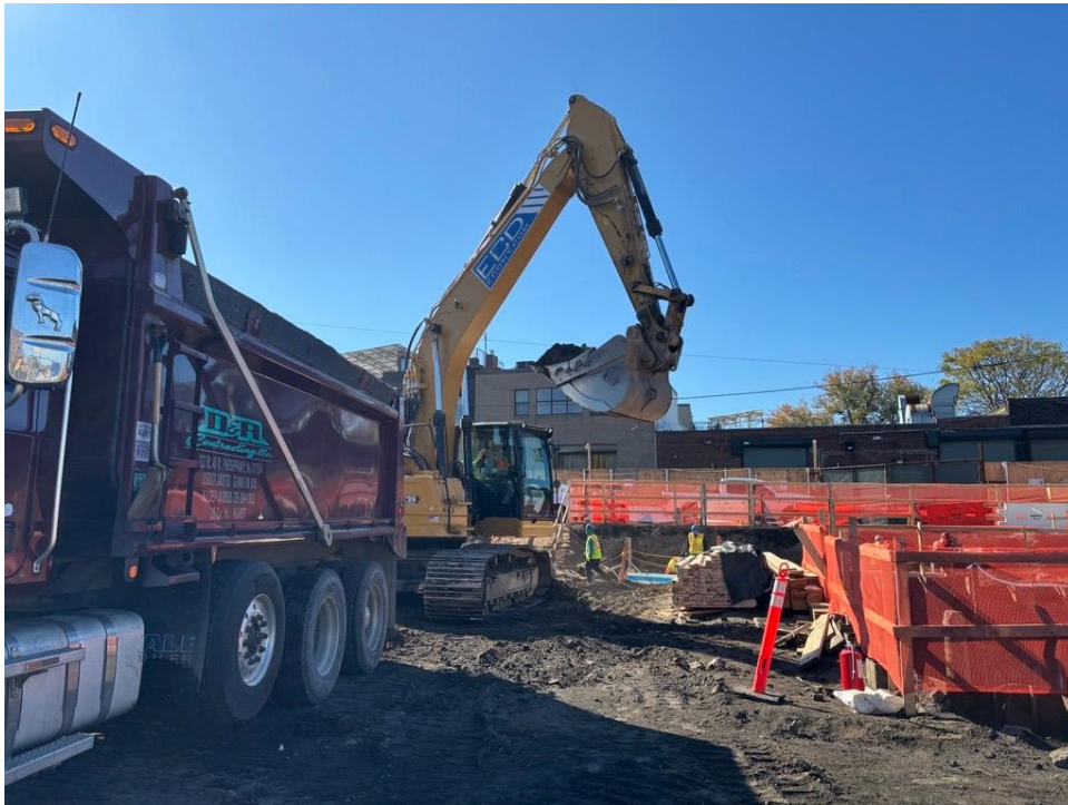
Photo 1: ECD live-loading non-hazardous non-native fill into triaxle trucks in the western part of the site for off-site disposal (facing west).
