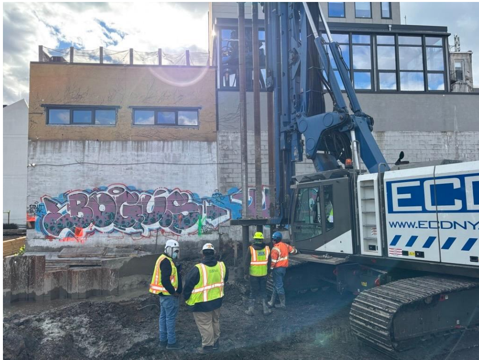
Photo 2: ECD advancing soil mix wall columns in the central part of the site (facing west)
