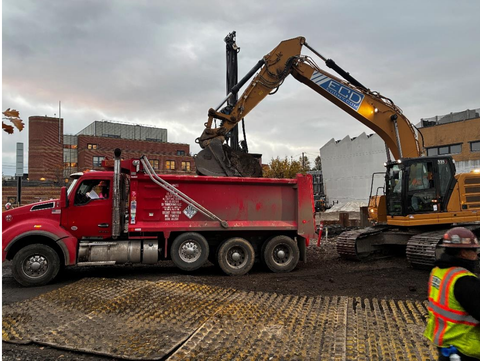
Photo 3: ECD loading non-native fill for off-site disposal (facing south).
