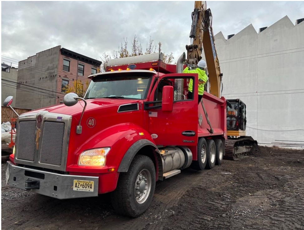
Photo 1: ECD loading stockpiled hazardous non-native fill into tri-axle trucks in the southern part of site (facing west).
