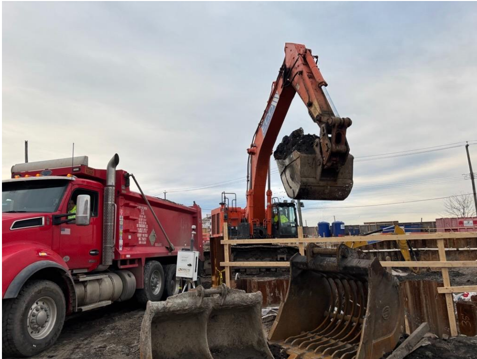
Photo 2: ECD live-loading non-hazardous non-native fill into tri-axle trucks for off-site disposal (facing northwest)
