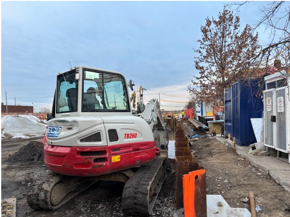
Photo 4: ECD excavating non-native fill in the eastern part of the site (facing north)
