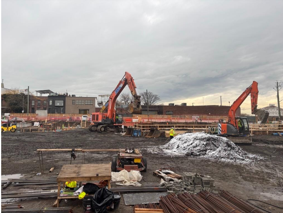
Photo 3: ECD applying odor suppressing foam to exposed non-native fill in the northern part of the site (facing west)
