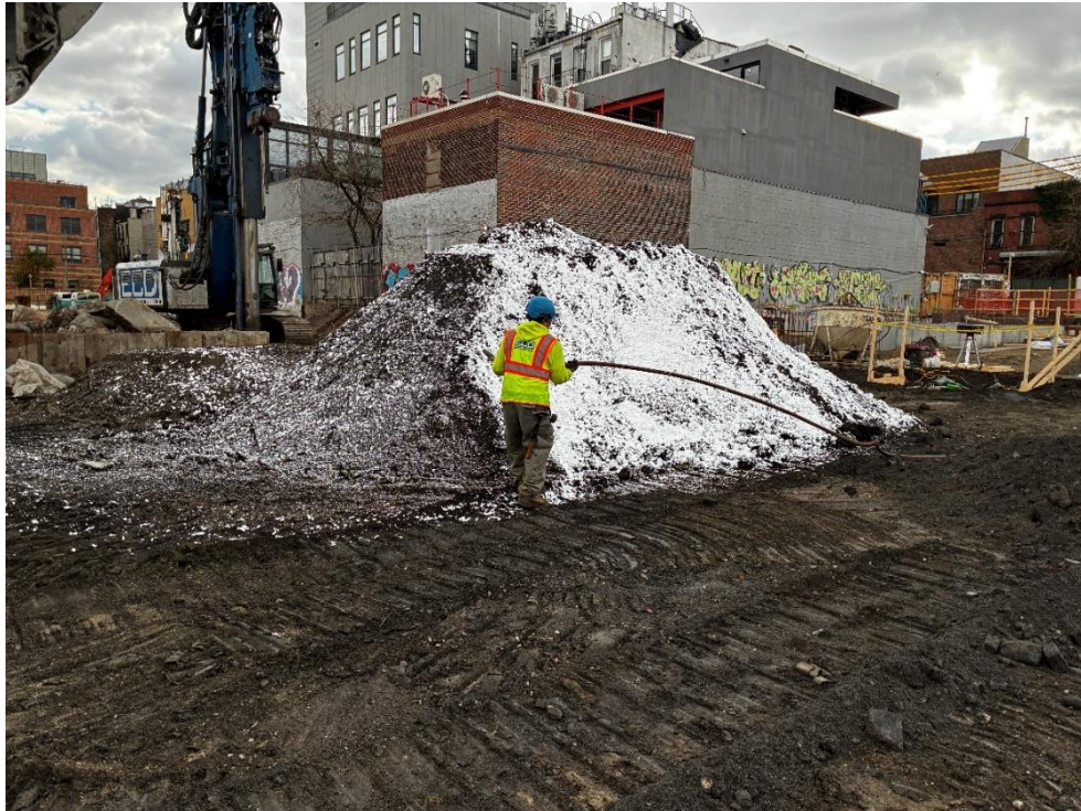
Photo 2: ECD applying odor suppressing foam in the central part of the site (facing south).
