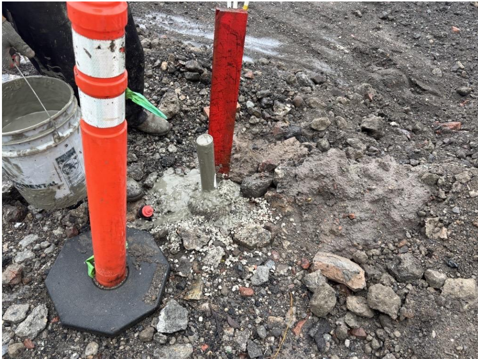
Photo 4: Decommissioned monitoring well MW-014 in the southern part of the site
