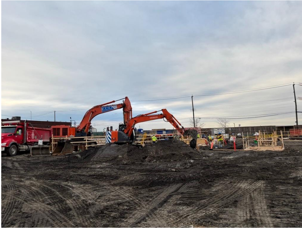
Photo 1: ECD excavating for pile cap installation in the northern part of the site (facing north).
