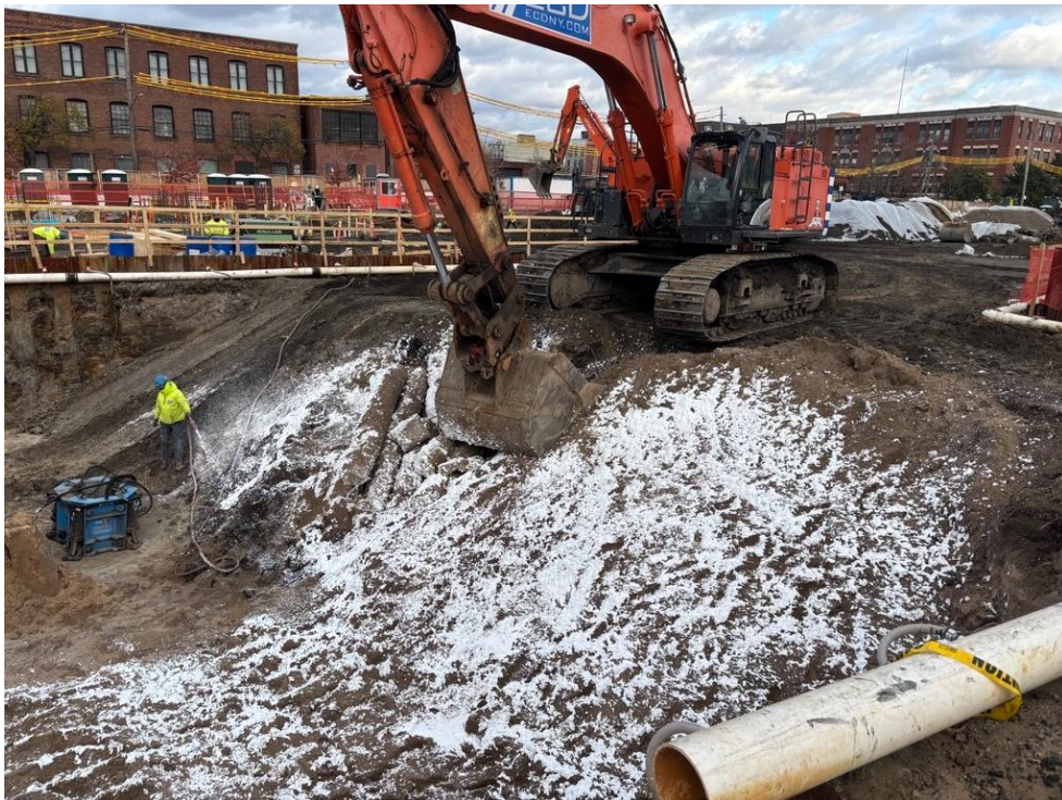
Photo 4: ECD applying odor suppressing foam to exposed non-native fill in the western part of the site (facing east).
