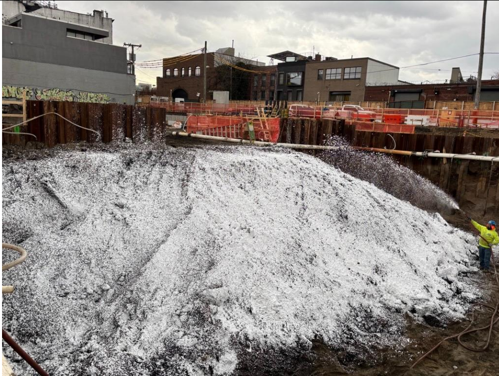
Photo 3: ECD applying odor suppressing foam to exposed non-native fill during live loading in the western part of the site (facing southeast)
