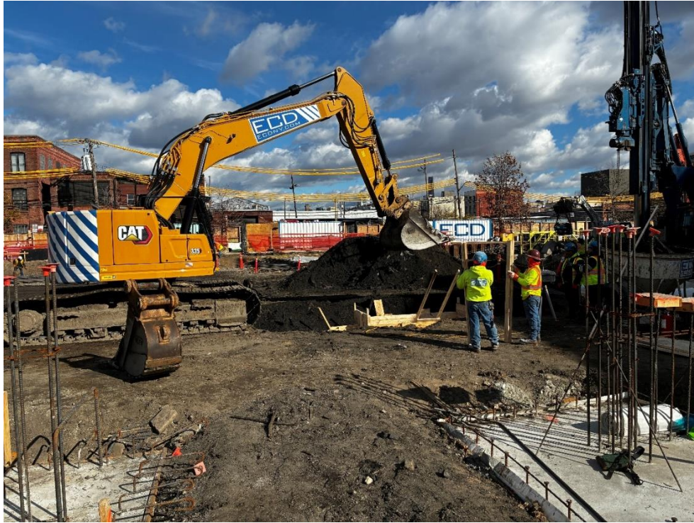
Photo 1: ECD excavating non-native fill in the central part of site (facing northeast.).
