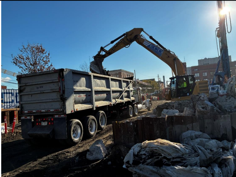
Photo 3: ECD loading C&D material into a truck for off-site disposal. (facing southeast)
