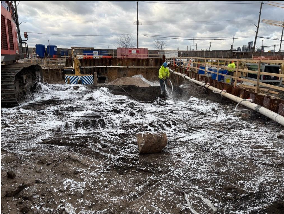
Photo 3: ECD applying odor suppressing foam to exposed non-native fill in the western part of the site (facing north)
