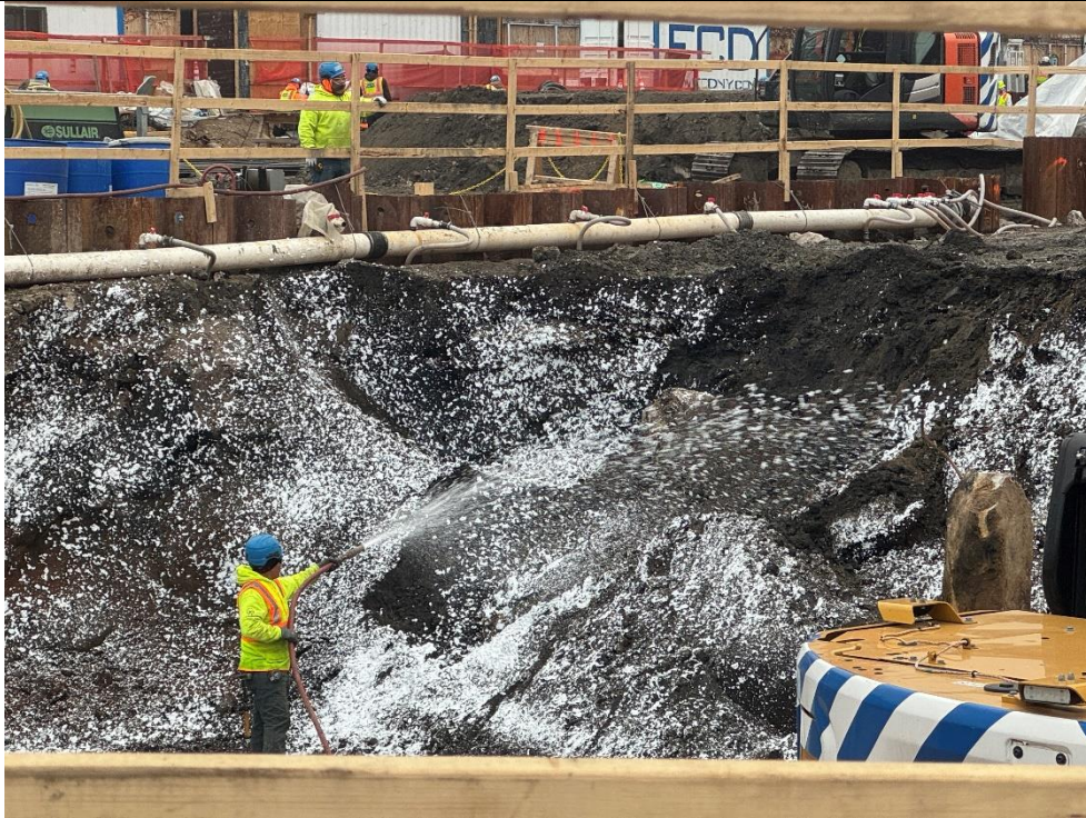
Photo 3: ECD applying odor suppressing foam to exposed non-native fill during live loading in the western part of the site (facing northeast)
