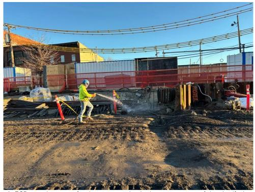
Photo 2: ECD spraying water for dust suppressing in the western part of the site (facing east).
