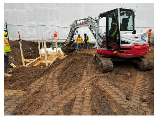
Photo 2: ECD construction pile cap forms in the southern part of the site (facing north).
