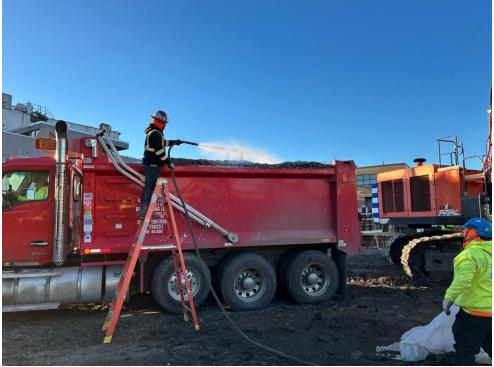
**Photo 3:** ECD applying odor suppressing foam to non-hazardous non-native fill loaded into tri-axle trucks prior to off-site disposal (facing west).
