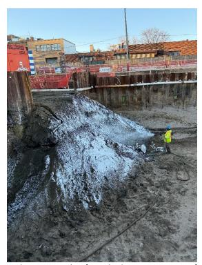
Photo 2: ECD applying odor suppressing foam in the western part of the site (facing west).
