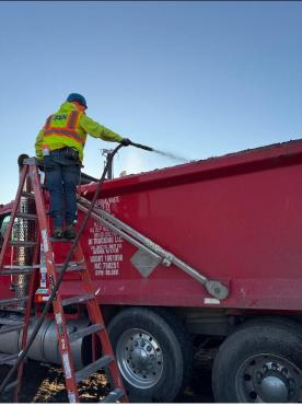
**Photo 3:** ECD applying odor suppressing foam to non-hazardous non-native fill loaded into tri-axle trucks prior to off-site disposal (facing west).
