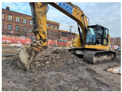
Photo 1: ECD excavating non-native fill in the northern part of site (facing east).
