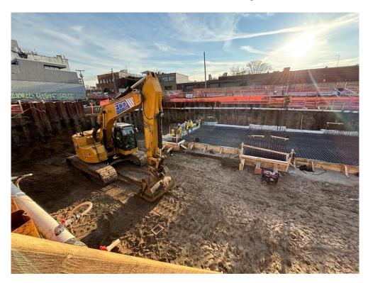
**Photo 4:** ECD installing rebar atop waterproofing/vapor barrier membrane within the detention tank area in the western part of the site (facing west).
