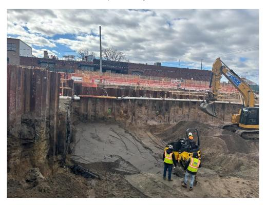
Photo 4: ECD grading bucket-mixed PetroFix and in-situ non-native fill in the western part of the site (facing west)
