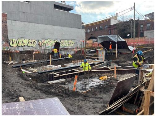
Photo 2: ECD installing formwork for electrical trenches in the western part of the site (facing southwest).
