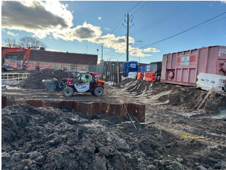
Photo 2: CFA pile spoils in the northwestern part of the site (facing west)
