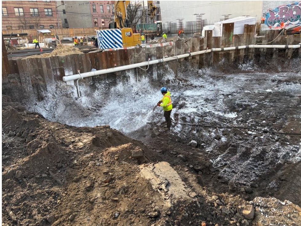
Photo 4: ECD spraying pneumatic foam unit NTC / 8 to apply odor control foam in the eastern part of the site (facing southeast)
