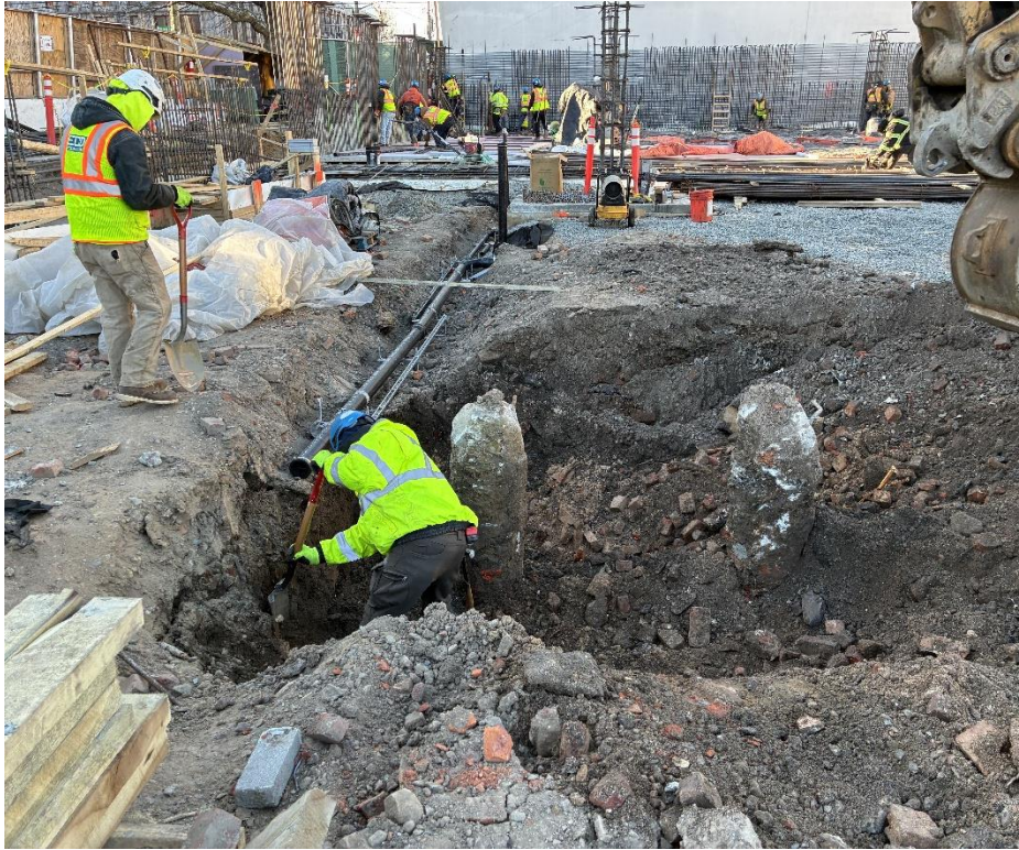
Photo 1: Pile cap excavation in the southeastern part of the site (facing south).
