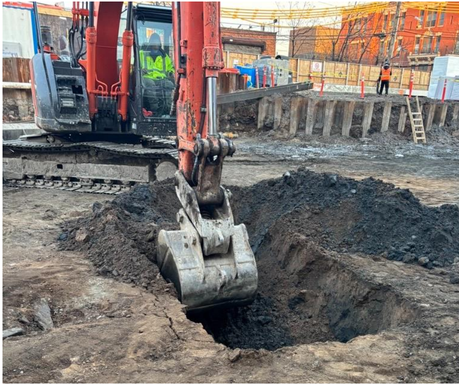
Photo 1: ECD excavating non-native fill in the central part of the site (facing east).
