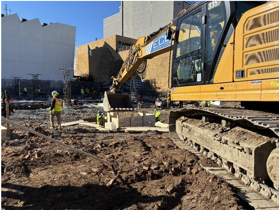
Photo 2: ECD installing forms in the excavations in the southeastern part of the site (facing south).
