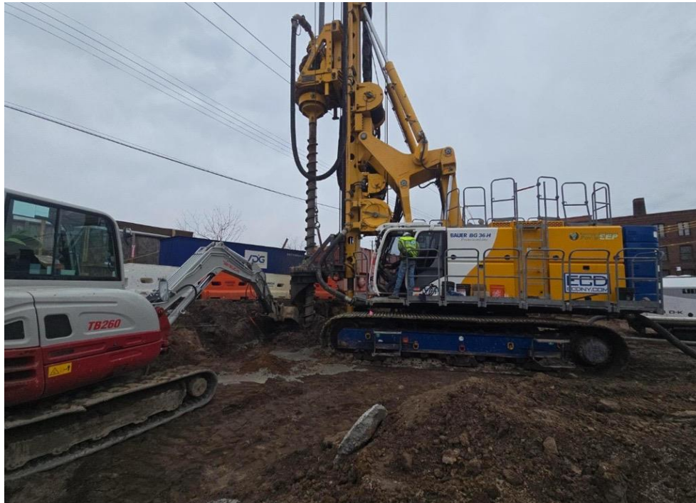
Photo 2: ECD advancing CFA piles in the northern part of the site (facing north)
