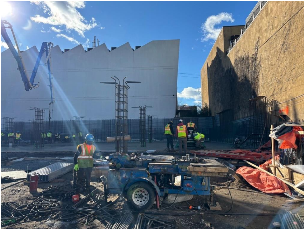
Photo 4: ECD pouring a concrete slab as part of the SSD system in the southern part of the site (facing southwest)
