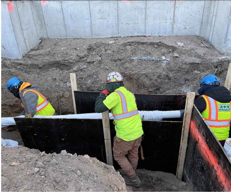
Photo 3: ECD installing SVE system components in the western part of the site (facing southeast)
