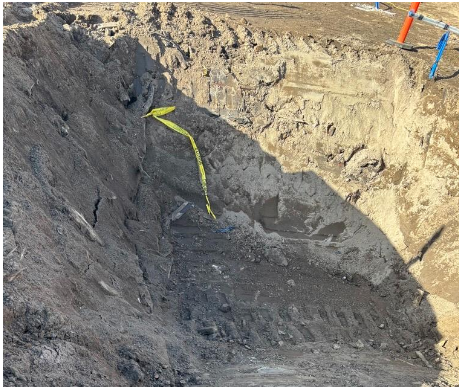
Photo 1: General excavation in the northern part of the site (facing north)
