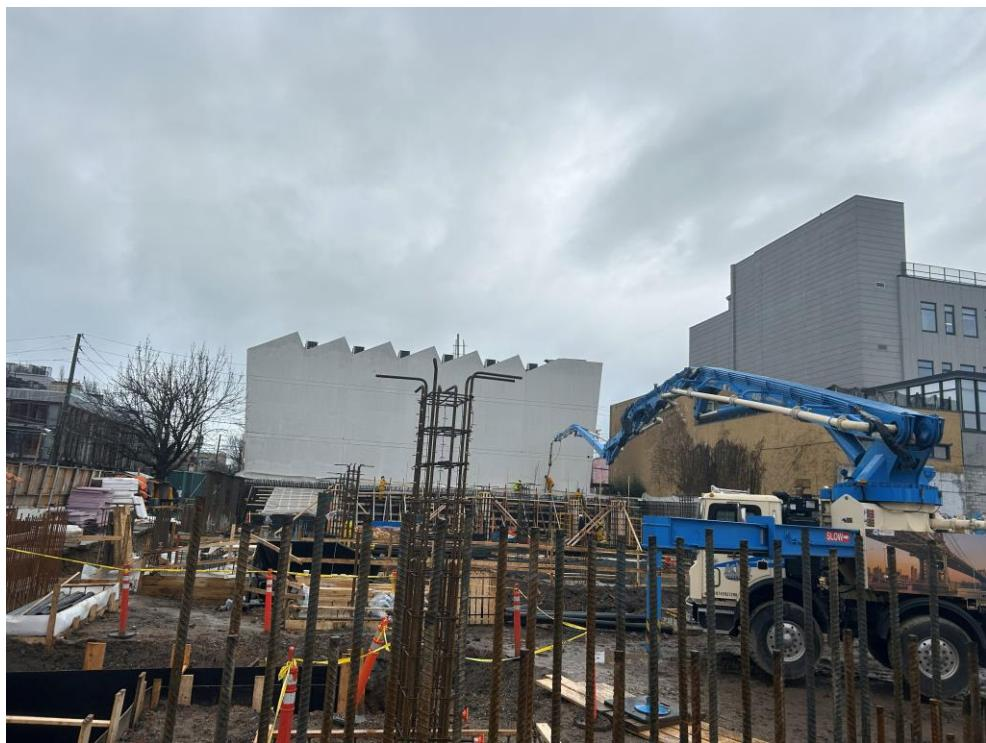
**Photo 1:** ECD pouring concrete within the southern part of site (facing southwest)
