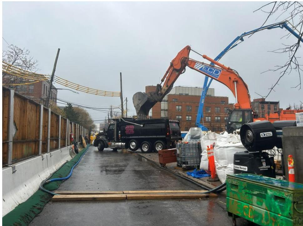
**Photo 2:** ECD live-loading non-hazardous non-native fill in the southeastern part of the site into tri-axle trucks for off-site disposal (facing southeast)
