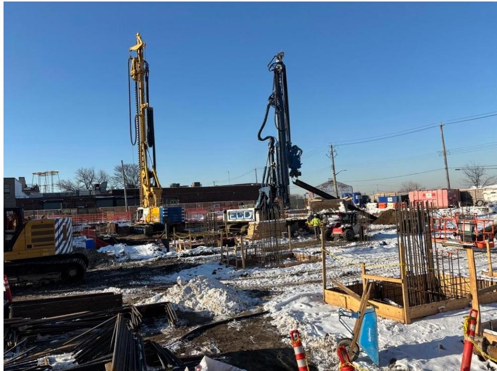
**Photo 4:** ECD advancing CFA piles in the western part of the site (facing south)
