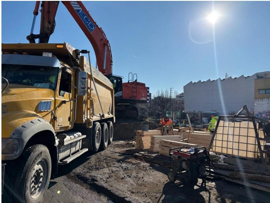
**Photo 2:** ECD loading stockpiled non-hazardous non-native fill in the southeastern part of the site into triaxle trucks for off-site disposal (facing south)
