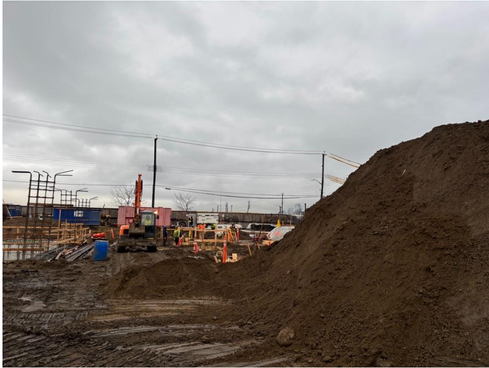
Photo 1: ECD excavating non-native fill to install foundation elements within the northwestern part of site (facing north)
