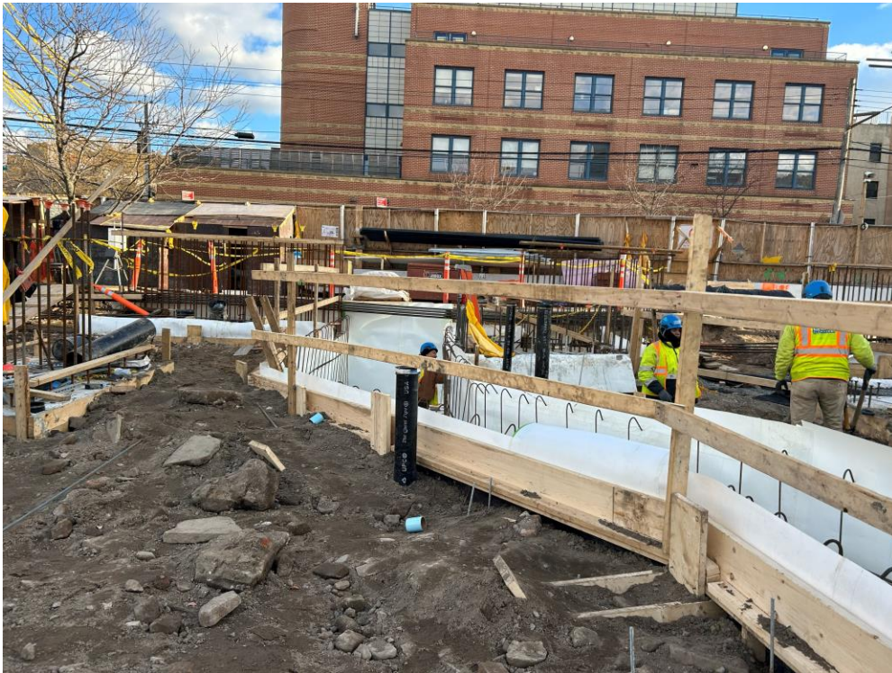
Photo 1: ECD installing waterproofing in the southern part of site for utility pit installation (facing southeast)
