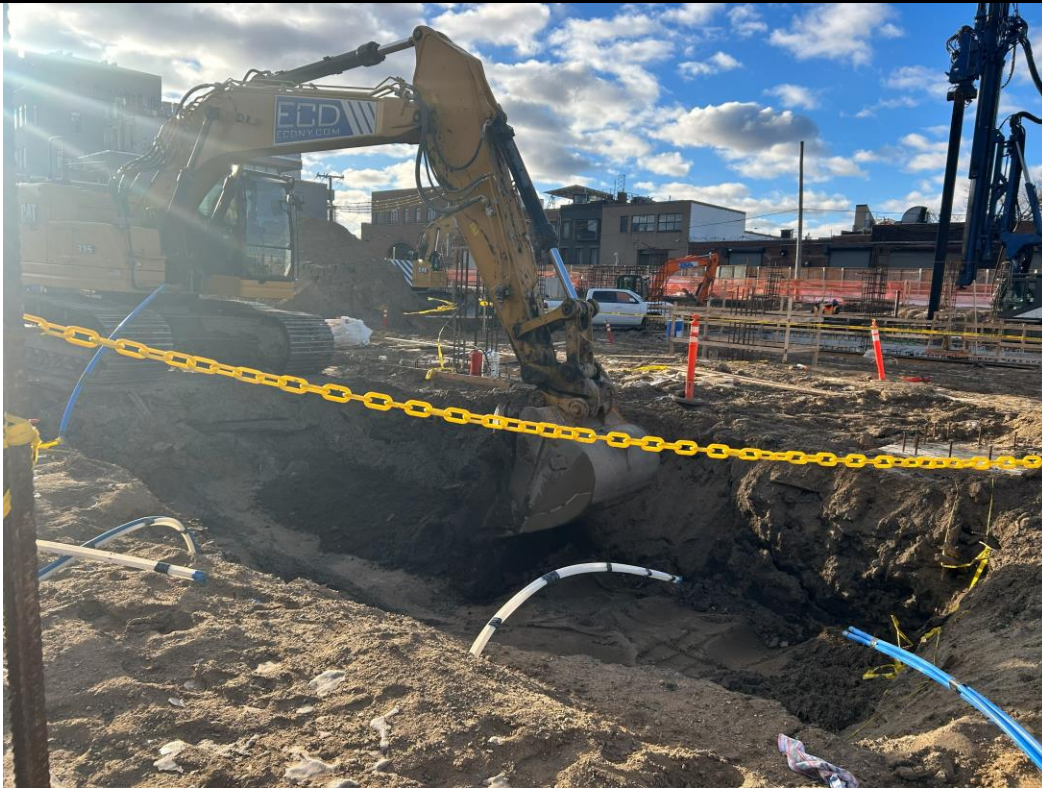
Photo 3: ECD backfilling with previously imported clean fill in the northern part of the site (facing west)
