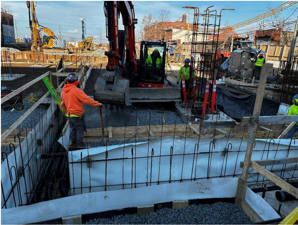
Photo 1: ECD using Kubota KX080-4α2 to backfill with ATSM No. 5 stone in the southern part of site (facing northeast)
