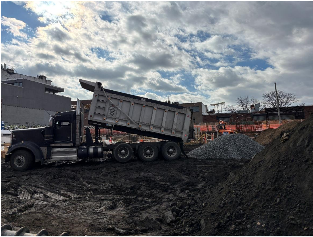
Photo 1: ECD importing ATSM No. 5 stone in the central part of site (facing southwest)
