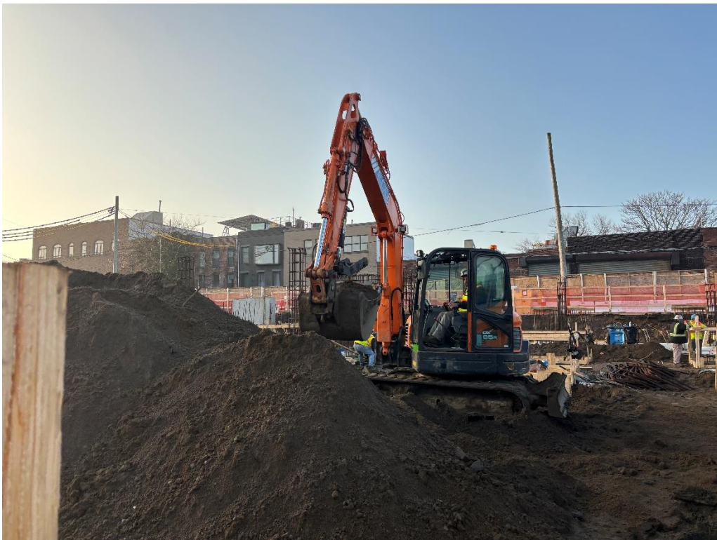
Photo 4: ECD excavating for pile cap installation in the northwestern part of site (facing southwest)
