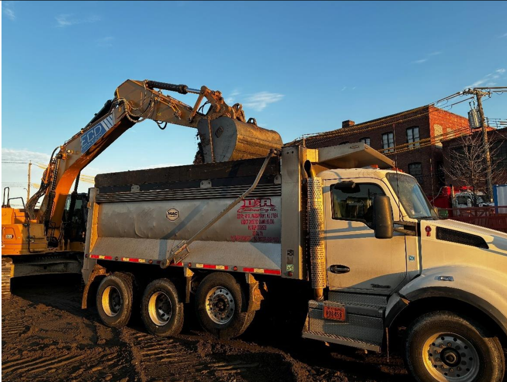
Photo 3: ECD loading tri-axle trucks with non-hazardous low pH non-native fill for off-site disposal (facing east)
