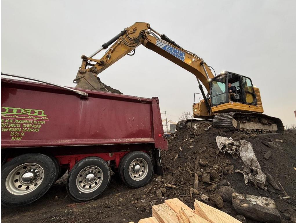
Photo 3: ECD loading trucks with non-hazardous non-native fill for off-site disposal (facing east)
