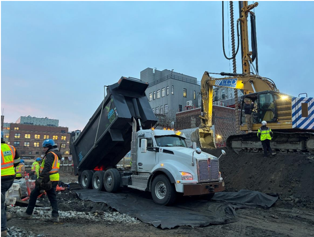
Photo 1: ECD importing clean fill in the eastern part of site (facing south)
