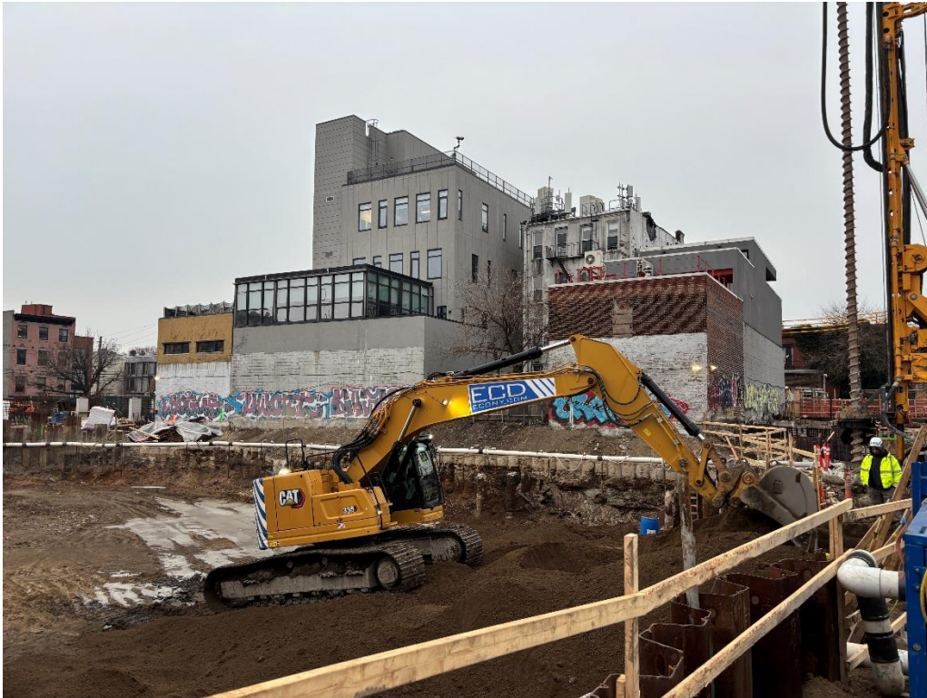
Photo 2: ECD backfilling with imported clean fill in the eastern part of site (facing southwest)
