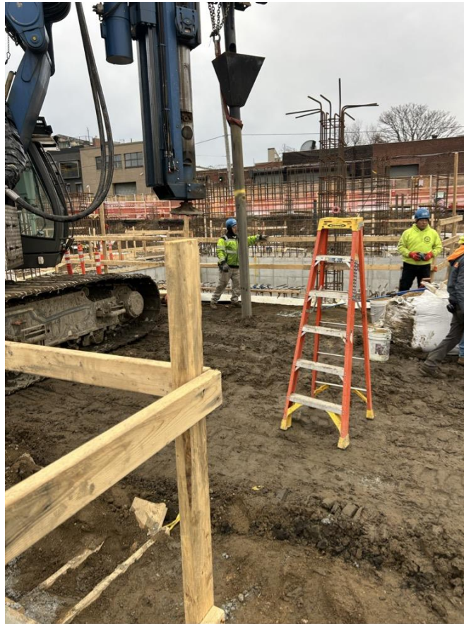
Photo 1: ECD advancing a PetroFix injection point in the southern part of the site (Area 3)
