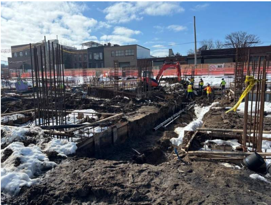
Photo 2: ECD excavating non-hazardous non-native fill in the western part of the site (facing west)
