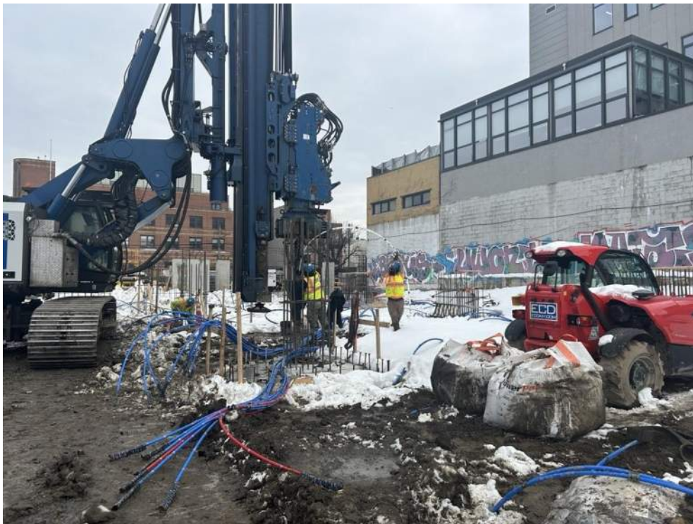
Photo 4: ECD installing the injection points in Treatment Area 2 in the eastern part of site (facing south)
