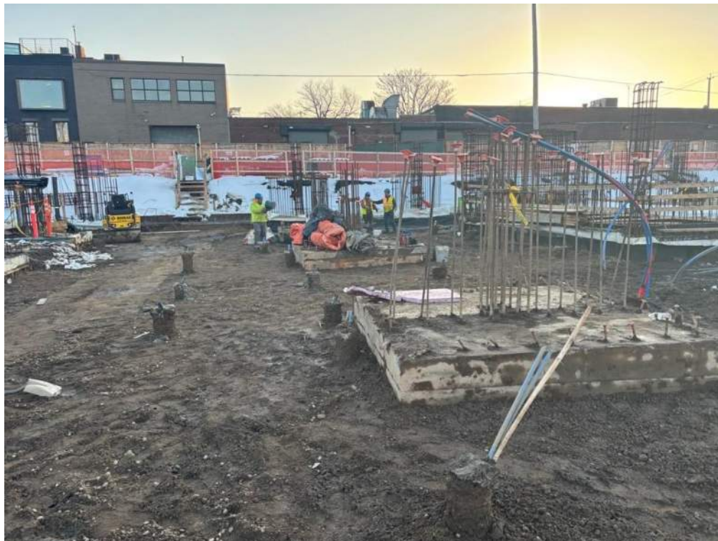
Photo 4: ECD excavating in the western part of the site (facing west)
