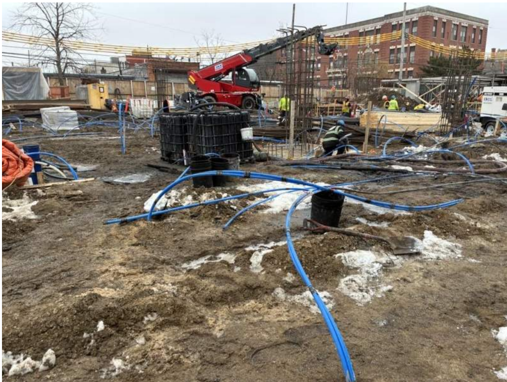
Photo 4: ECD injecting PetroFix in Treatment Area 2 in the central part of the site (facing east)
