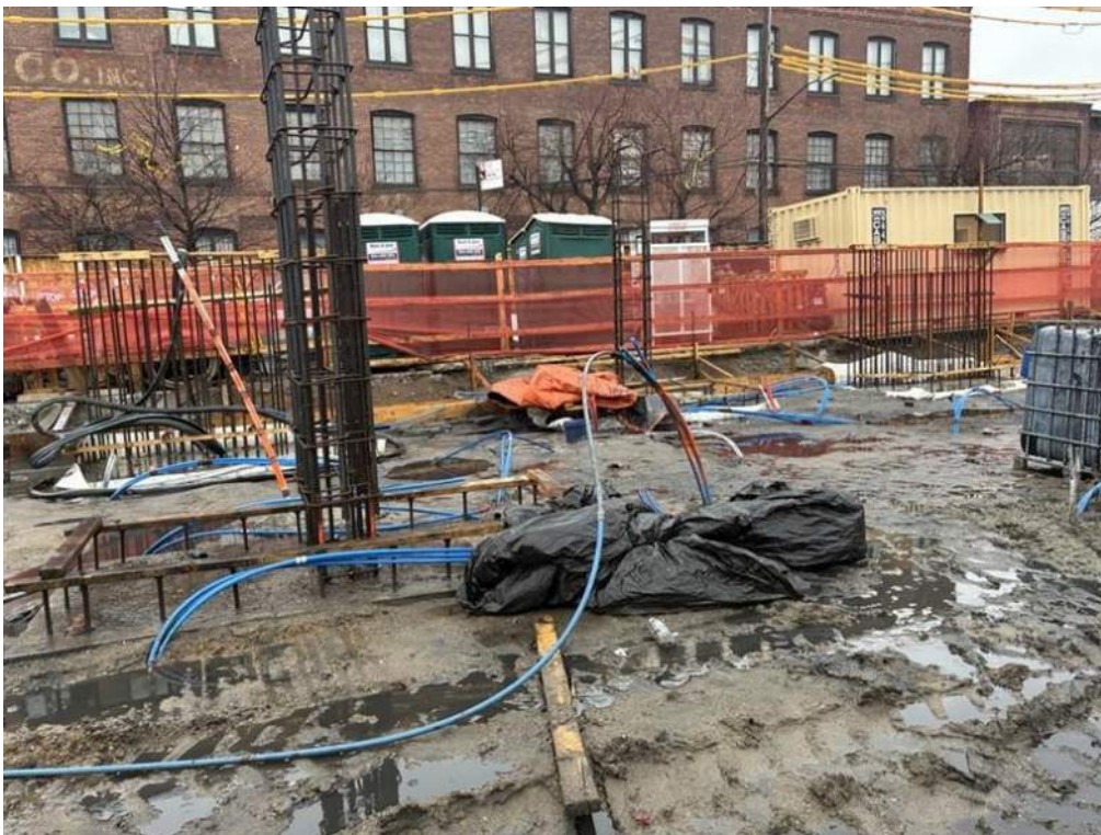
Photo 2: ECD injecting PetroFix within Treatment Area 1 in the northern part of the site (facing northeast)
