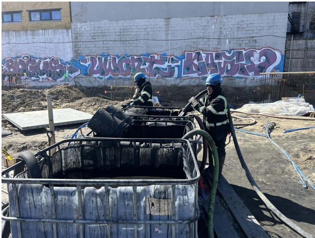
Photo 1: ECD injecting PetroFix in Treatment Area 2 within the central part of the site (facing south)
