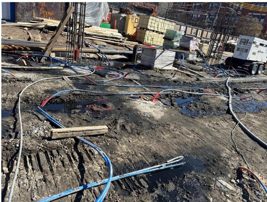
Photo 2: ECD injecting PetroFix in Treatment Area 2 within the central part of the site (facing southeast)
