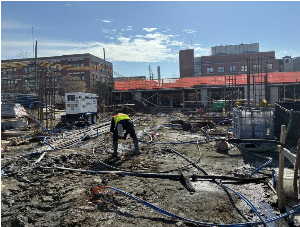
Photo 4: ECD injecting PetroFix in Treatment Area 2 within the central part of the site (facing southeast)
