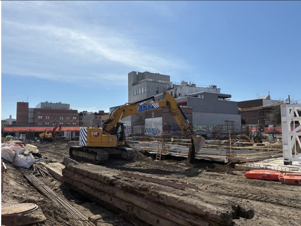
Photo 3: ECD grading non-native fill in the northwestern part of the site (facing southeast)
