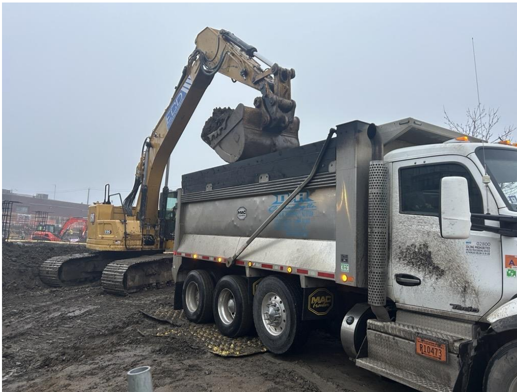
Photo 1: ECD loading a permitted tri-axle truck with stockpiled non-hazardous non-native fill in the northeastern part of the site (facing west)
