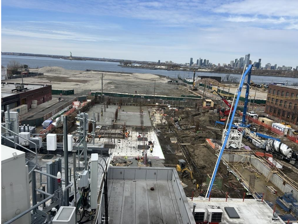
Photo 3: General view of the western part of the site (facing northwest)
