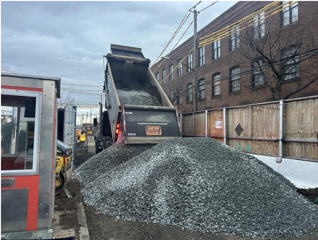
Photo 1: ECD importing 3/4-inch virgin stone in the eastern part of the site (facing northwest)
