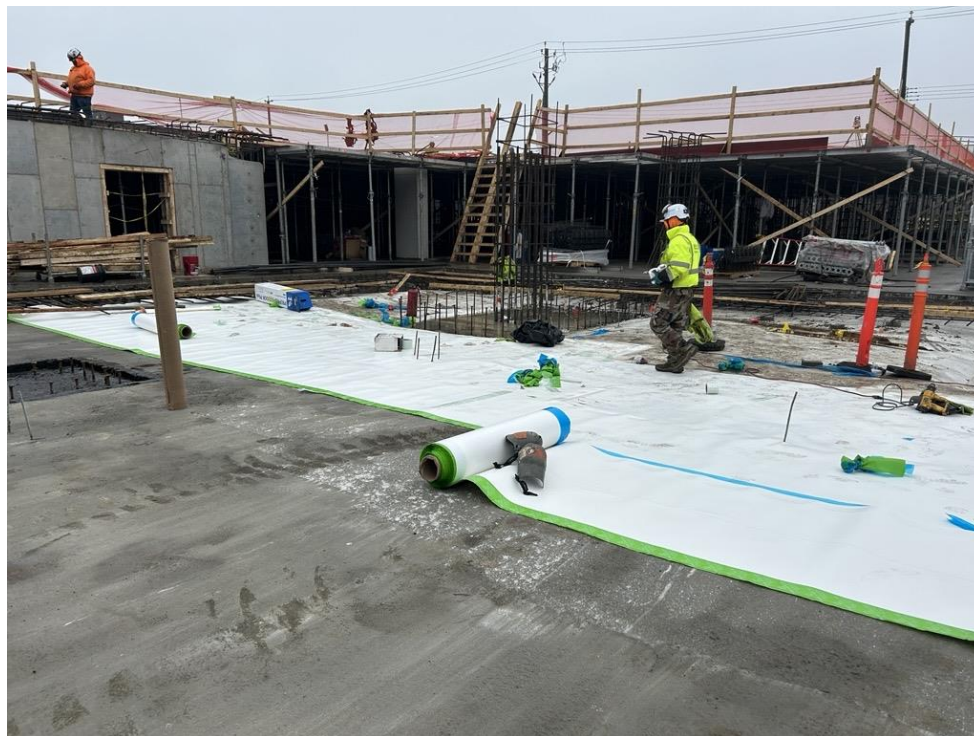
Photo 2: ECD installing Preprufe 300R Plus waterproofing/vapor barrier in the western part of the site (facing west)
