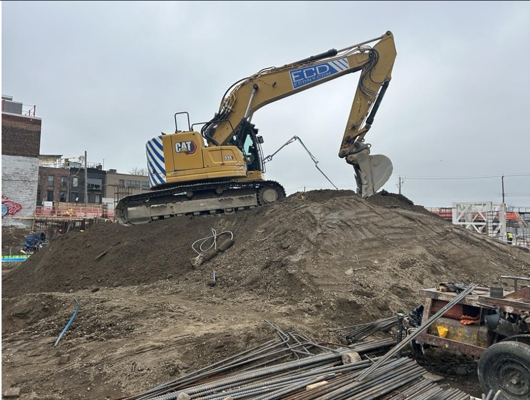
Photo 3: ECD stockpiling previously imported clean fill within the central part of the site (facing northwest)
