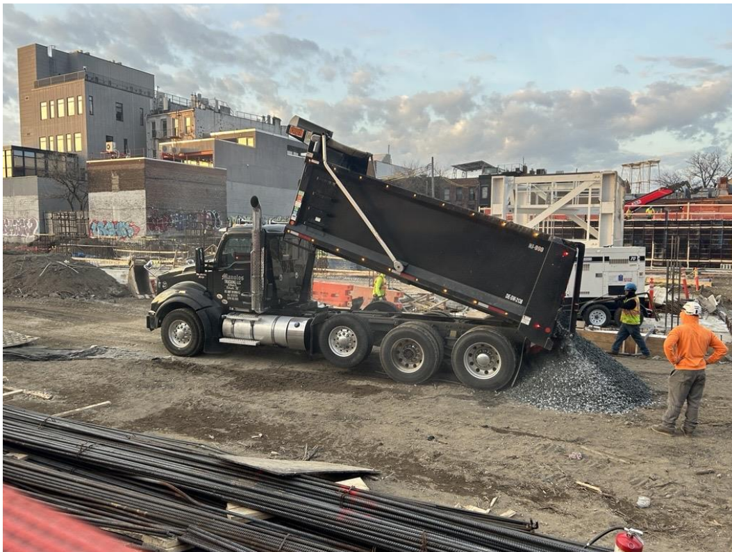
Photo 1: ECD importing ¾-inch virgin stone in the central part of the site (facing southwest)
