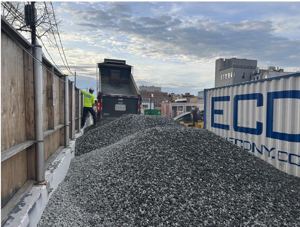
Photo 1: ECD importing ¾-inch virgin stone in the central part of the site (facing southeast)
