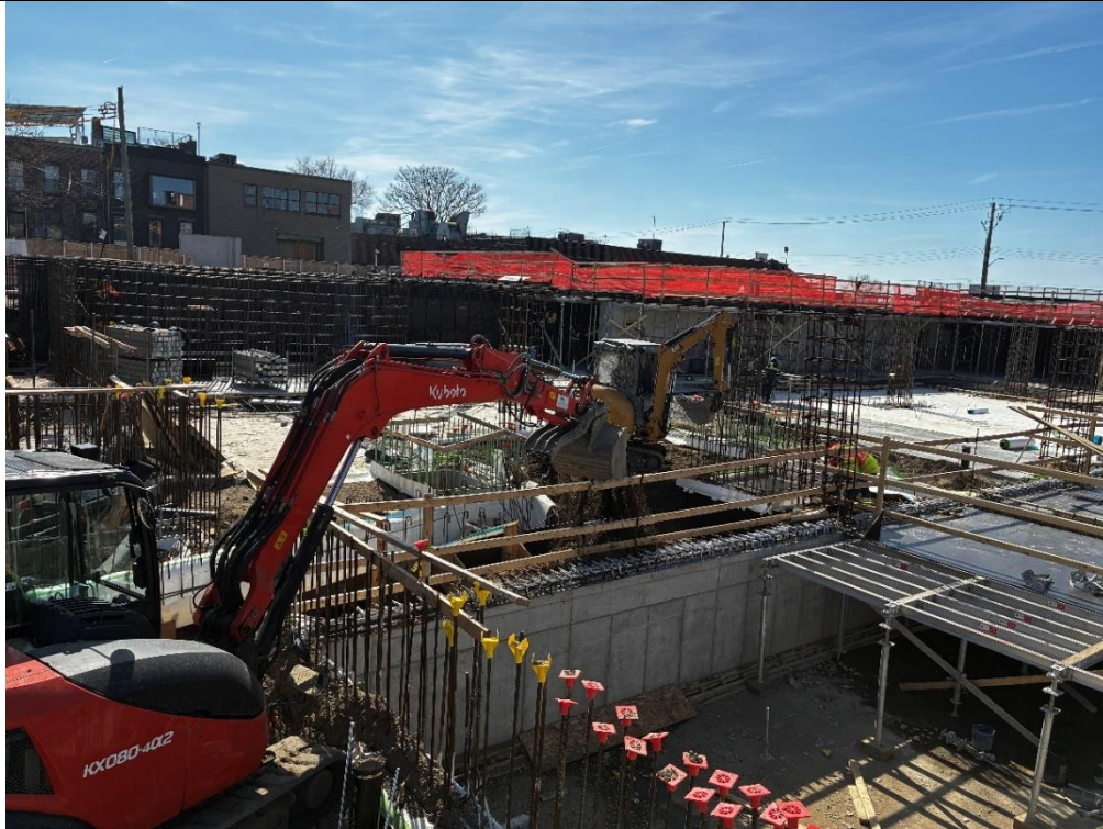
Photo 3: ECD using a Kubota KX080-4 \alpha 2 to backfill previously imported clean fill in the central part of the site (facing west)
