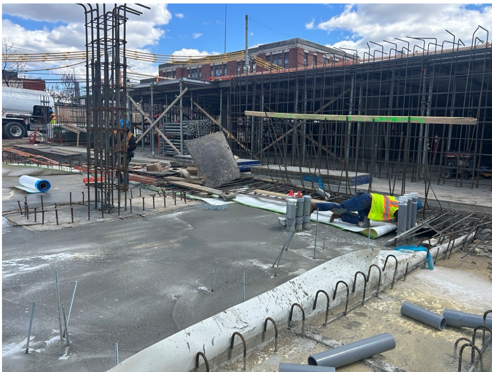
Photo 2: ECD installing Preprufe 300R Plus waterproofing/vapor barrier atop the rat slab in the central part of the site (facing east)
