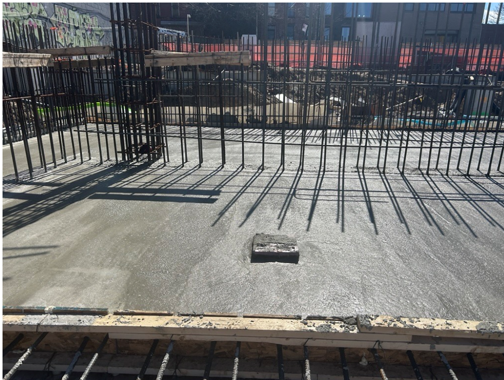
Photo 1: ECD installing a box-out within the slab for future monitoring point installation for the SSDS in the western part of site (facing southwest)
