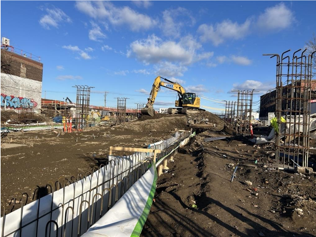
Photo 1: ECD stockpiling previously imported clean fill in the central part of the site for future backfill (facing northwest)
