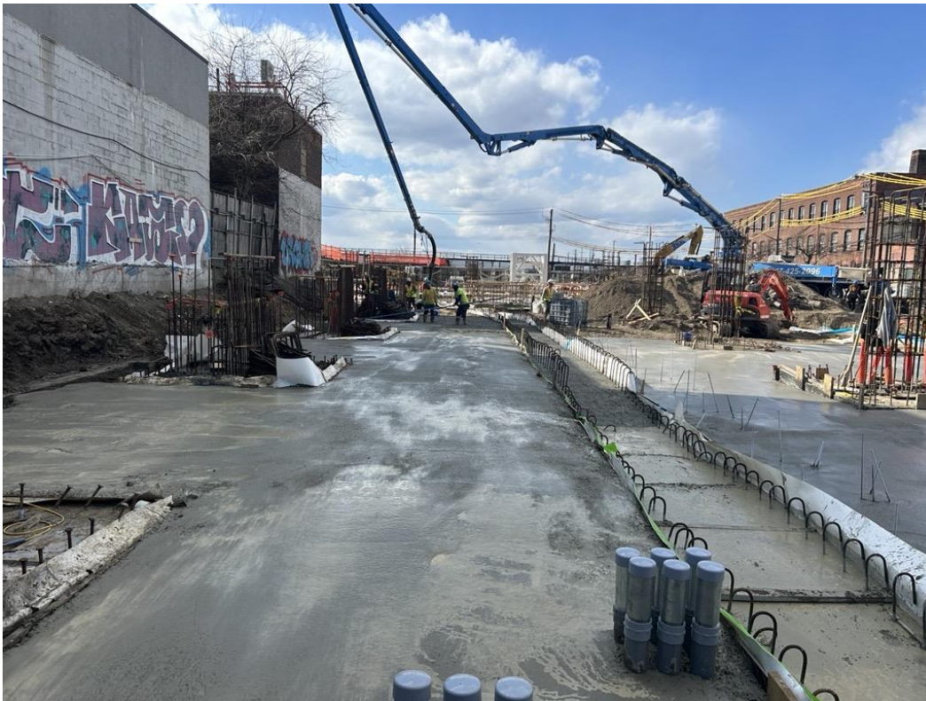
Photo 4: ECD pouring an about 3-inch-thick rat slab in the central part of the site (facing north)
