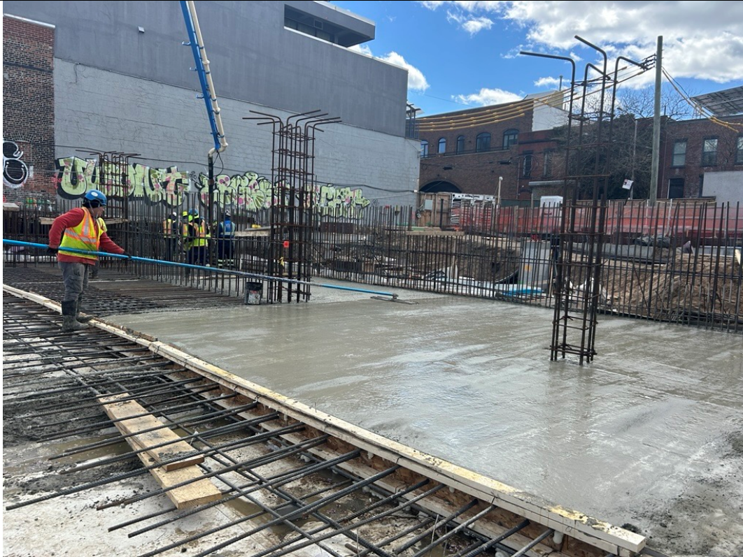
Photo 3: ECD pouring an about 12-inch-thick concrete slab within the western part of the site (facing south)
