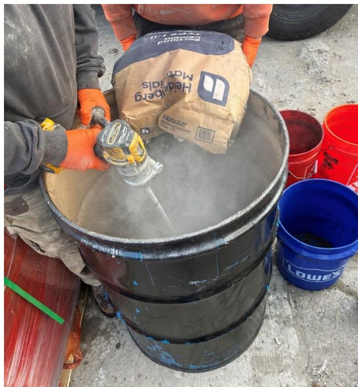
Photo 2: Coastal hand mixing grout for monitoring well decommissioning.
