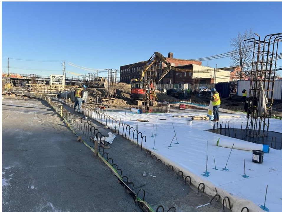
Photo 2: ECD installing Preprufe 300R Plus waterproofing/vapor barrier atop the rat slab in the central part of the site (facing north)
