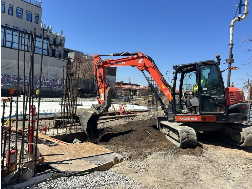
Photo 3: ECD backfilling with previously imported clean fill in the central part of the site (facing west)
