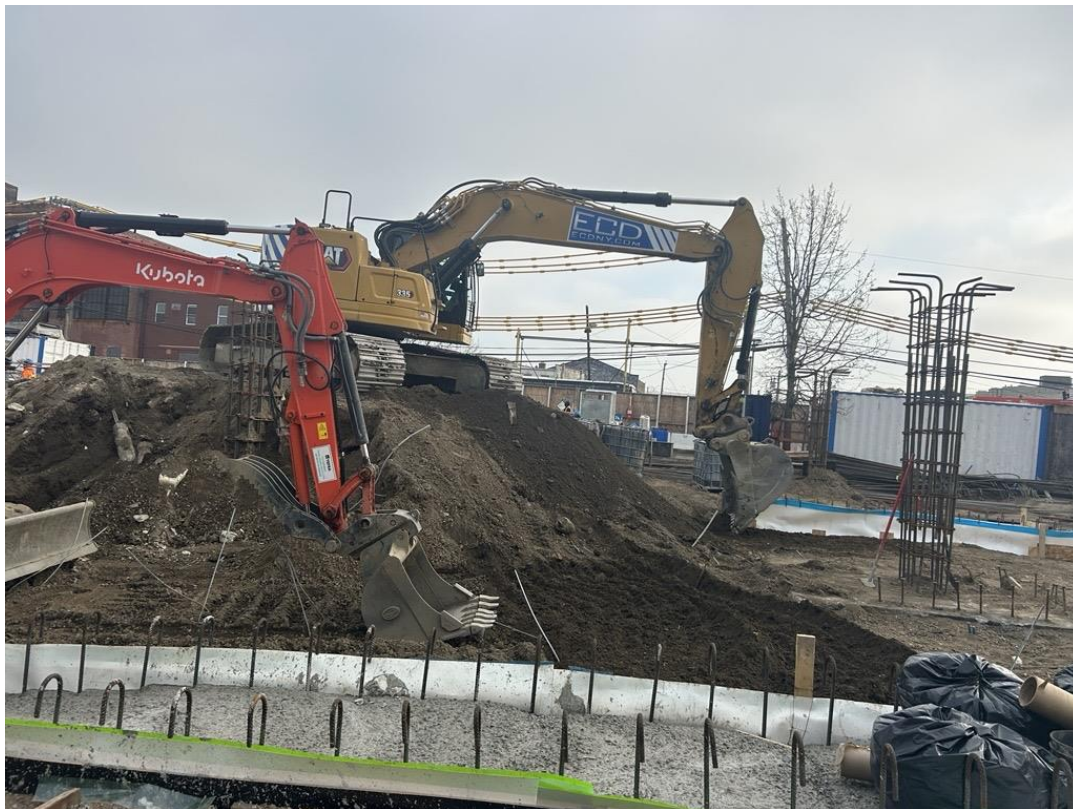
Photo 1: ECD grading previously imported clean fill in the central part of site (facing east)
