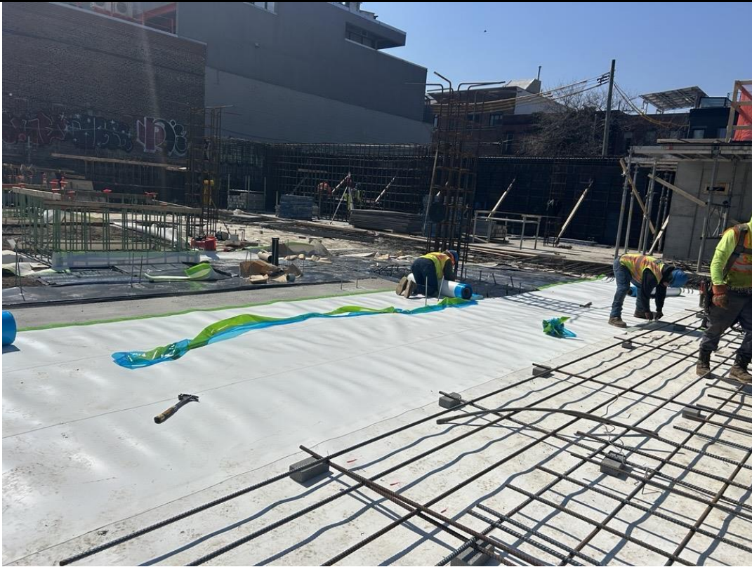
Photo 3: ECD installing Preprufe 300R Plus waterproofing / vapor barrier in the western part of the site (facing south)
