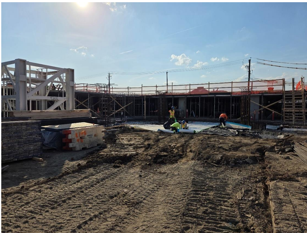
Photo 2: ECD installing Preprufe 300R Plus waterproofing/vapor barrier in the northern part of the site (facing west).
