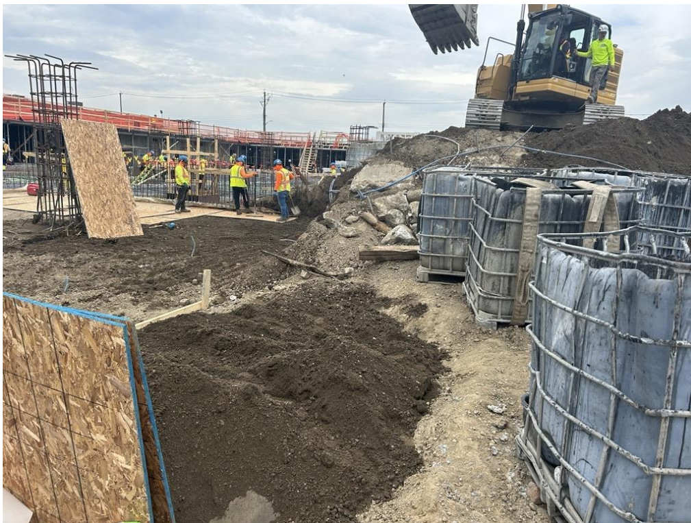
Photo 2: ECD backfilling previously imported clean fill in the central part of the site (facing west)
