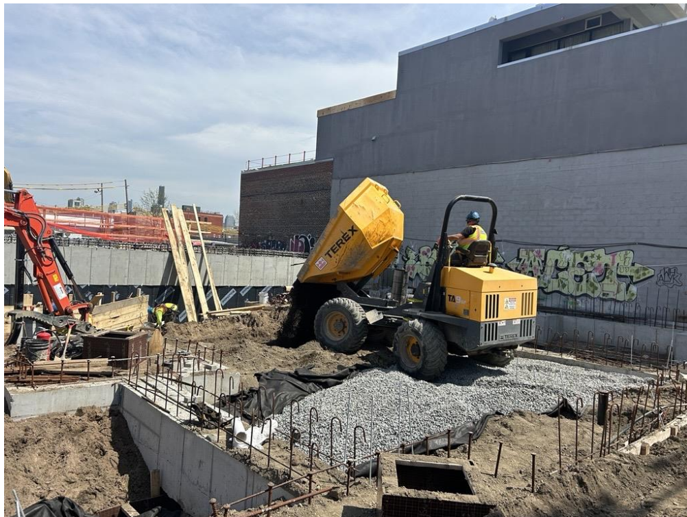
Photo 4: ECD stockpiling previously imported clean fill from the eastern part of the site in the western part of the site (facing east)
