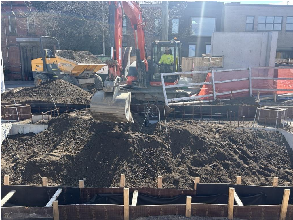
Photo 2: ECD backfilling previously imported clean fill in the western part of the site (facing west)
