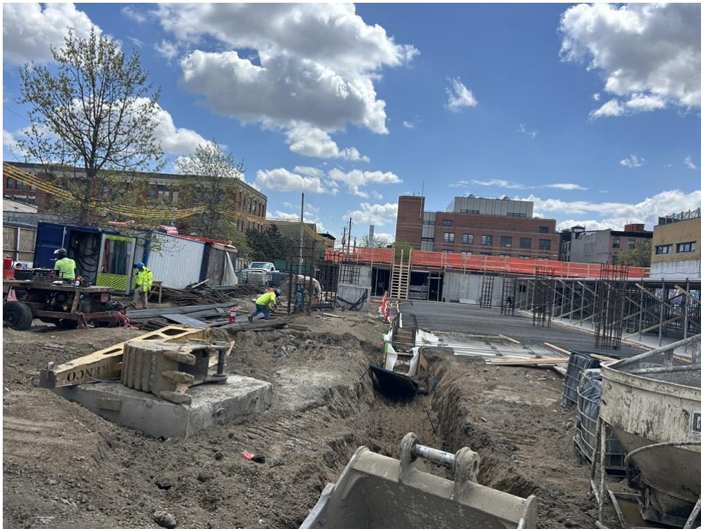
Photo 4: General view of the southern part of the site (facing south)
