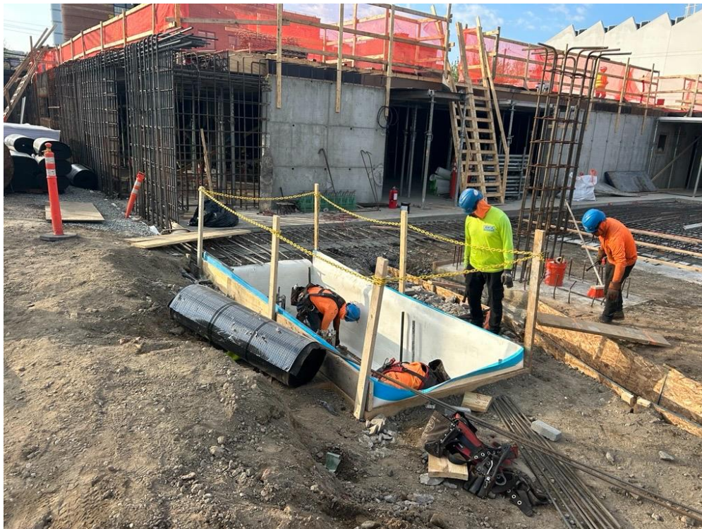
Photo 2: ECD installing Preprufe 300R Plus waterproofing/vapor barrier in the eastern part of the site (facing south)
