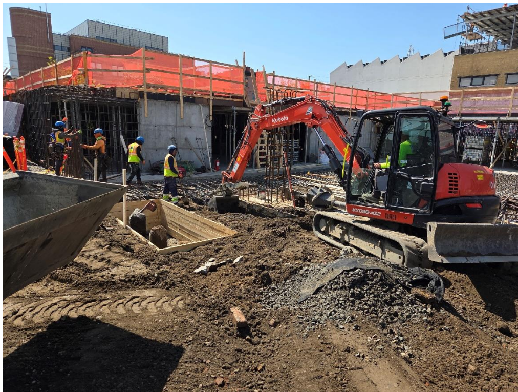
Photo 2: ECD excavating in the eastern part of the site (facing south)
