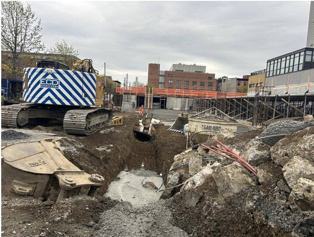
Photo 1: General view of the southern part of the site (facing south)
