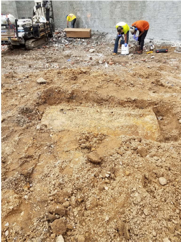
Photo 10, View of underground storage tank (UST) identified on-Site during site characterization sampling activities
