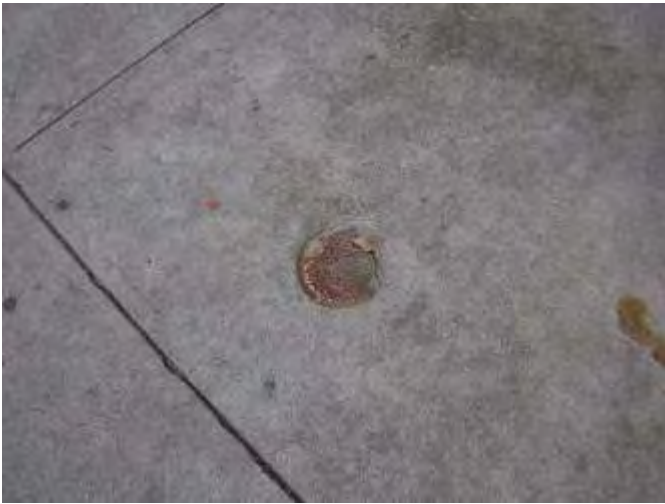
9. Abandoned monitoring well in sidewalk
