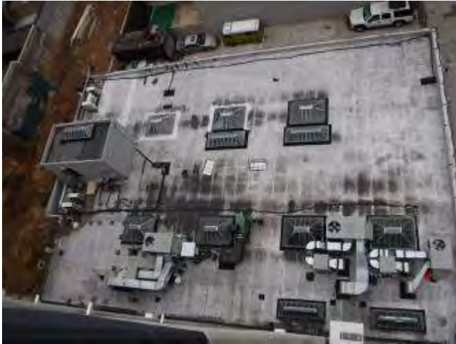
19. Roof of 98 South 4 th
