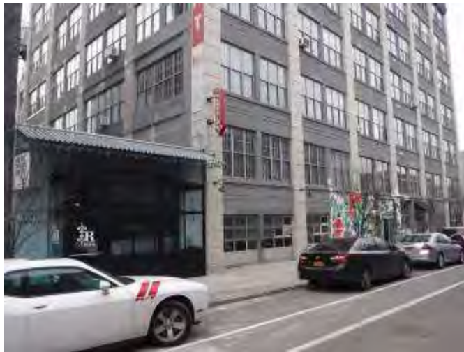
3. Front of 104 (and 100) South 4 th Street
