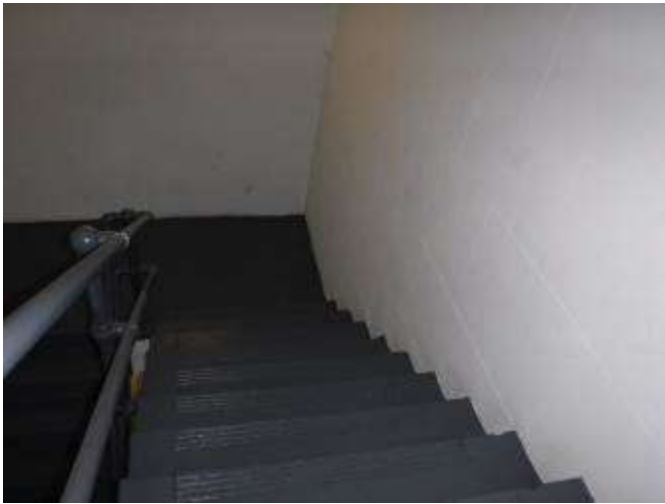
21. 100 South 4 th stairwell
