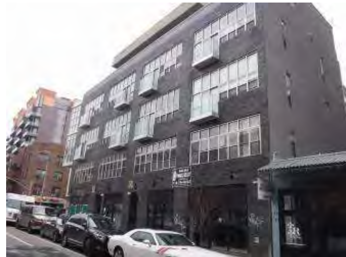
4. Abutting to east
