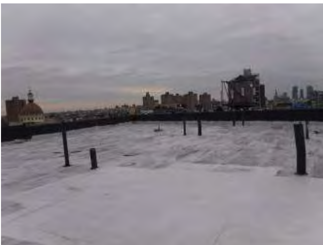
17. 100 South 4 th roof
