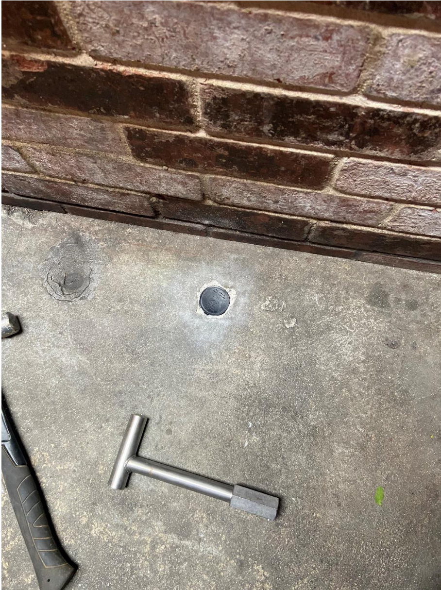
Photograph No. 3: View of typical conversion of temporary to permanent soil vapor point.
