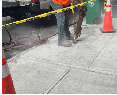
Photo showing dust from breaking concrete pre-hand clear.
