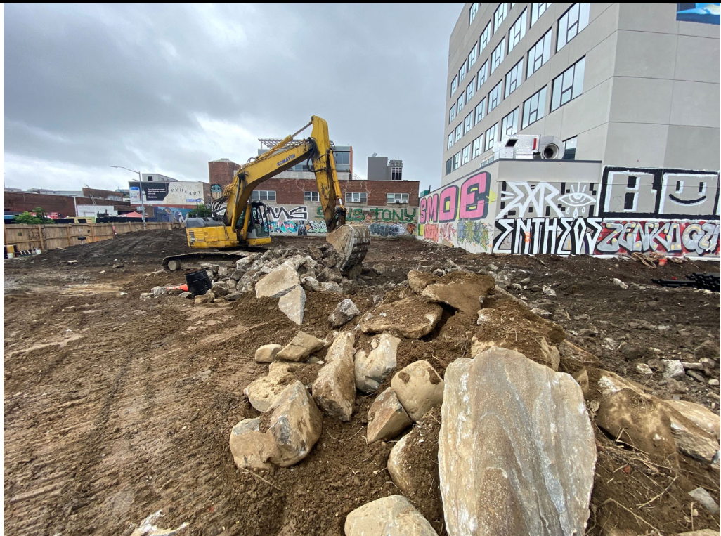
Photo 2: View of the Site and concrete debris awaiting offsite disposal.
