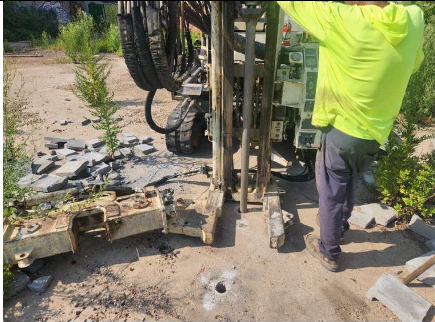
Photo 1: View of geoprobe boring operation.
