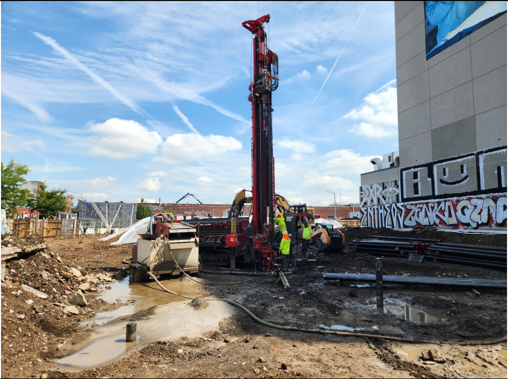
Photo 2: View of geothermal well installation.
