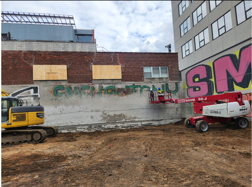
Photo 2: Removal of graffiti on a neighboring façade.
