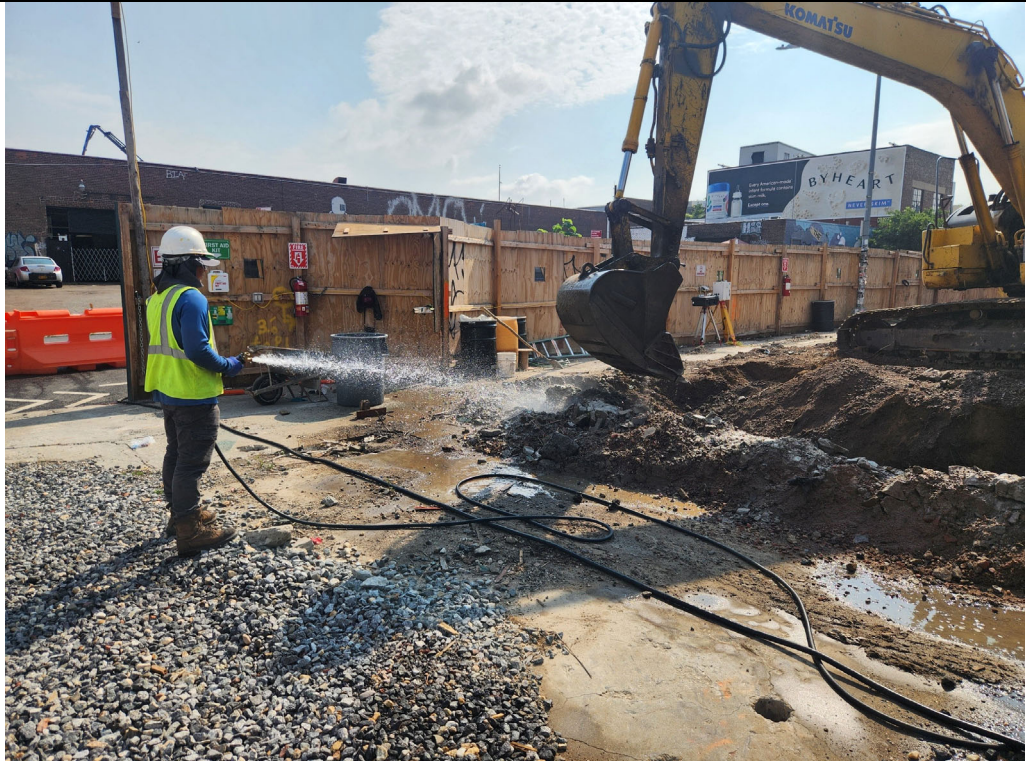
Photo 2: Utilizing water during excavation to minimize dust generation.
