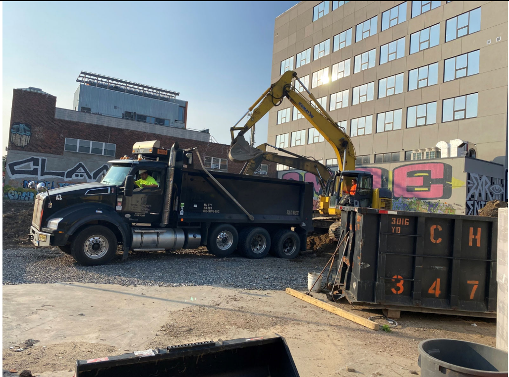
Photo 2: Concrete debris is being loaded into a truck for offsite disposal.
