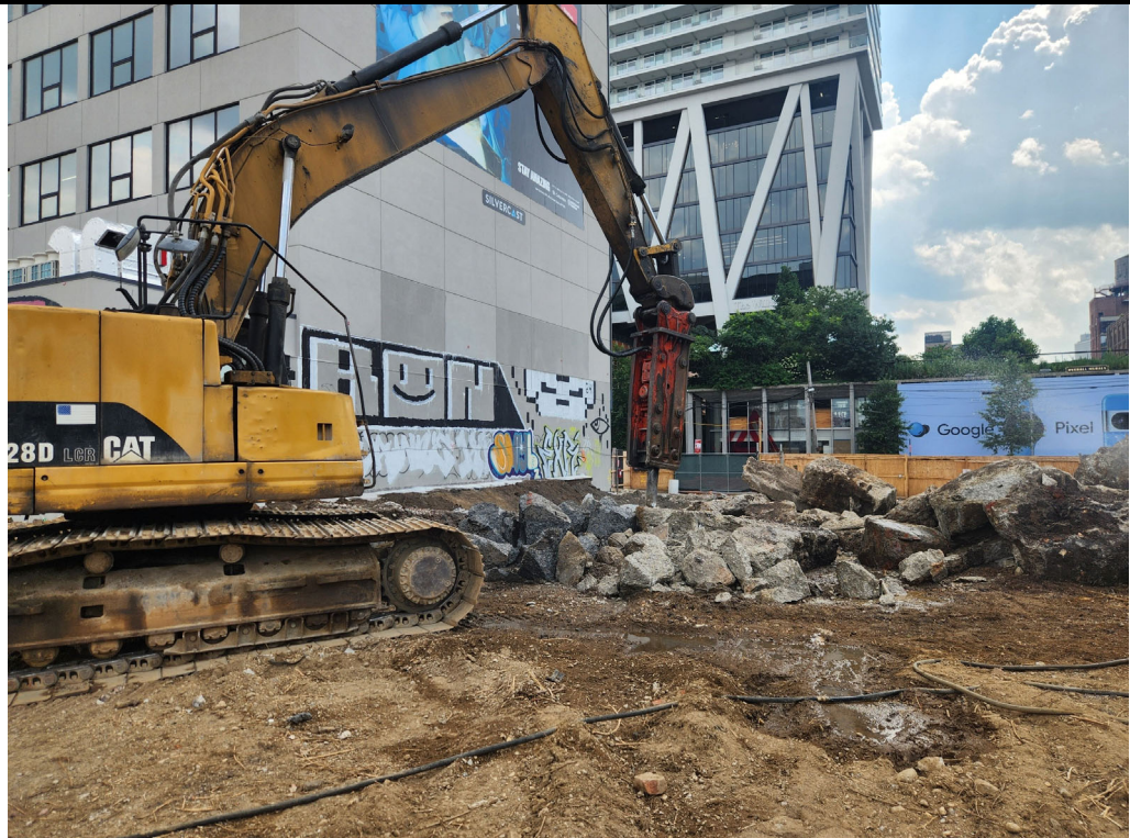
Photo 2: View of concrete demolition.
