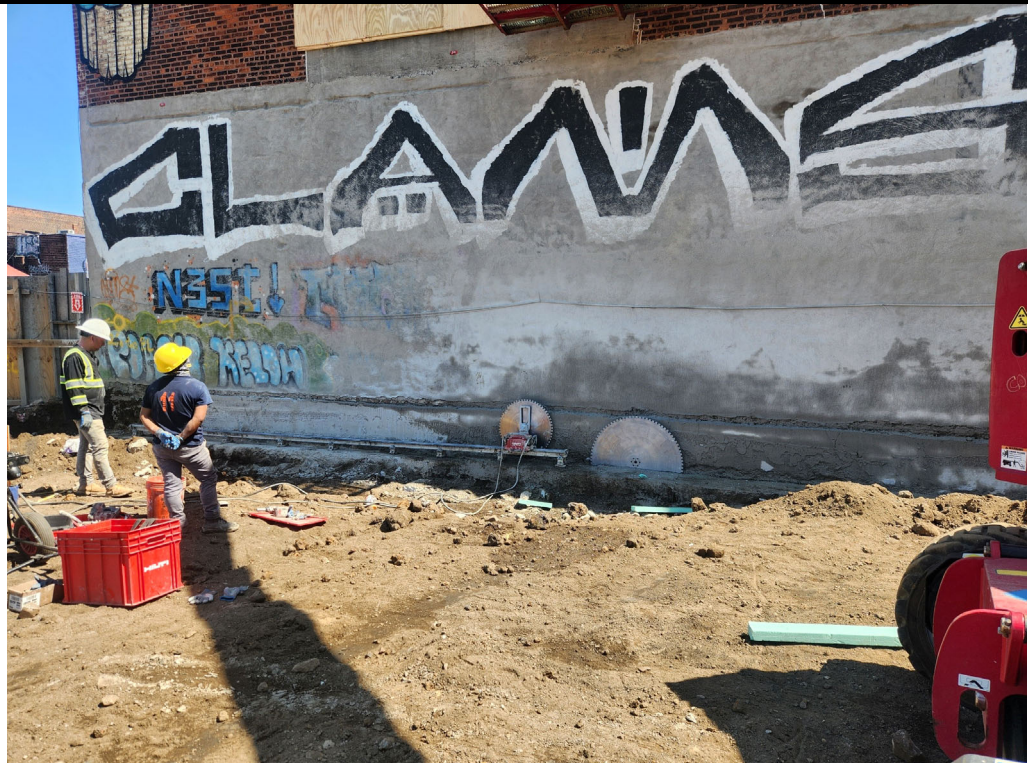
Photo 2: View of demolition of former building foundations.
