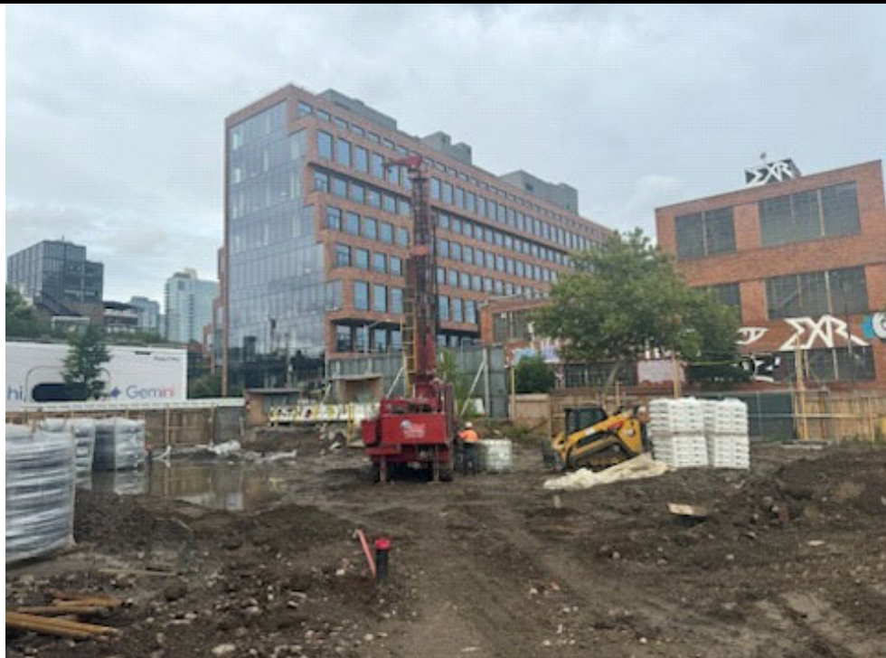
Photo 2: View of geothermal well installation.
