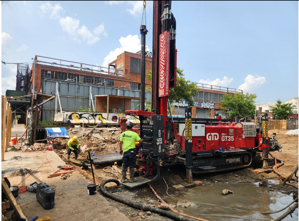
Photo 2: View of geothermal well installation.
