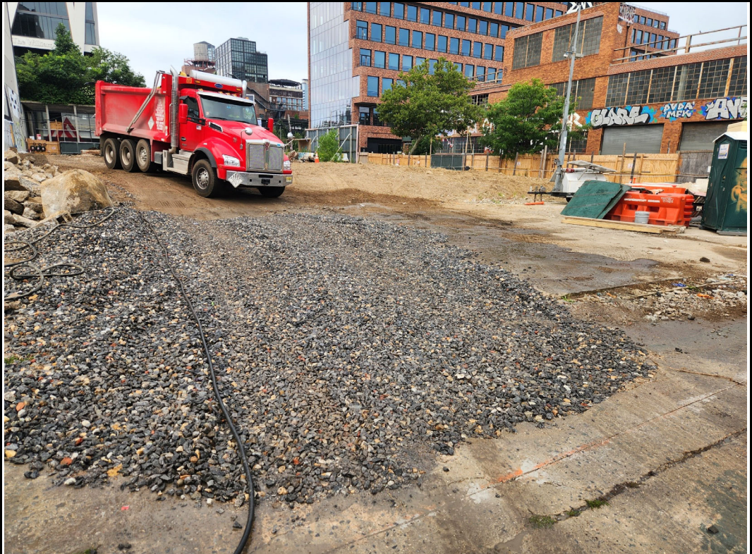
Photo 2: View of the truck wash pad.
