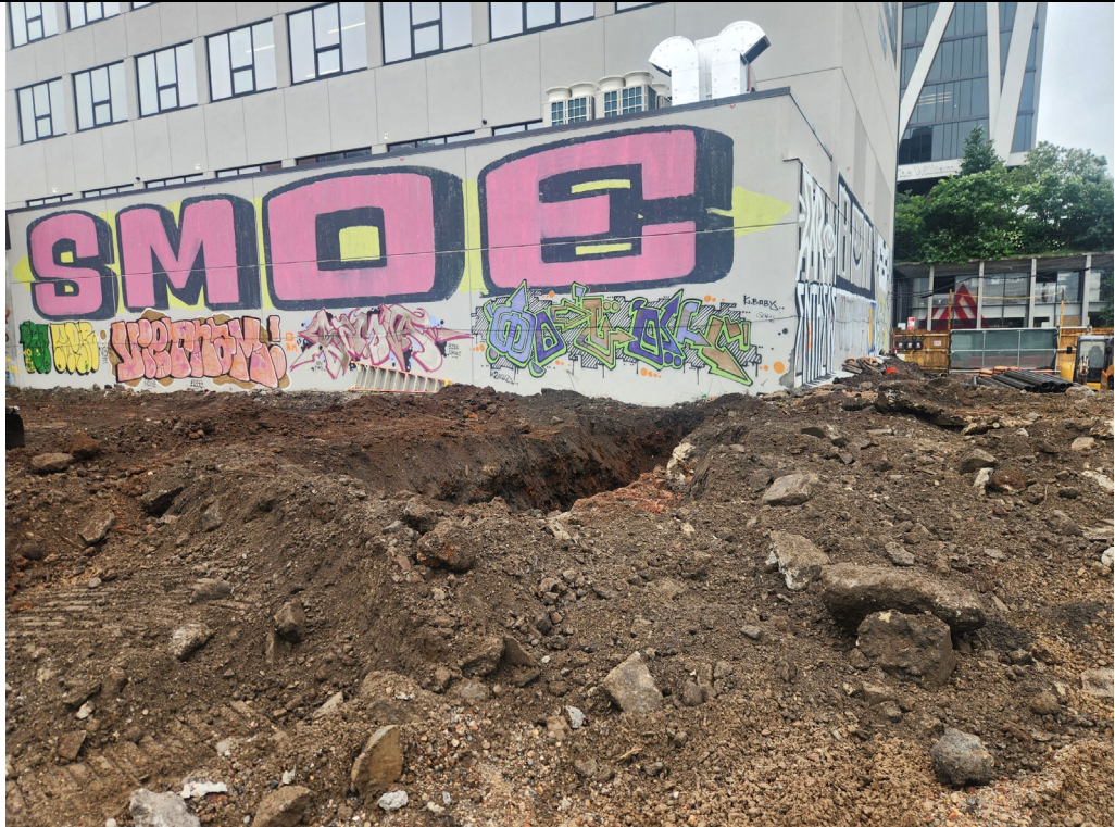
Photo 2: View of excavation.
