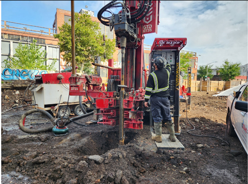
Photo 2: View of geothermal well installation.
