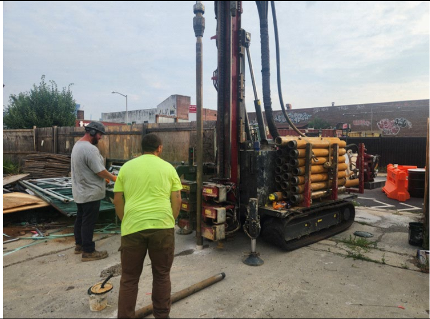
Photo 1: View of drilling operation.
