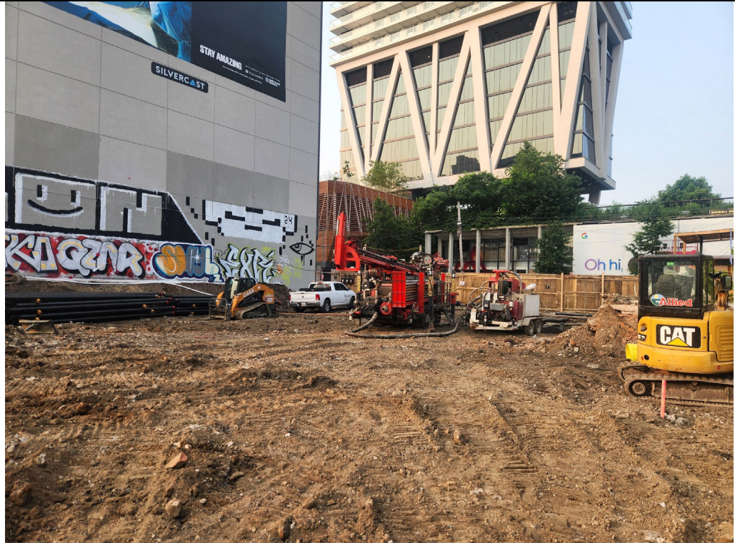
Photo 2: View of geothermal well installation.
