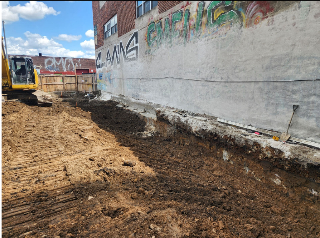
Photo 2: View of former building foundational elements exposed for demolition.
