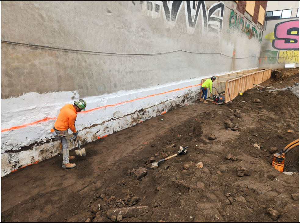
Photo 2: Preparing for SOE installation.
