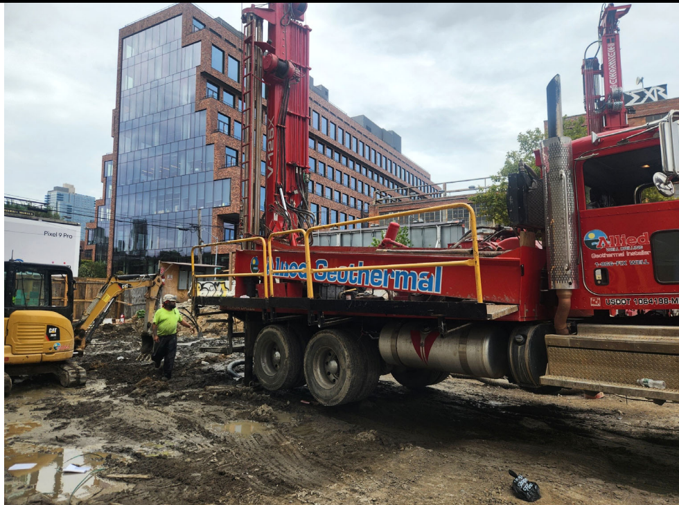
Photo 2: View of geothermal well installation.
