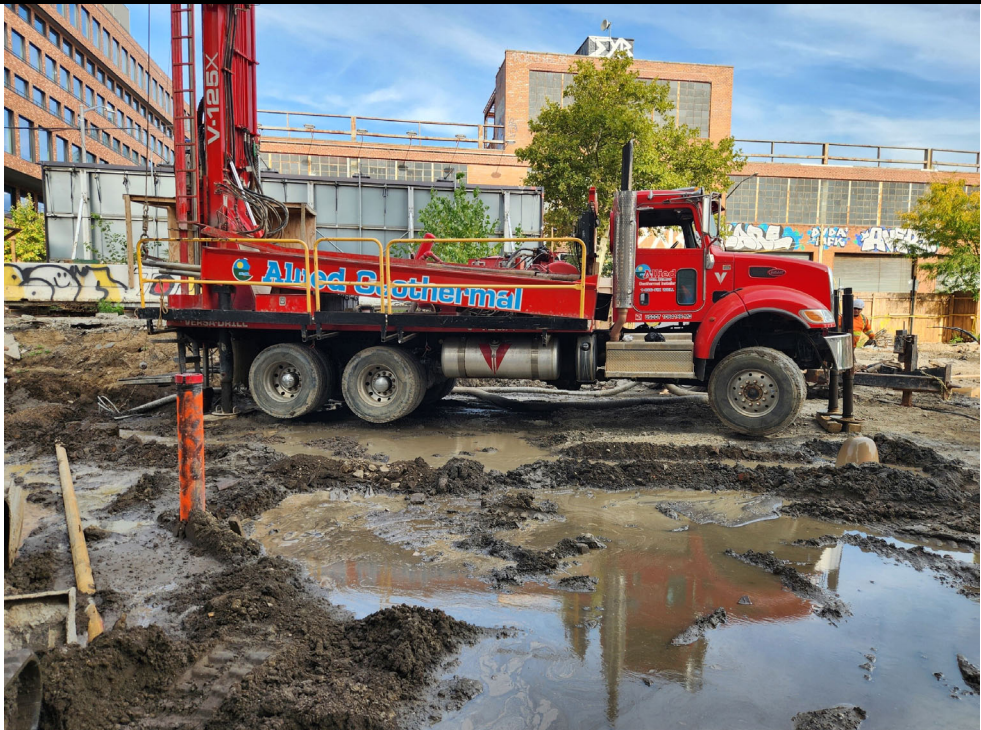
Photo 2: View of geothermal well installation.
