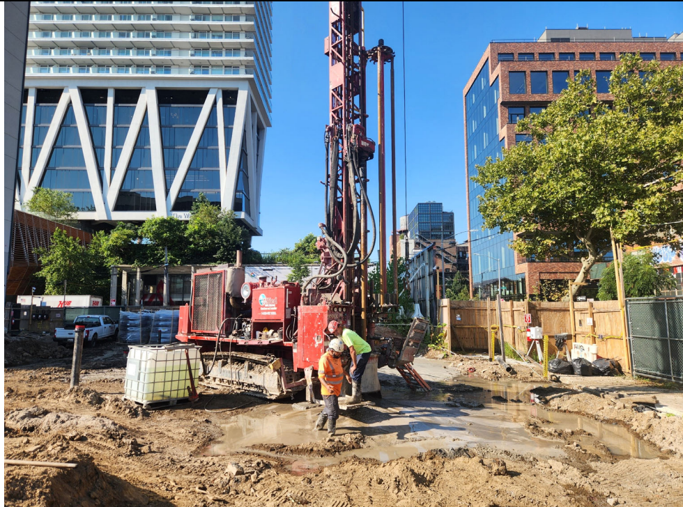
Photo 2: View of geothermal well installation.
