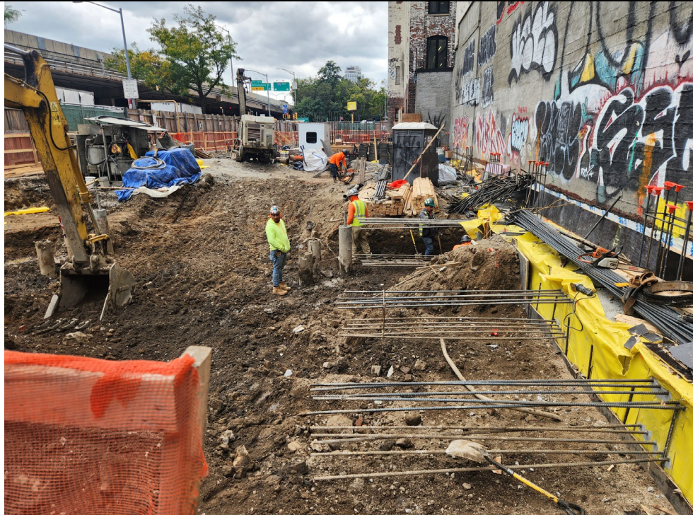
Photo 2: View of soil excavation.
