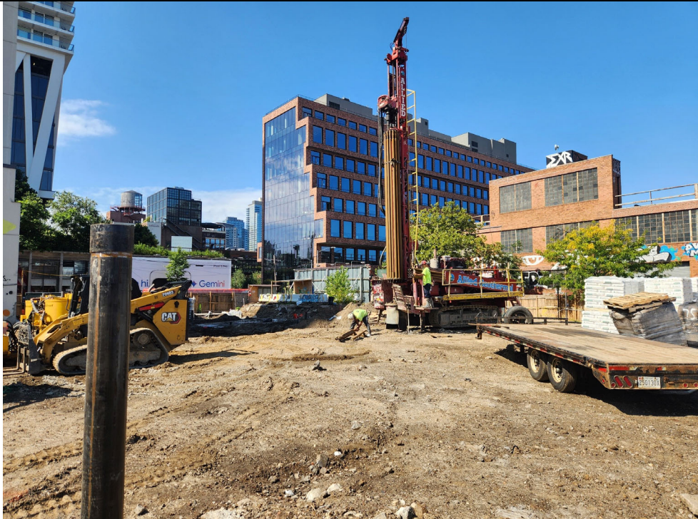
Photo 2: View of geothermal well installation.
