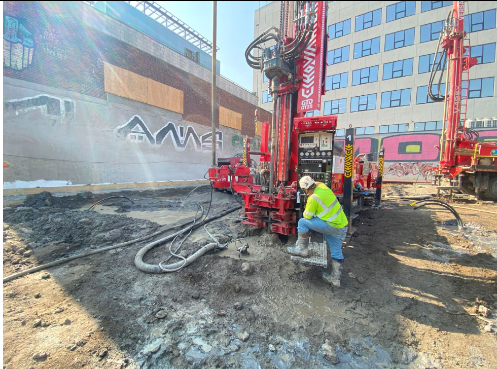
Photo 2: View of geothermal well installation.
