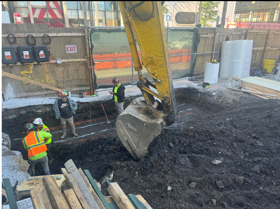
Photo 2: Minor excavation in preparation for SOE installation.
