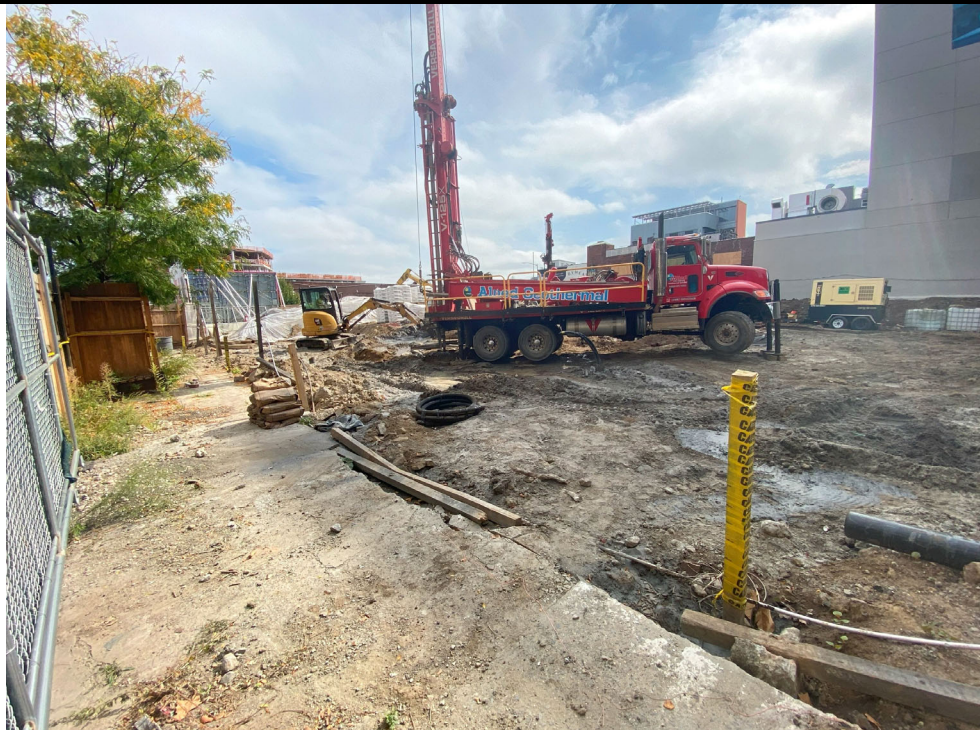
Photo 2: View of geothermal well installation.
