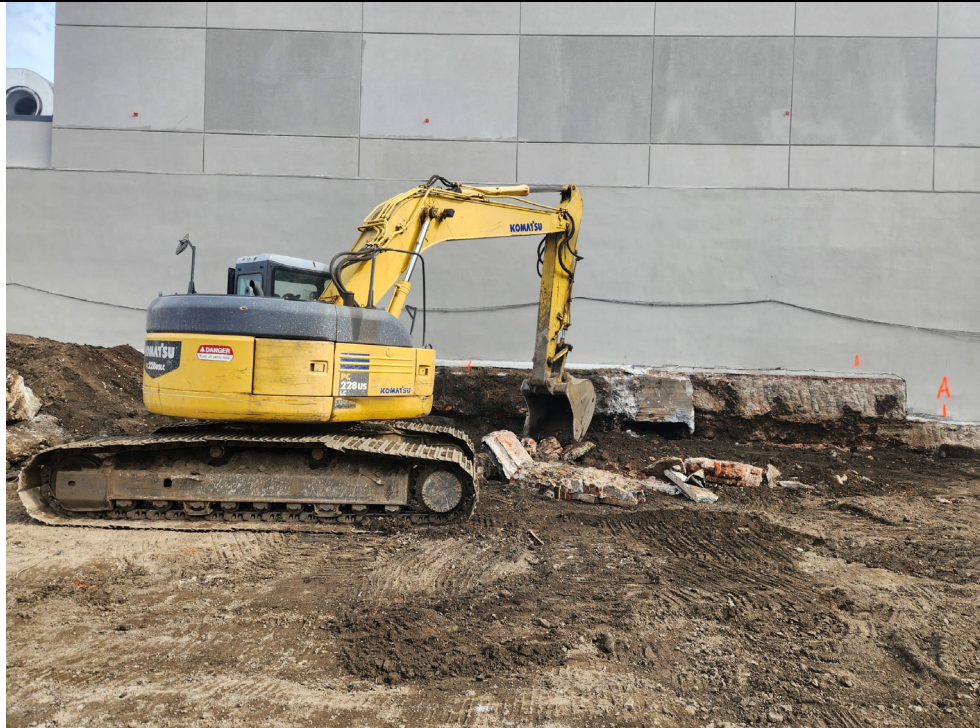
Photo 2: View of excavation in preparation to install SOE elements.
