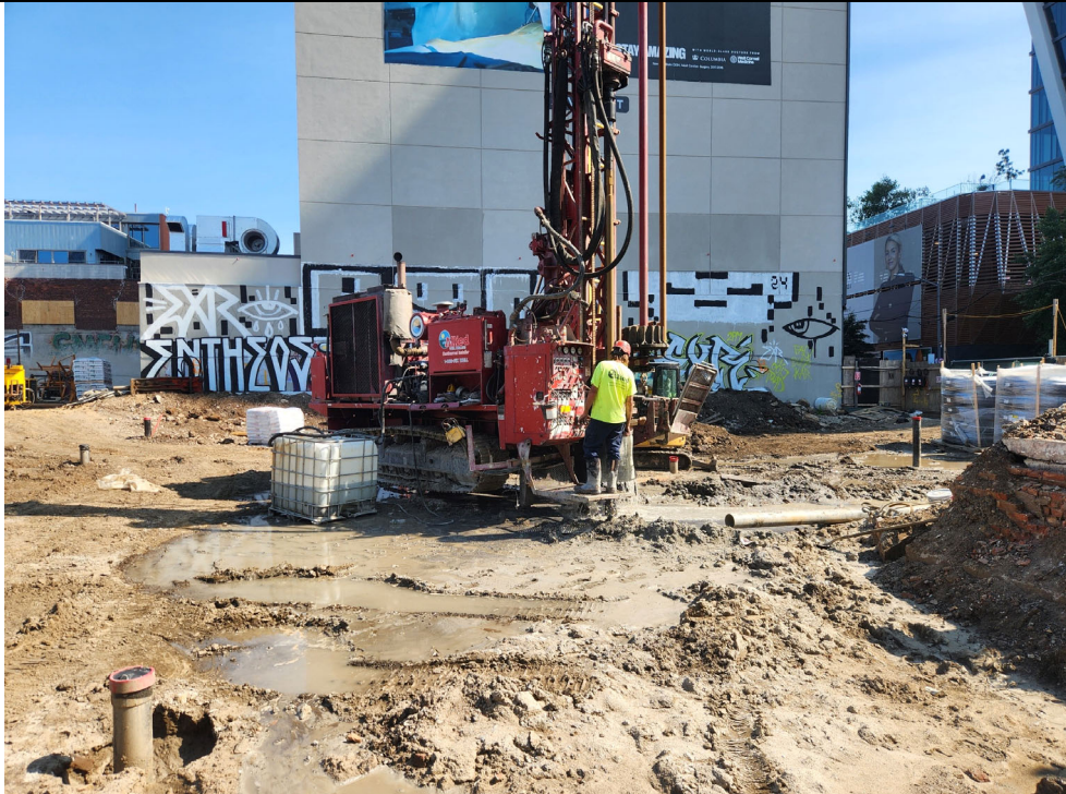
Photo 2: View of geothermal well installation.
