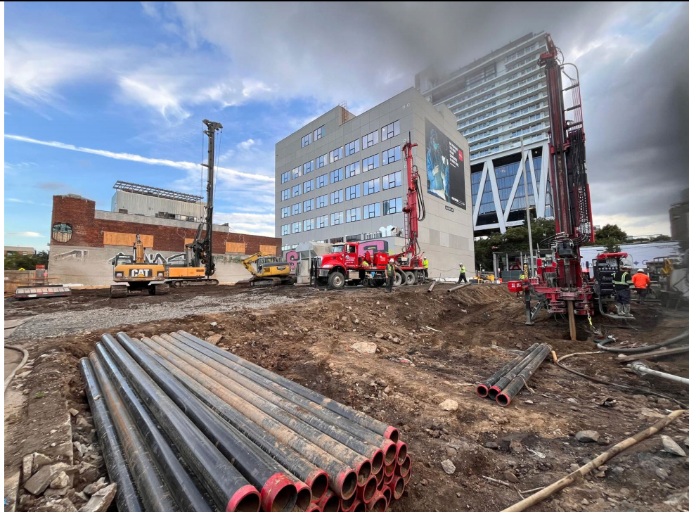
Photo 2: View of geothermal well installation.
