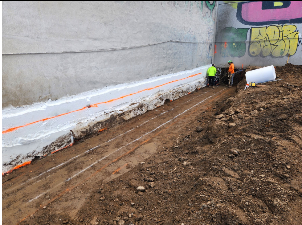
Photo 2: Preparing for SOE installation.
