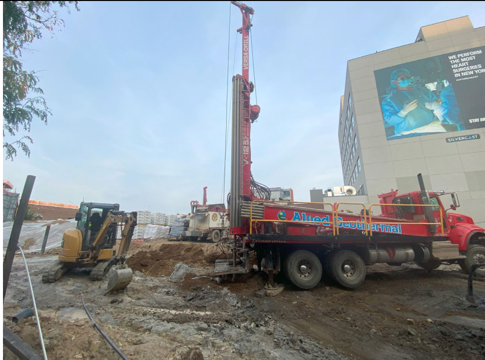
Photo 2: View of geothermal well installation.
