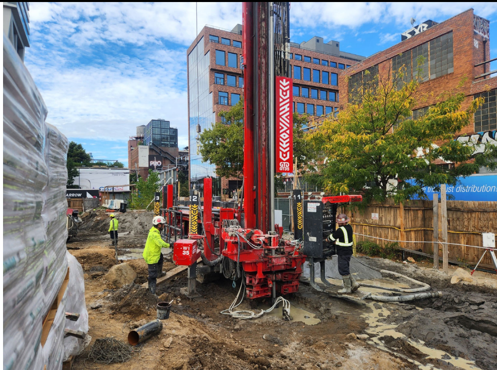
Photo 2: View of geothermal well installation.
