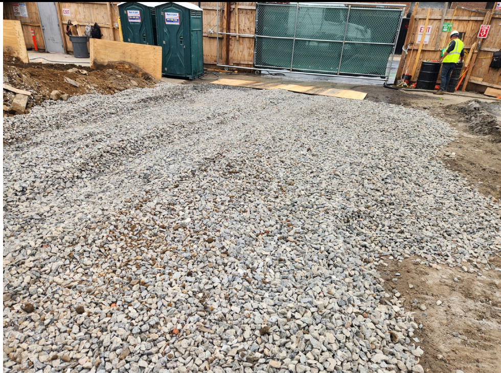
Photo 2: View of the truck wash pad.
