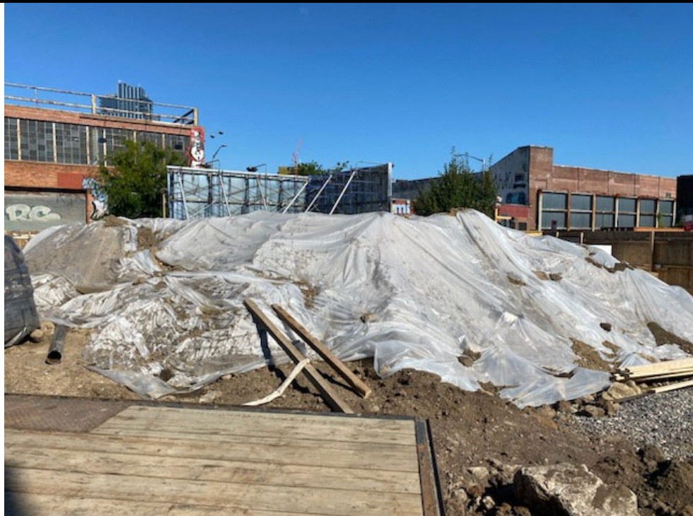
Photo 2: View of a covered non-hazardous soil stockpile.
