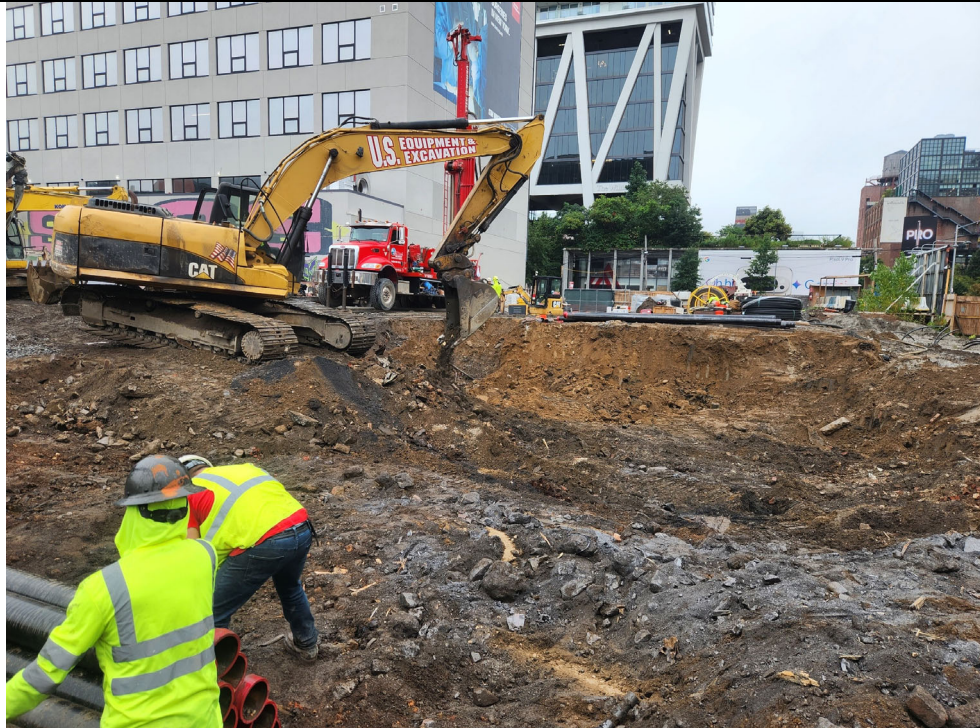
Photo 2: View of excavation.
