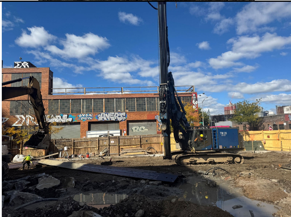
Photo 2: View of sheet pile installation.
