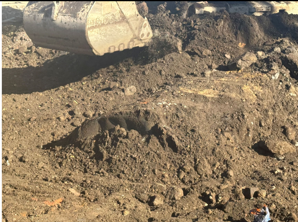
Photo 2: View of the second UST discovered during excavation.
