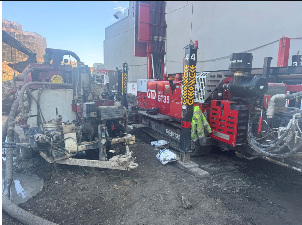
Photo 2: View of geothermal well installation.
