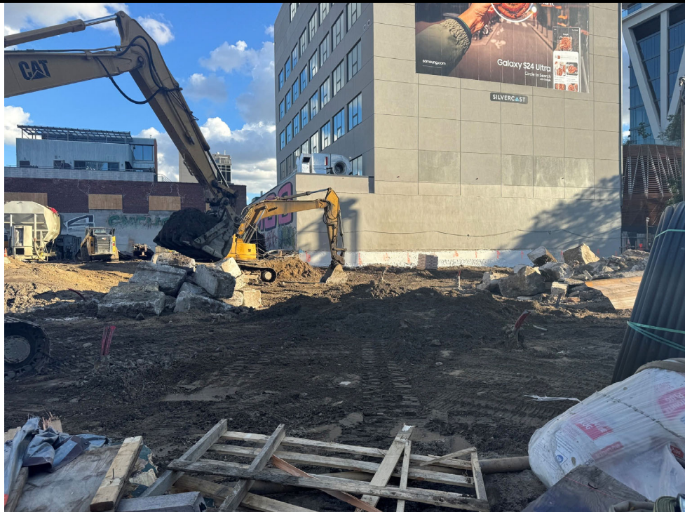
Photo 2: View of excavation.
