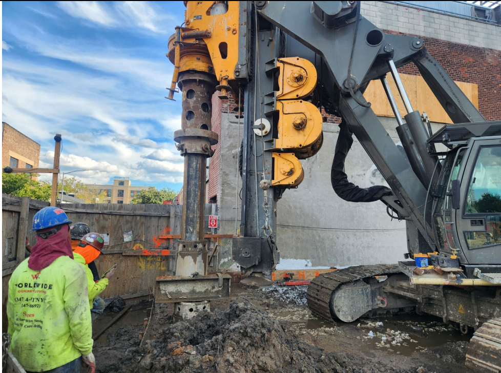
Photo 2: View secant pile installation.
