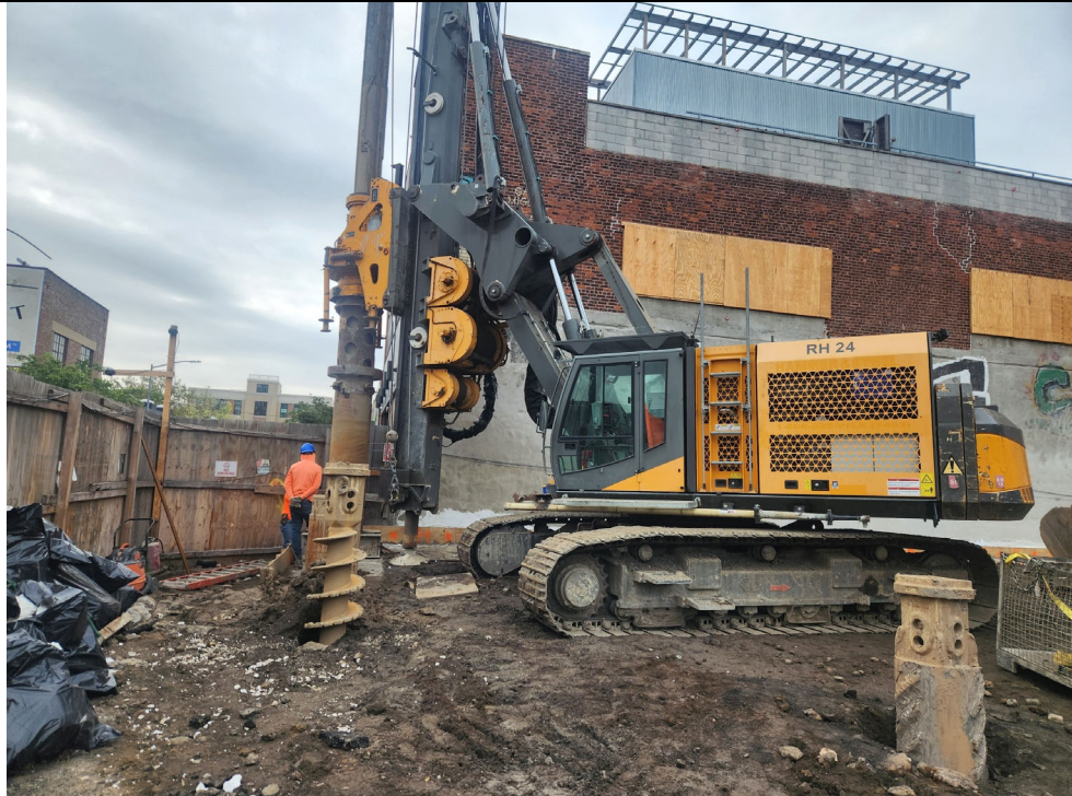
Photo 2: View of secant pile installation.
