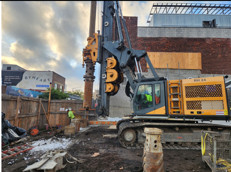
Photo 2: View of secant pile installation.
