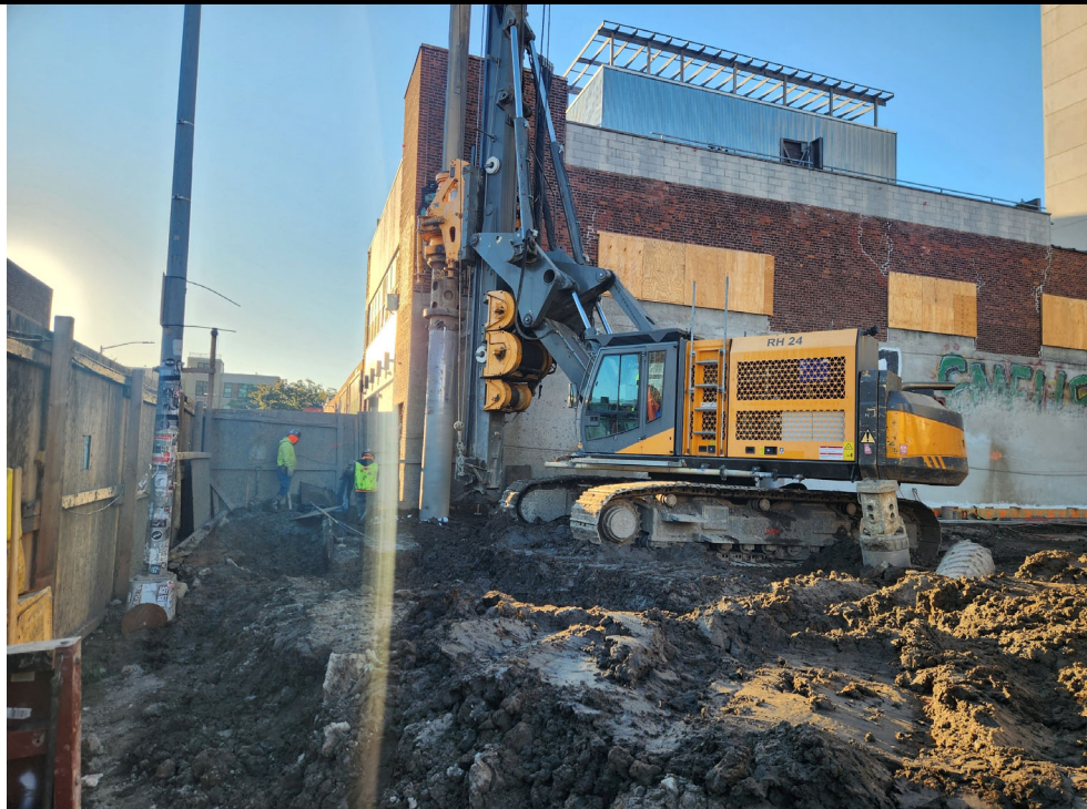
Photo 2: View of secant pile installation.
