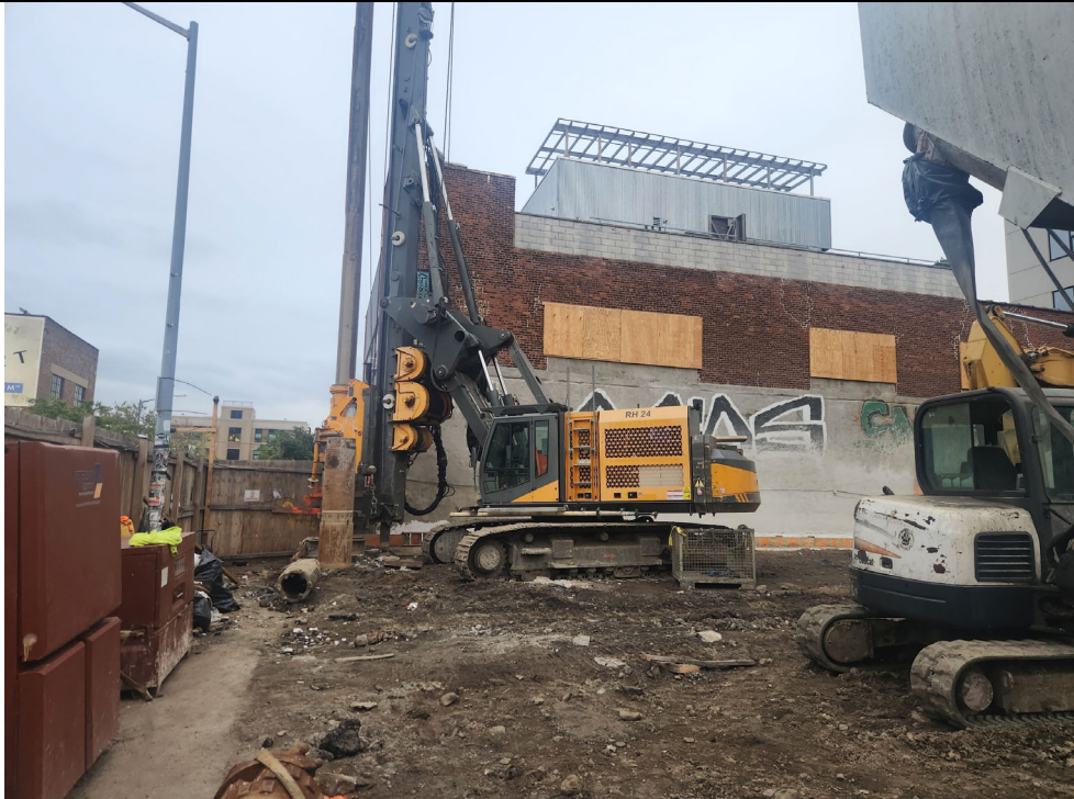
Photo 2: View secant pile installation.
