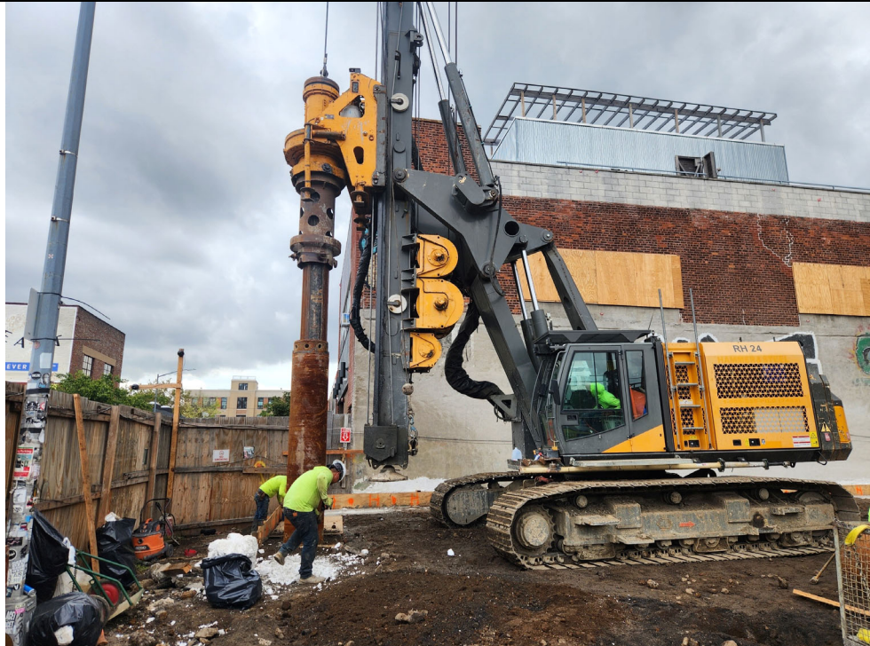
Photo 2: View of secant pile installation.
