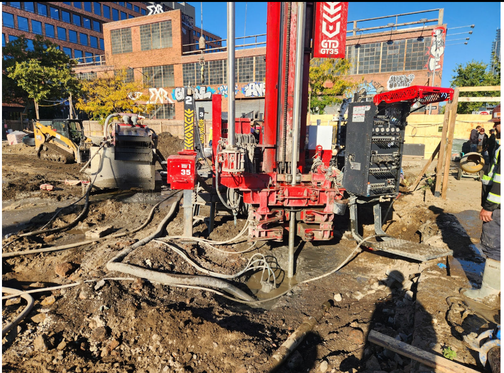
Photo 2: View of geothermal well installation.
