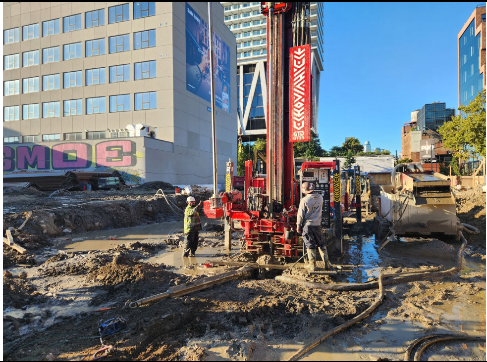
Photo 2: View of geothermal well installation.
