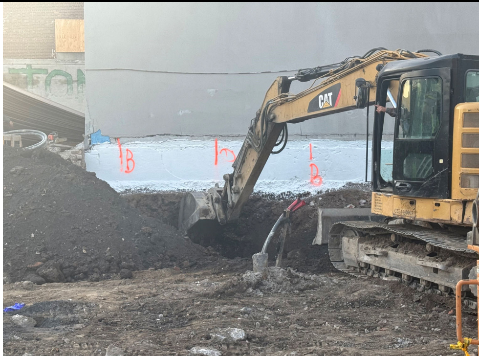
Photo 2: View of non-hazardous soil excavation.
