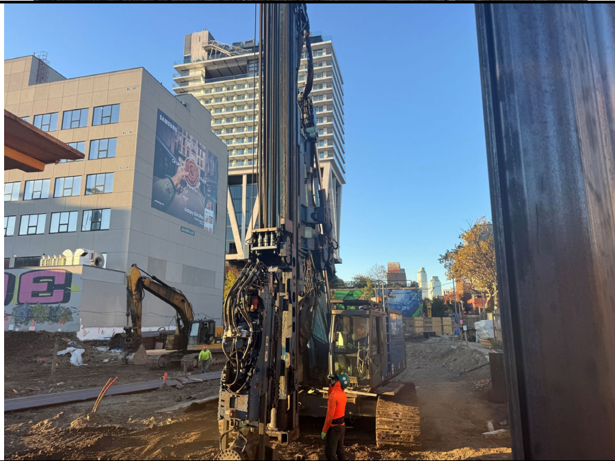
Photo 2: View of sheet pile installation.
