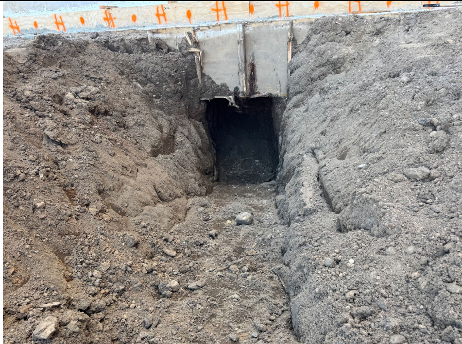
Photo 2: View of excavation.
