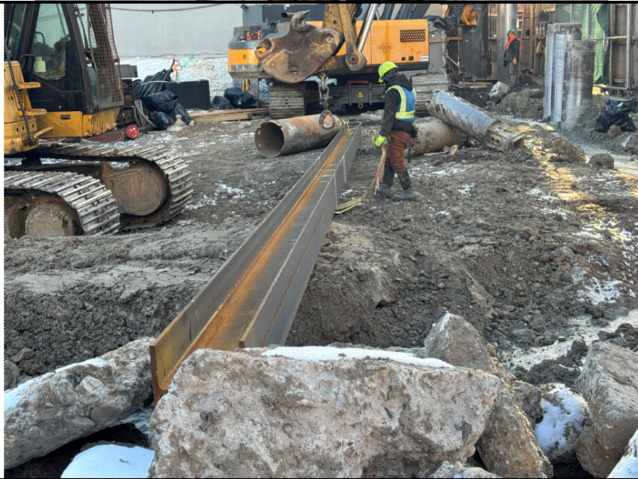
Photo 2: View of secant pile installation and material mobilization.
