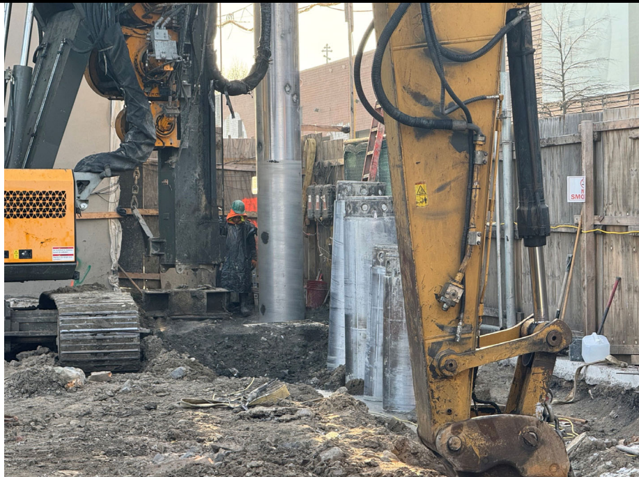
Photo 2: View of secant pile installation.
