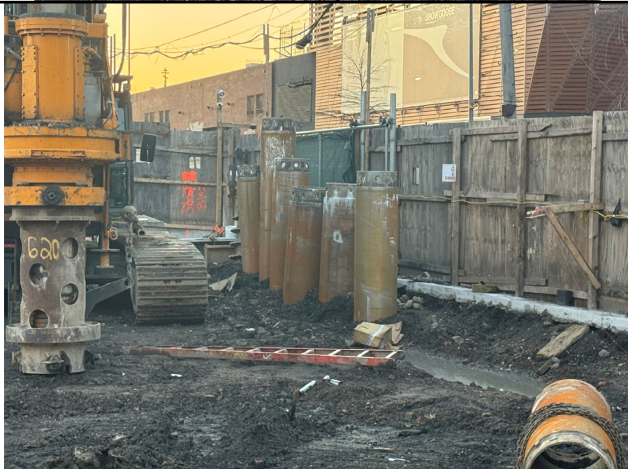
Photo 2: View of secant pile installation.
