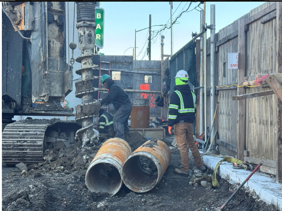
Photo 2: View of secant pile installation.
