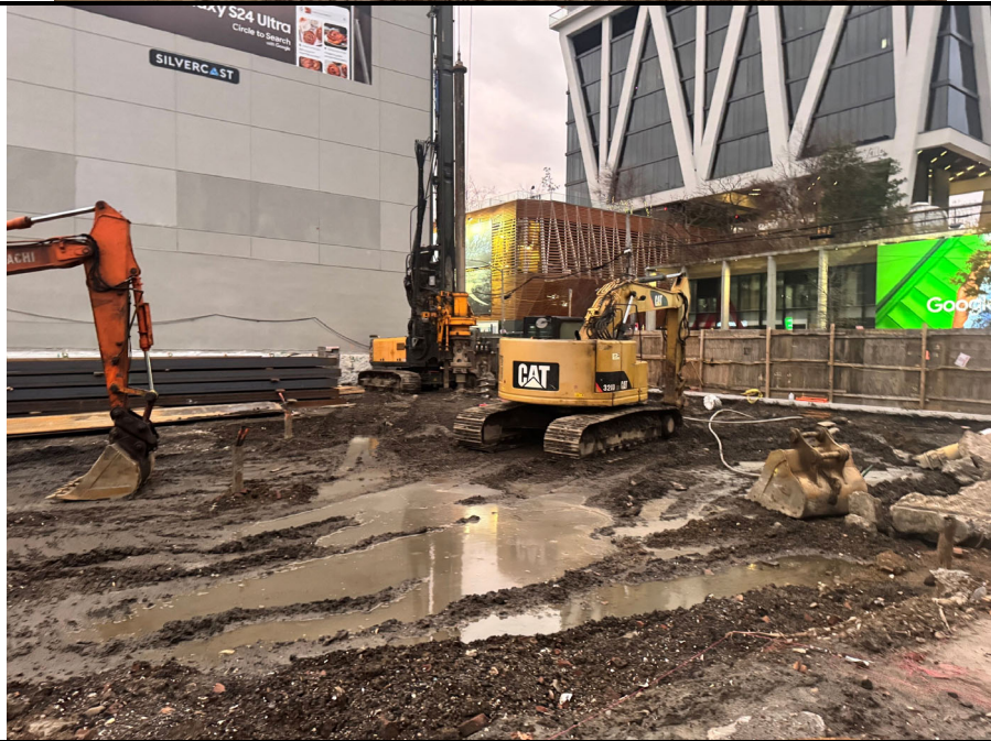
Photo 2: View of secant pile installation.
