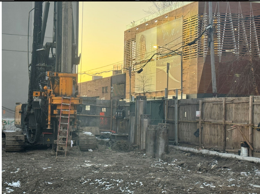
Photo 2: View of secant pile installation.
