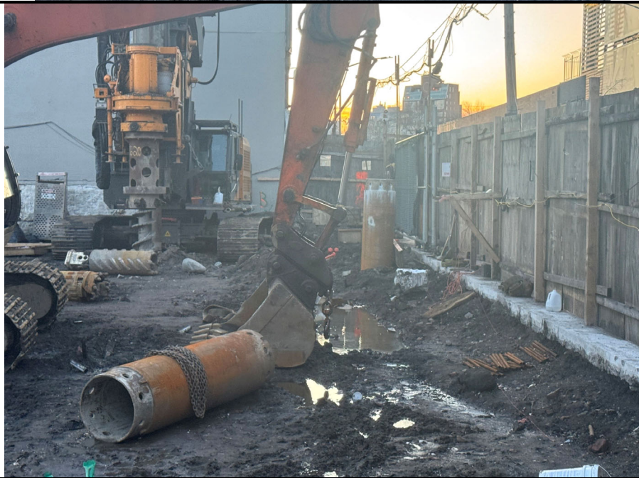
Photo 2: View of secant pile installation.
