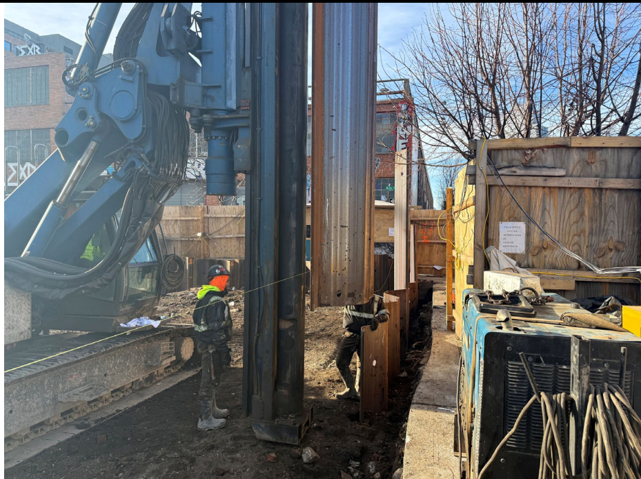
Photo 2: View of sheet pile installation.
