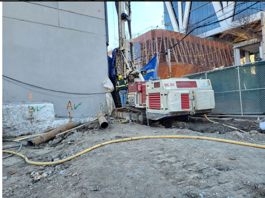
Photo 2: View of secant pile installation.
