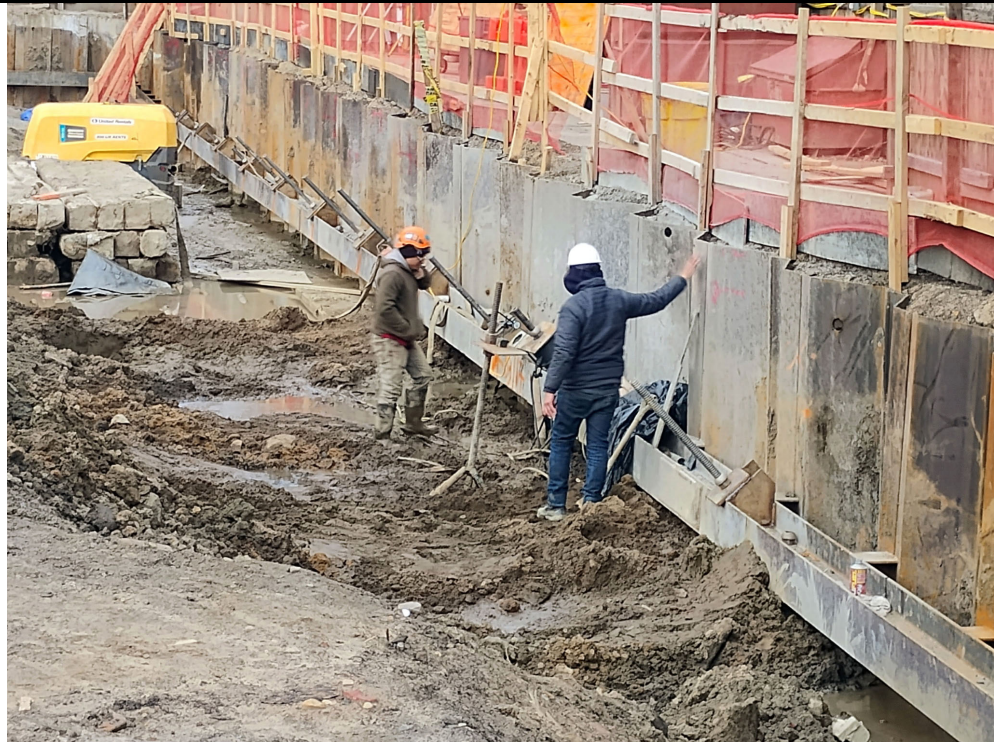
Photo 2: View of tie back testing.
