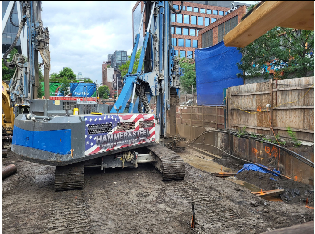
Photo 2: View of caisson installation.
