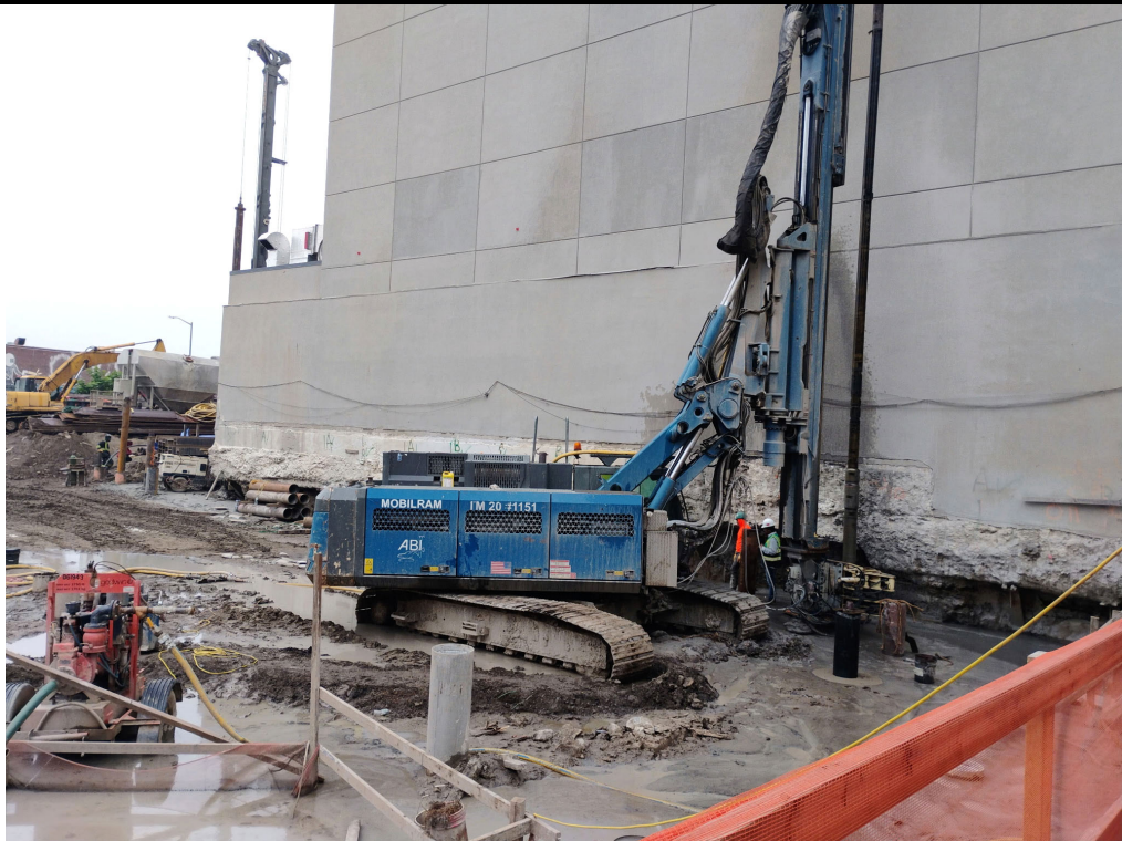
Photo 2: View of caisson installation.
