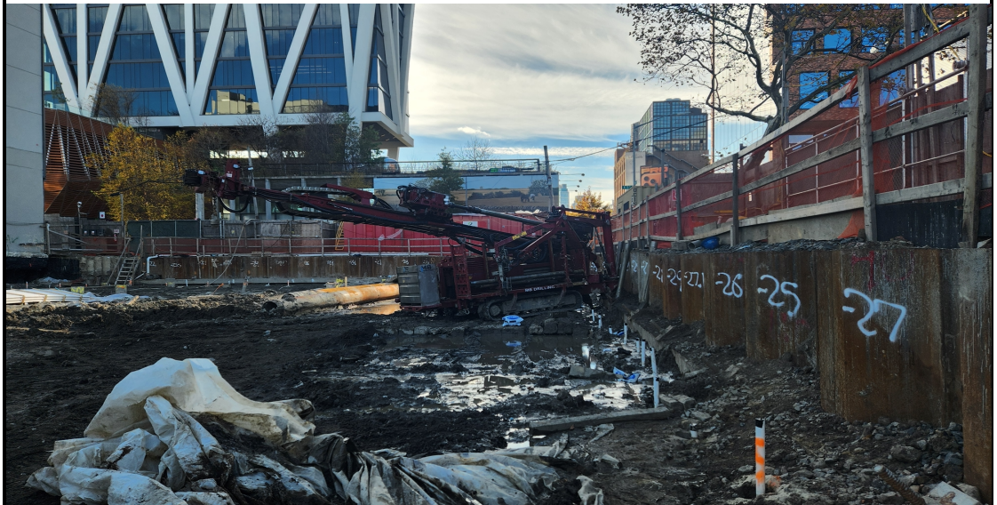
Photo 2: View of dewatering well installation.
