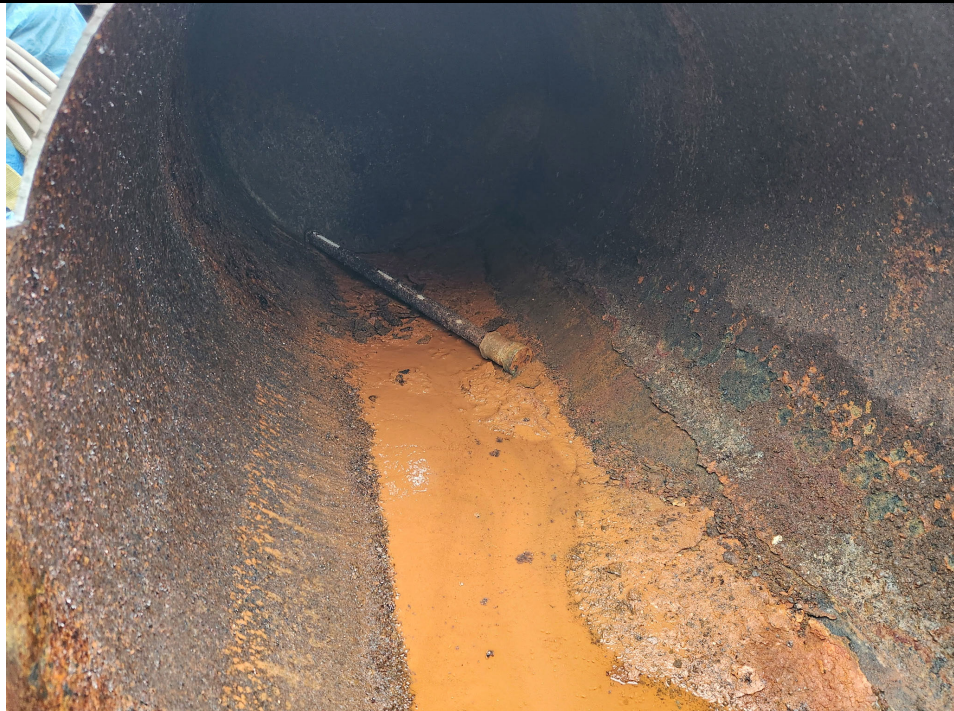
Photo 2: View of the interior of UST-5 prior to cleaning.
