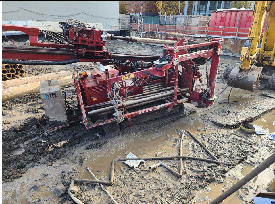
Photo 2: View of drill rig mobilization.
