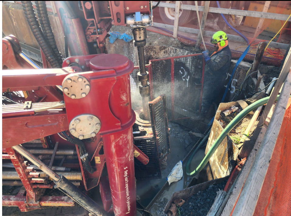
Photo 2: View of dewatering well installation.
