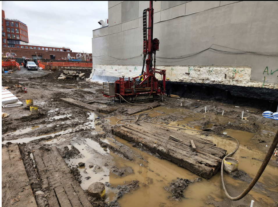
Photo 2: View of dewatering well installation.
