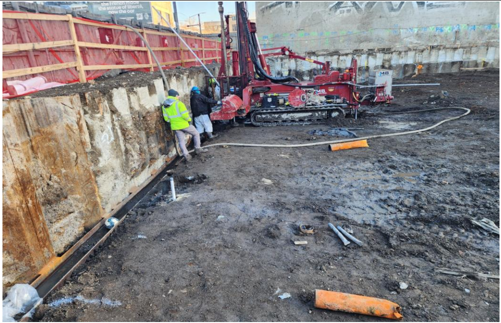
Photo 1: View of dewatering well installation
