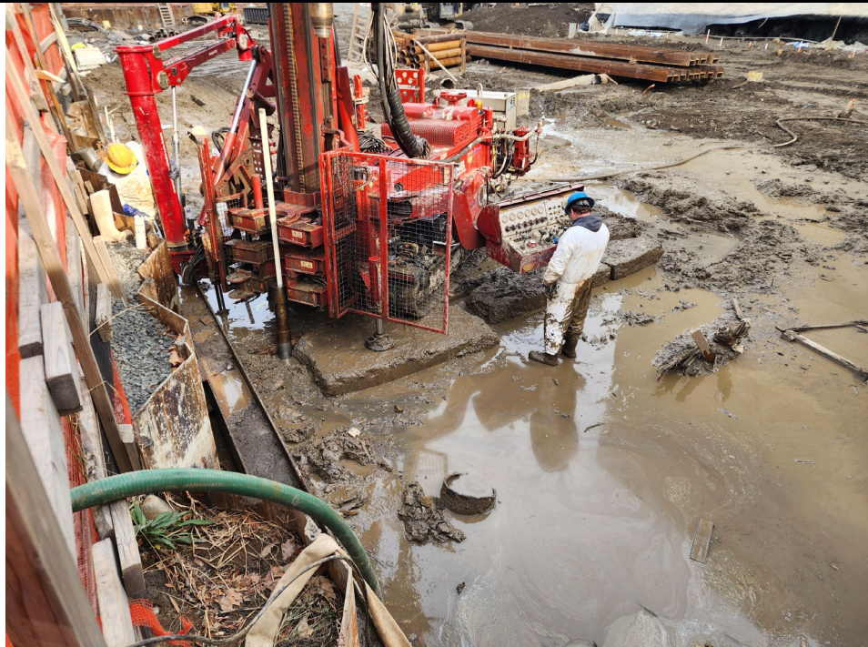
Photo 2: View of dewatering well installation.
