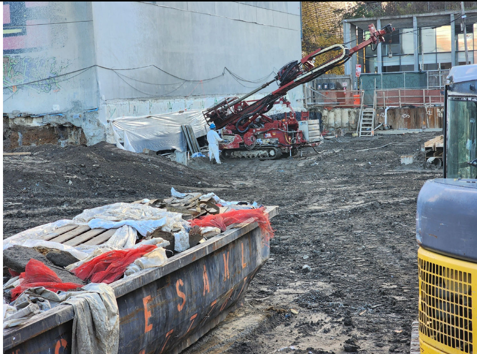
Photo 2: View of dewatering well installation.
