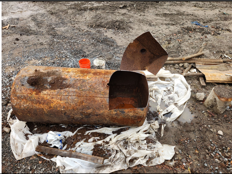
Photo 1: View of UST-5 following cutting.
