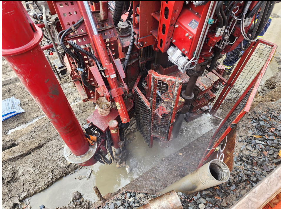
Photo 2: View of dewatering well installation.
