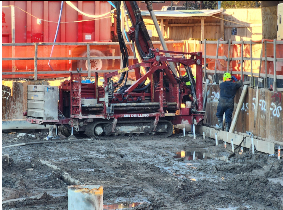
Photo 2: View of dewatering well installation.
