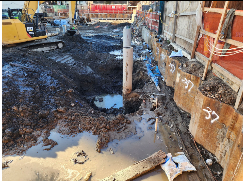
Photo 2: View of dewatering well installation.
