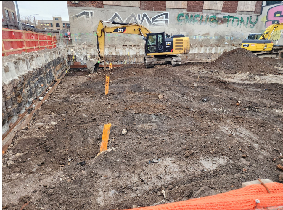
Photo 2: View of grading to accommodate drill rig for dewatering well installation.
