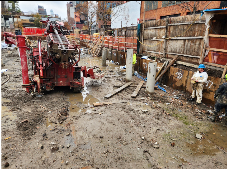
Photo 2: View of dewatering well installation.
