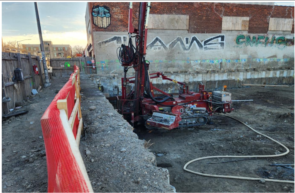
Photo 1: View of staged drill rig.
