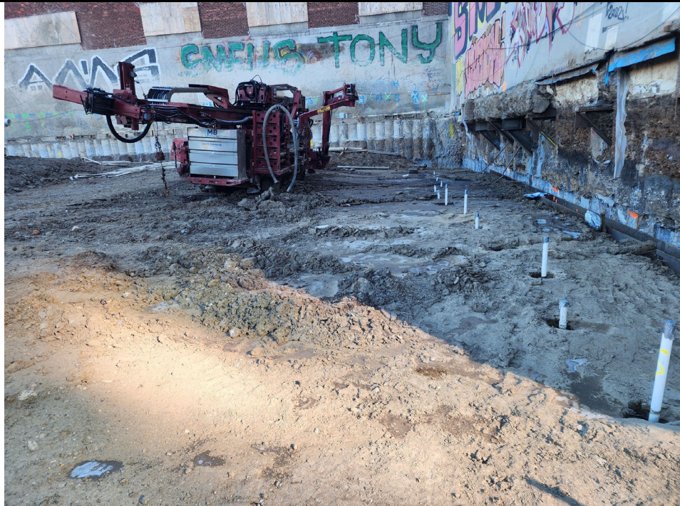
Photo 2: View of dewatering well installation.
