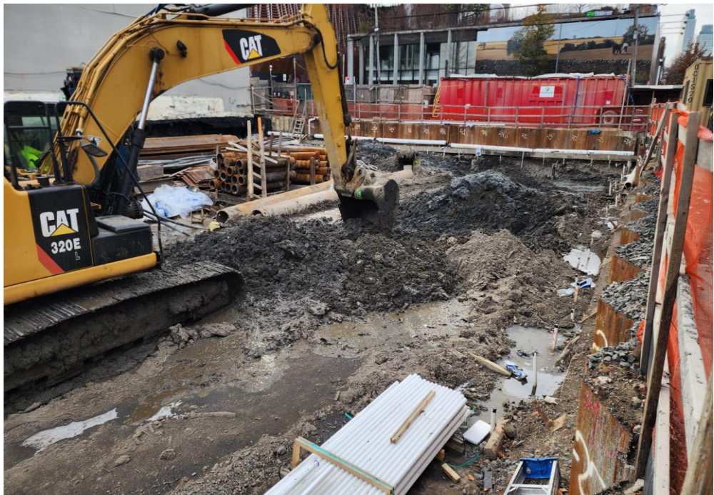
Photo 2: View of soil grading.
