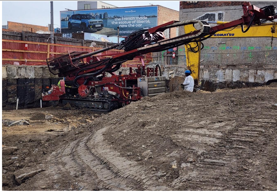
Photo 1: View of dewatering well installation.
