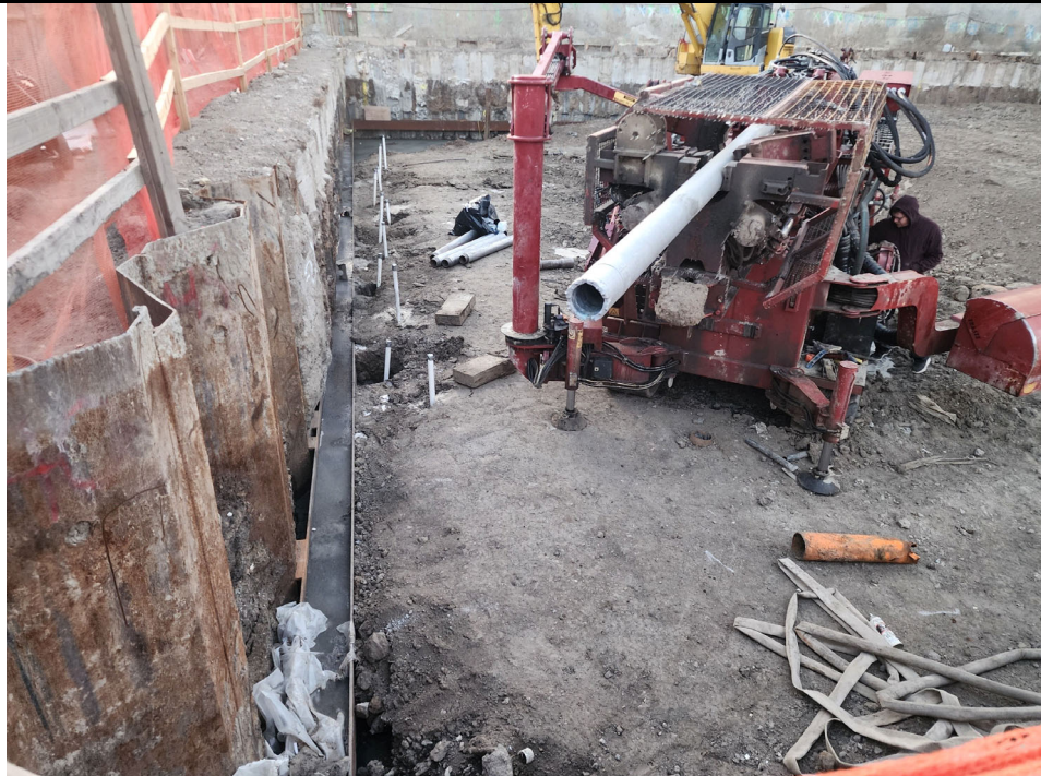
Photo 2: View of dewatering well installation.
