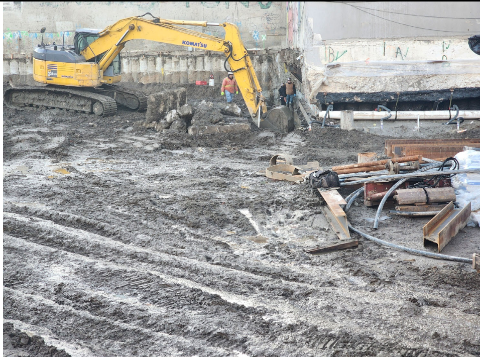
Photo 2: View of grading and stockpiled soil in preparation for offsite disposal.
