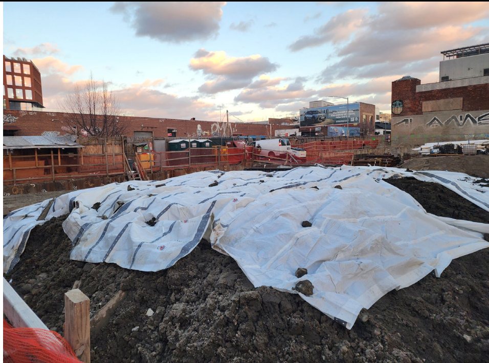
Photo 2: View of a soil stockpile covered with poly in preparation for offsite disposal.
