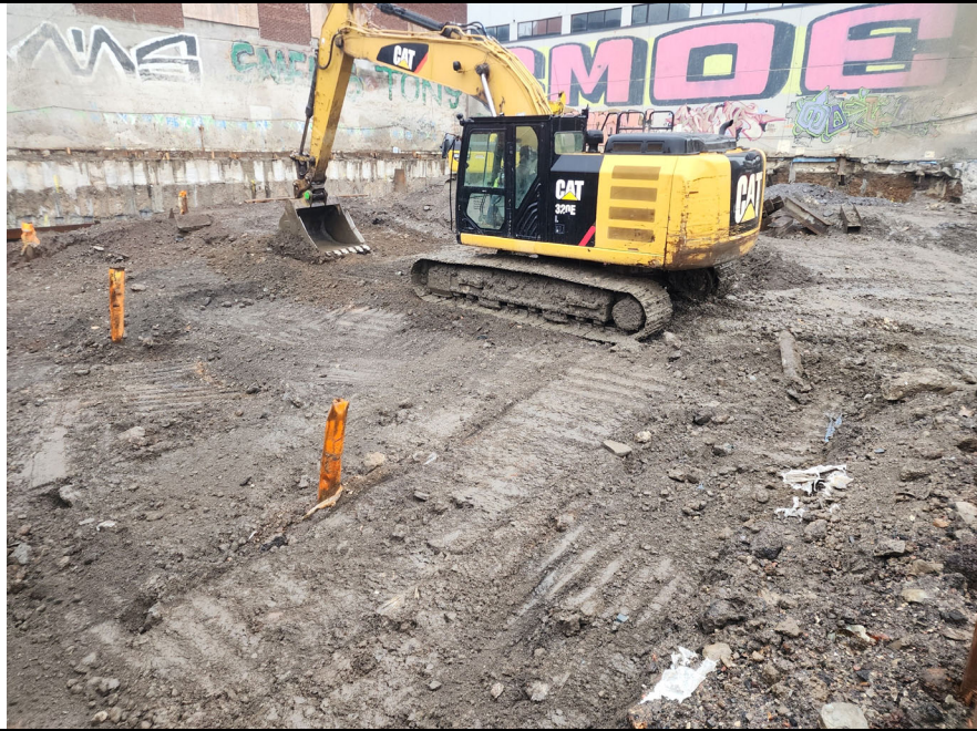
Photo 1: View of grading to accommodate drill rig for dewatering well installation.
